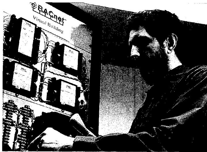
Mr. Steven Bushby, electronics engineer, checks wiring connections for controllers in the BACnet™ Virtual Building.
