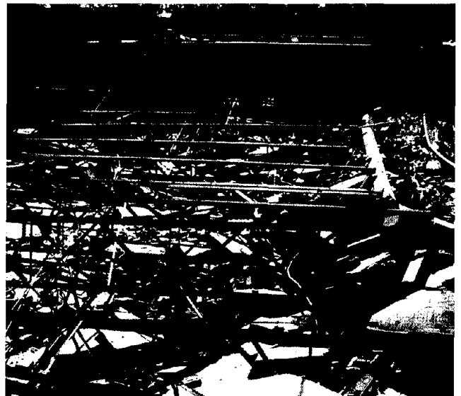
Collapsed, Oakgrove Elementary and High School Building constructed of lightly reinforced masonry block and brick veneer walls with RC bond beams that connected the steel roof truss to walls, Jefferson County, Alabama.
