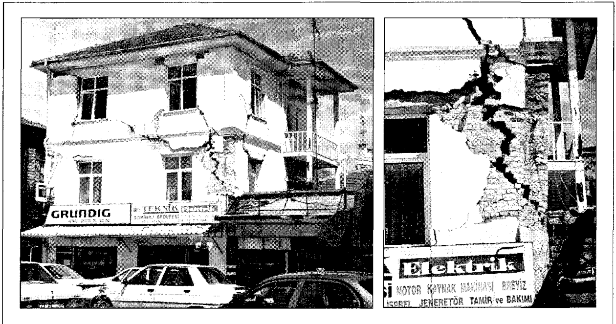
Figure 4-25 Damage to an unreinforced masonry building
