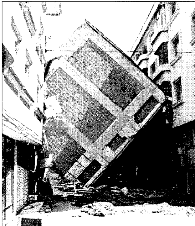
Figure 4-8 Failure of soft first story
