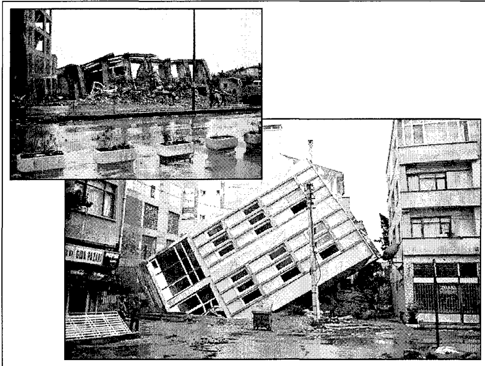
Figure 3-4 Buildings in Adapazarı that either toppled or partially overturned because soil beneath them liquefied and weakened the foundation
