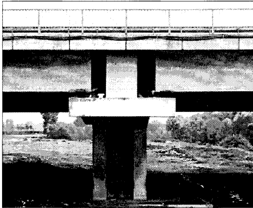
Figure 5-5 A side elevation of one of the pier of the northbound E-80 Motorway bridge over the Sakarya River. Note the concrete rubble located between the span ends and the diaphragm upstand.
