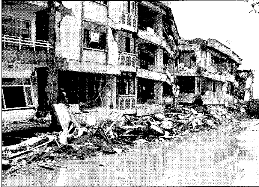
Figure 4-7 Failure of soft first story
