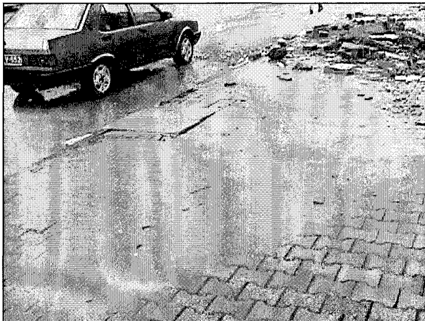
Figure 3-5 Sand boil on sidewalk in Adapazarı. Sand ejected from underground when sandy soils beneath the ground-water table liquefied during the earthquake.
