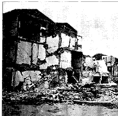
Figure 3-6 City of Pereira: Carrera 12/Calle 22, 3-Story Building, Collapsed
