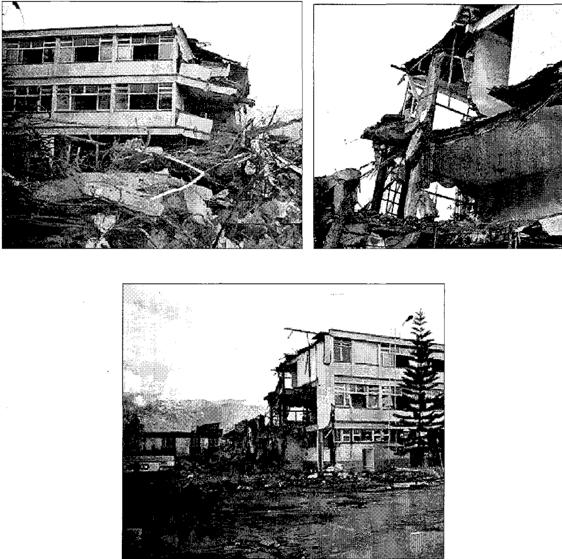
Figure 4-13 Collapse of Armenia's Centralized Police Station
