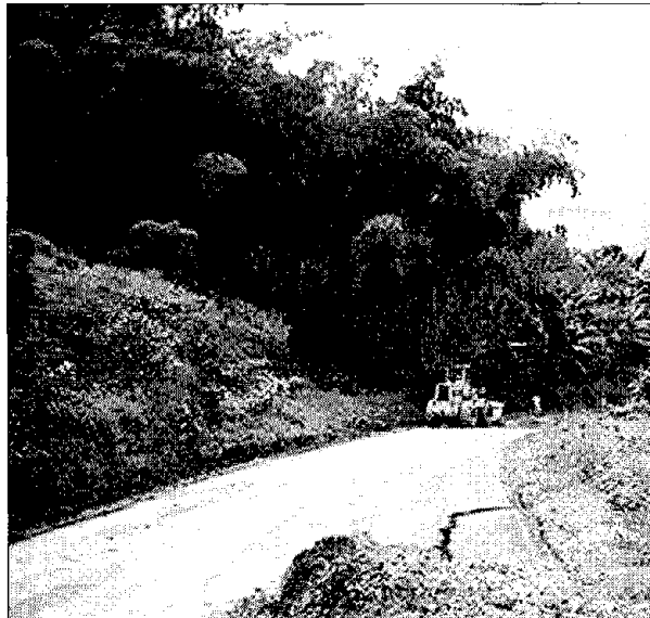
Figure 4-7 Crack on Pavement Due to Movement of Downhill Side of the Road on Road Armenia-Pijao
