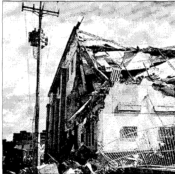
Figure 3-14 Damage to San Francisco Solano School in Armenia. URM Building
