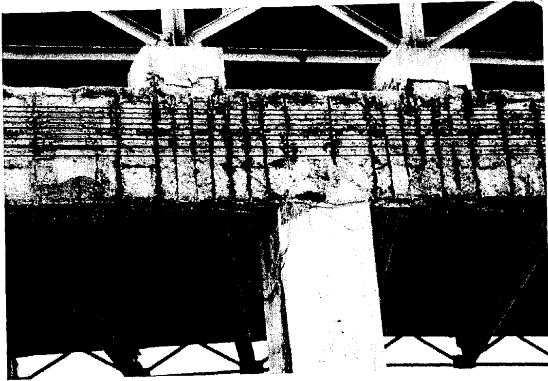
Figure 18. Finished concrete supports on Bent #5
