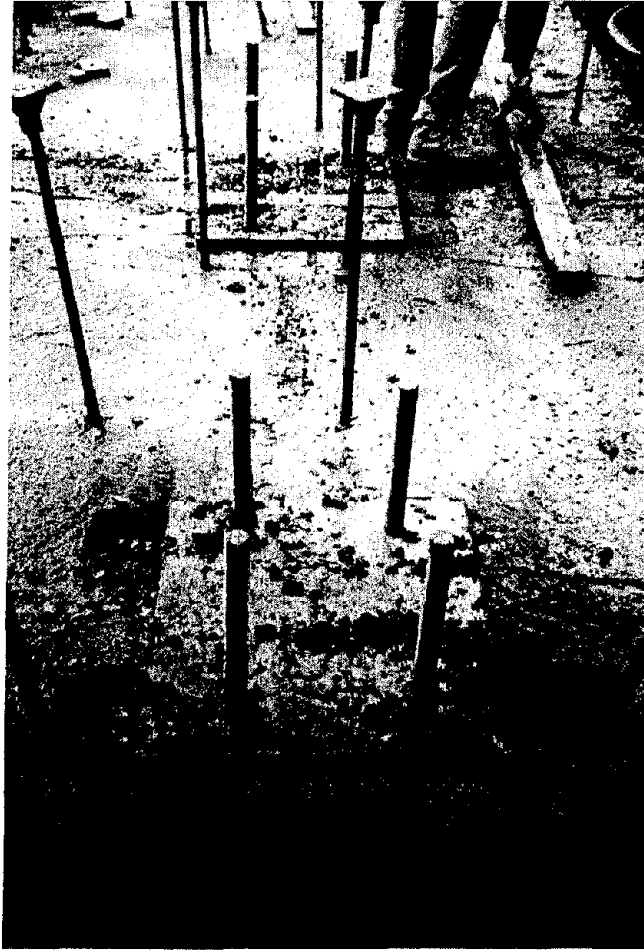
Figure 43. Detail of embedded channel and 1 1/2 in. diameter threaded rods in one leg of the load frame footing
