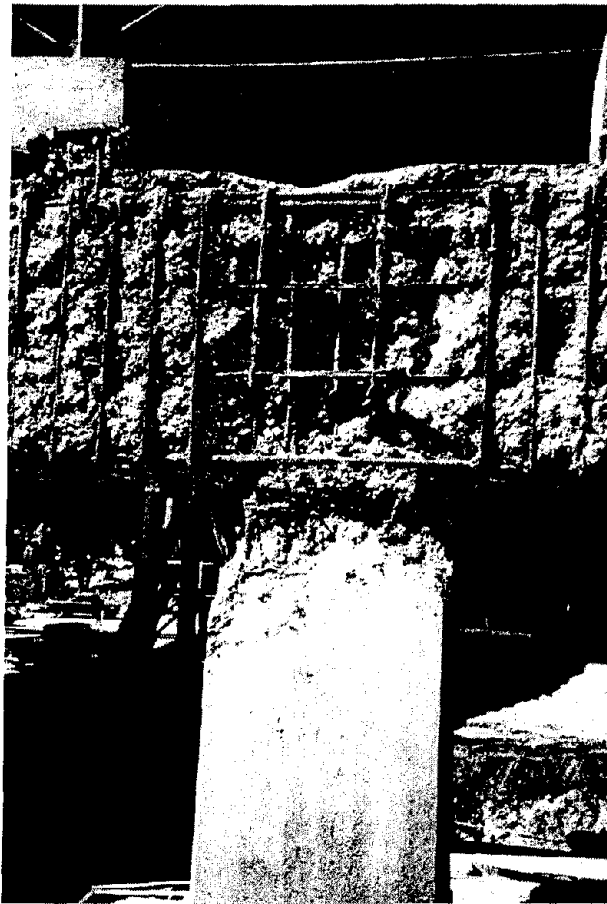
Figure 67. Bond deterioration and bar slippage at interior beam cap – column joint
