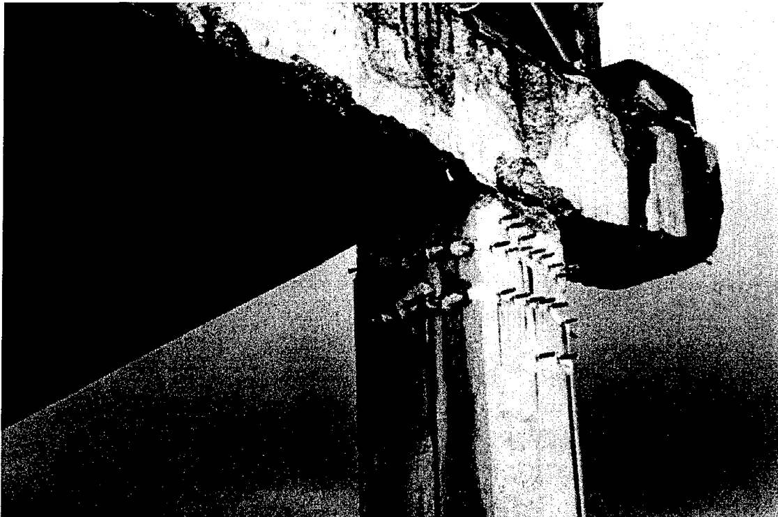
Figure 122. Repair of Bent #5R showing injection balloons on east column
