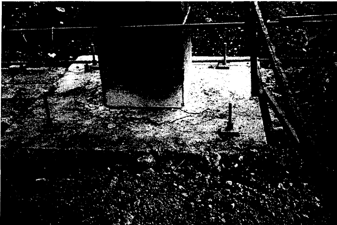
Figure 14. Detail of Dywidag bars in the pile cap
