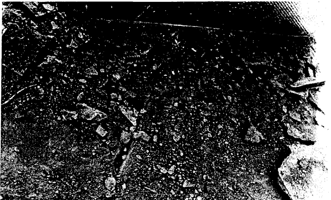
Figure 134. Radial cracks at pile cap surface of Bent #5R
