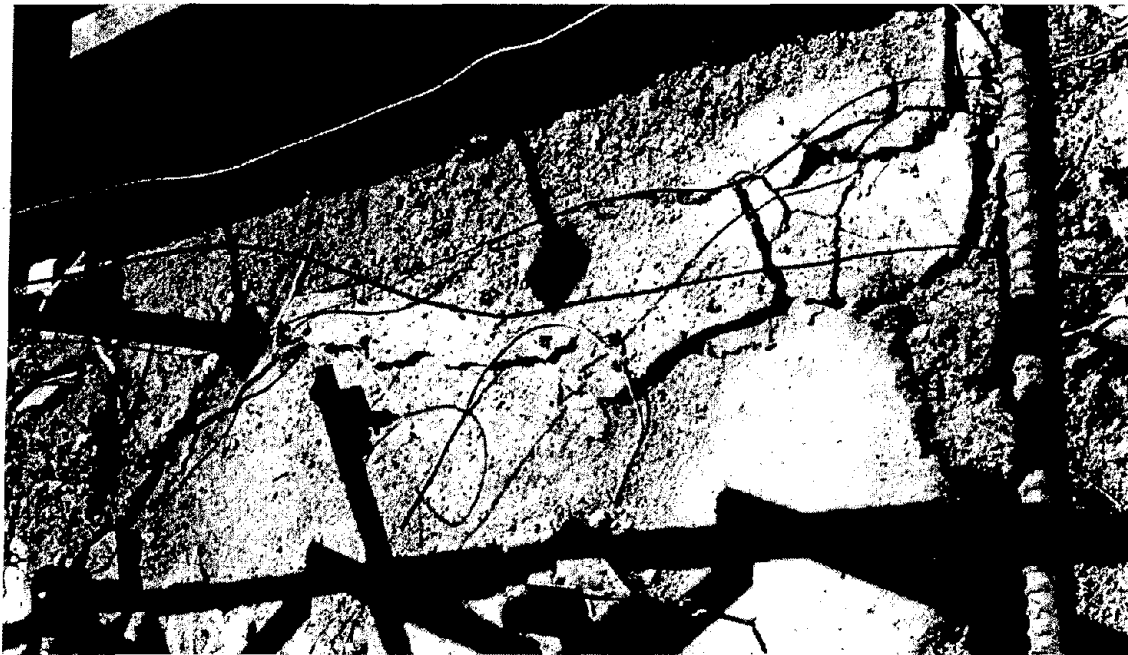
Figure 136. Damage in rigid link beam between pile cap and load frame footing
