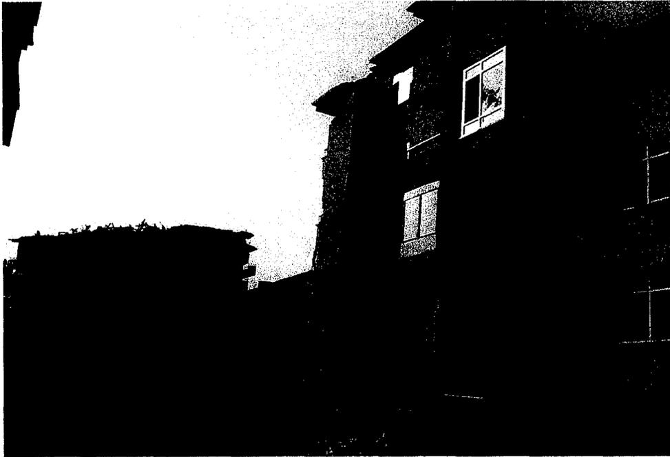
**Figure 10 Severe Damage to Multi-Story Apartment Buildings. Lower Floors have “Pancaked” and Building is not tilted. May be visible from aerial photos; collapse of lower floors may be detectable from radar imagery (Photo: R. Eguchi).**
