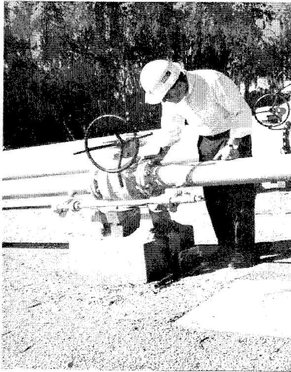
Post-Earthquake Investigation of the Behavior of Piping Systems
