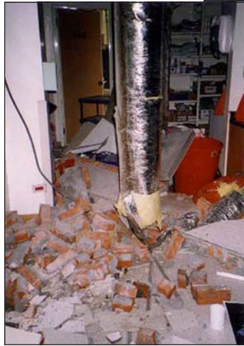
■ Figure 5. Interior damage in the Shiu-Tuan Hospital. Shown are (left) fallen brick inside the hospital and (right) a damaged interior glass brick wall.
