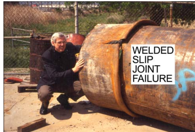
■ Figure 1. Compressive failure of the 1,245 mm Granada Trunk Line
