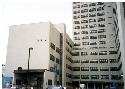
■ Figure 15. Plaza and the middle tower of the hospital
