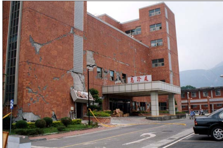
Photograph by M. Bruneau
