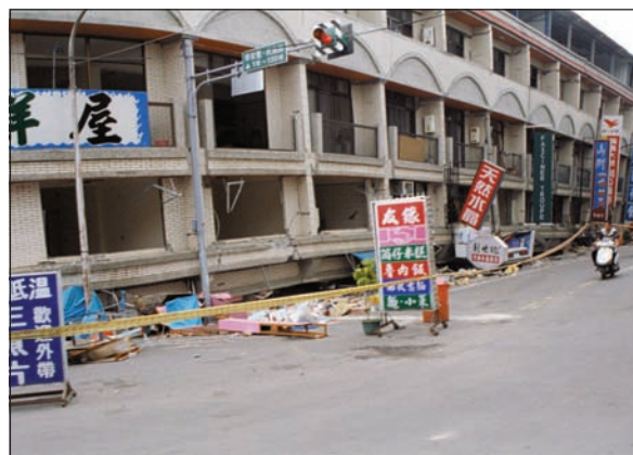
Photograph by M. Bruneau
