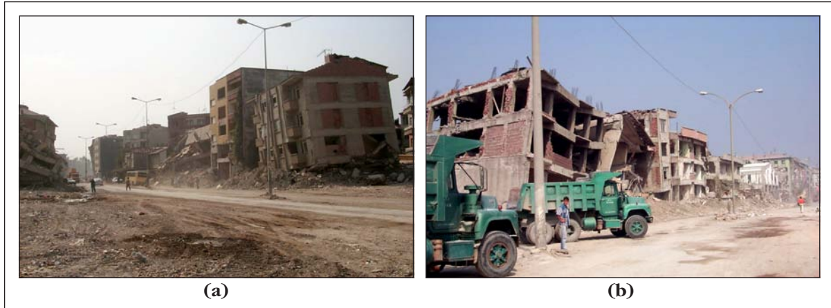
■ Figure 15 . Damage to apartment buildings in the “Circle Area” of Adapazari. Left image is view (a) in Figure 14b. Right image is view (b) in Figure 14b.
