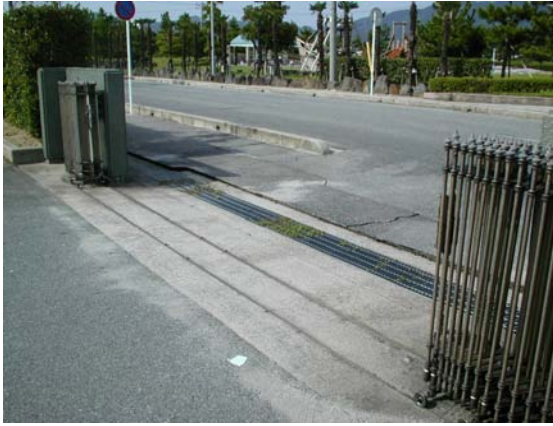
Photograph 1. Front gate and road (10 minutes after the earthquake)
