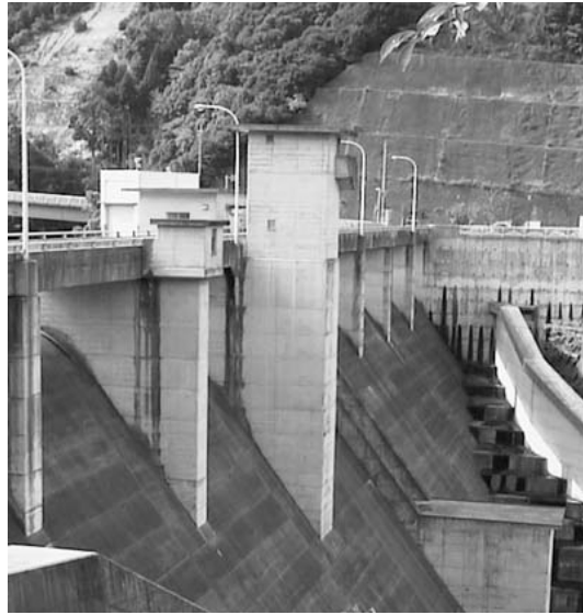
Figure 3 Kasho Dam viewed from the downstream right bank.
