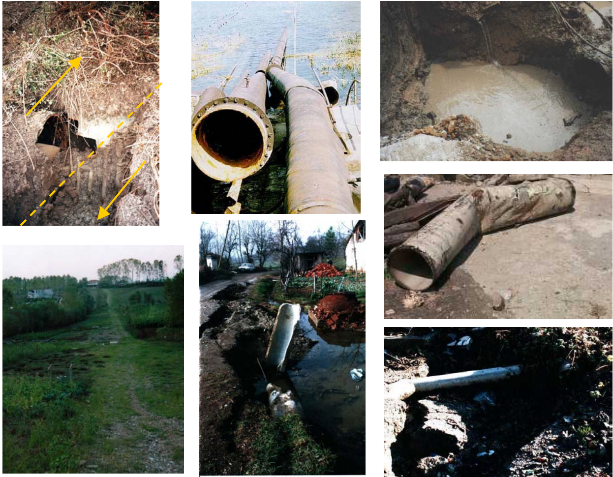
Figure 10 Damage to pipes in the 1999 Kocaeli and 1999 Düzce earthquakes
