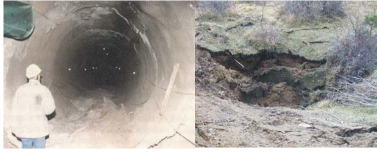
Figure 7: Collapse of Bolu tunnel in squeezing ground
