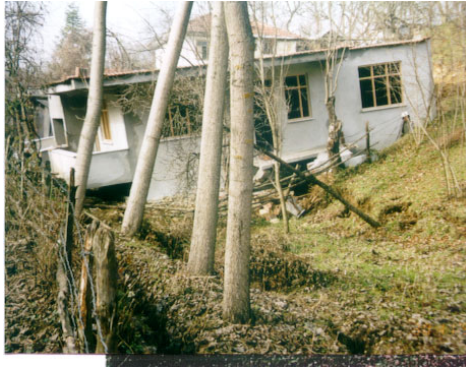
Figure 11: The behaviour of a single story reinforced building at Fındıklı
