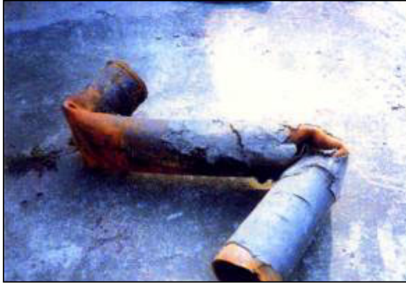
Photo.2 Deformation of a buried gas pipeline near Wu-Xi Bridge in Taiwan
