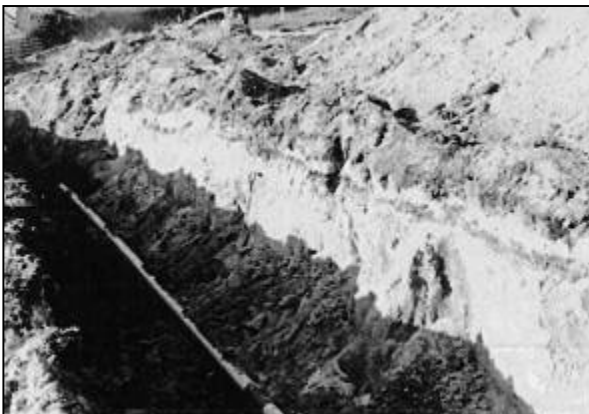
Photo.4 Buried gas pipeline survive the surface fault rupture at Wakatane in New Zealand
