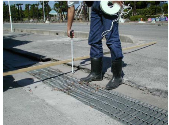
Photograph 4. Increase of settlements of road (1 week after the earthquake)
