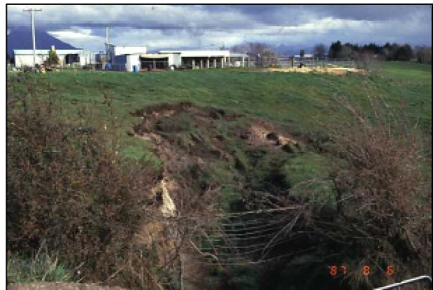
Photo.5 Surface fault rupture observed at the site shown in Photo.4
