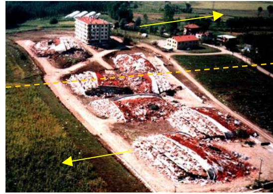
Figure 12: The collapse of apartment blocks at Kullar village
