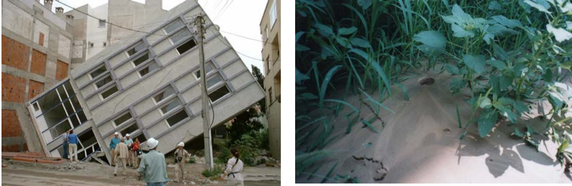
Figure 2: Examples of liquefaction in Adapazari
