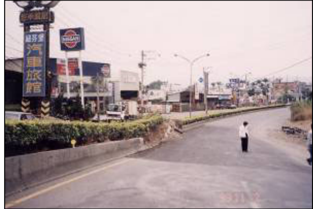
Photo.3 Surface fault associated with the damage to the buried gas pipelines
