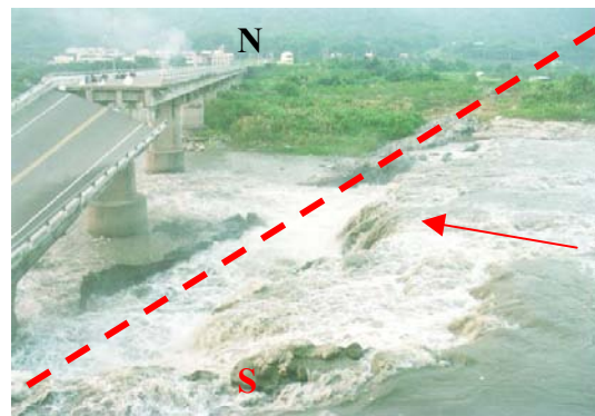
Figure 5 Collapse of Pefong Bridge (note the uplifted ground on RHS)
