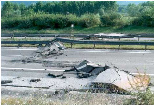
Figure 2: Buckling of roadway surfacing
