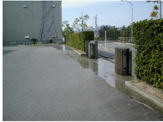
Photograph 2. Sand boil from crack of road (25 minutes after the earthquake)
