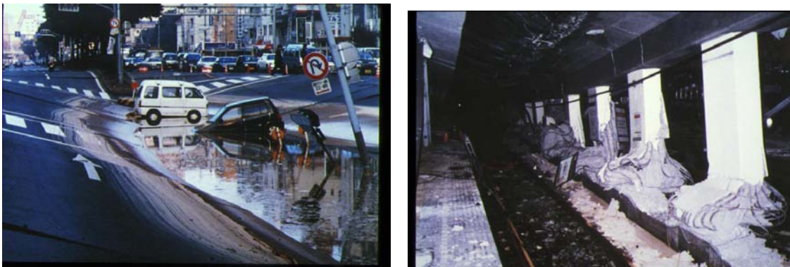
Figure 8 The collapse of Daikai station
