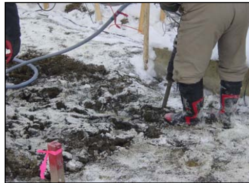
Figure 6. Breaking up Frozen Ground Surface Using Jack Hammer.
