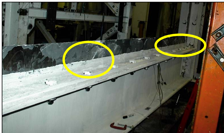
Figure 5. Poor epoxy coverage – Specimen F1
