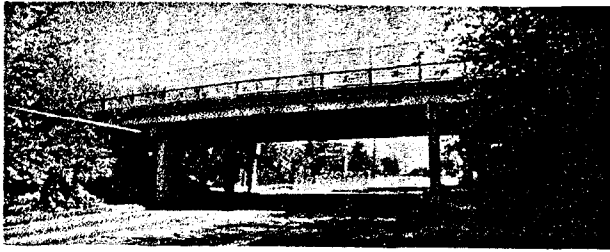
Fig. 1: Steel-Stringer Test Bridge
