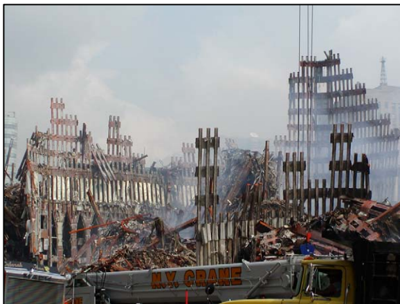
Figure 5-5. Three-column panels in down-down-down-down pattern
