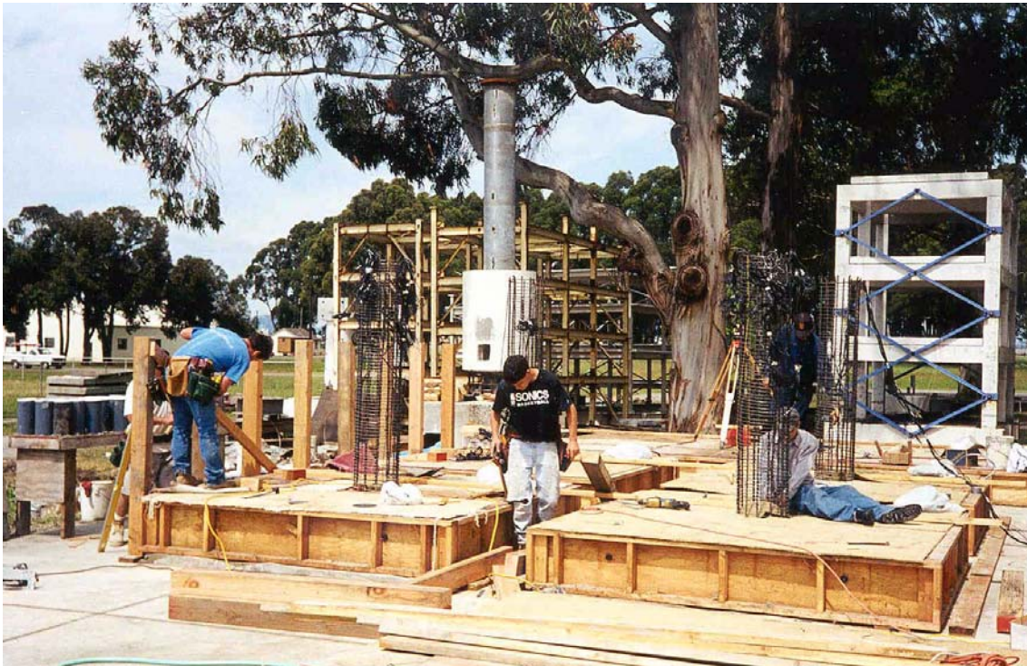
Figure 3-17. Construction of formwork to support the top slabs, while curing the footings.
