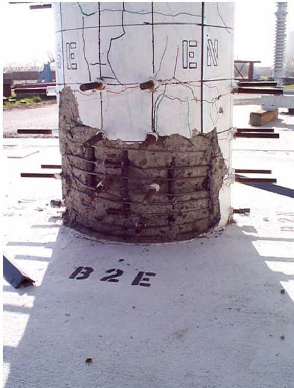
Figure C-79. Specimen B1 after Run 13 (east face).
