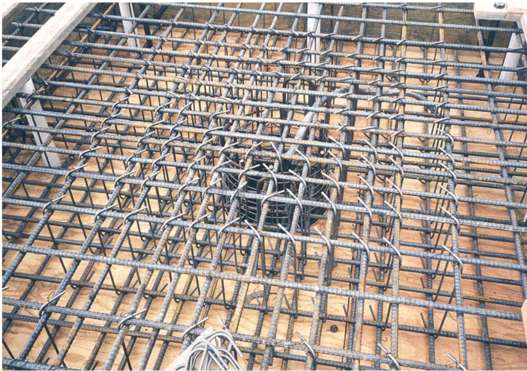
Figure 3-21. View of the top slab steel layout.
