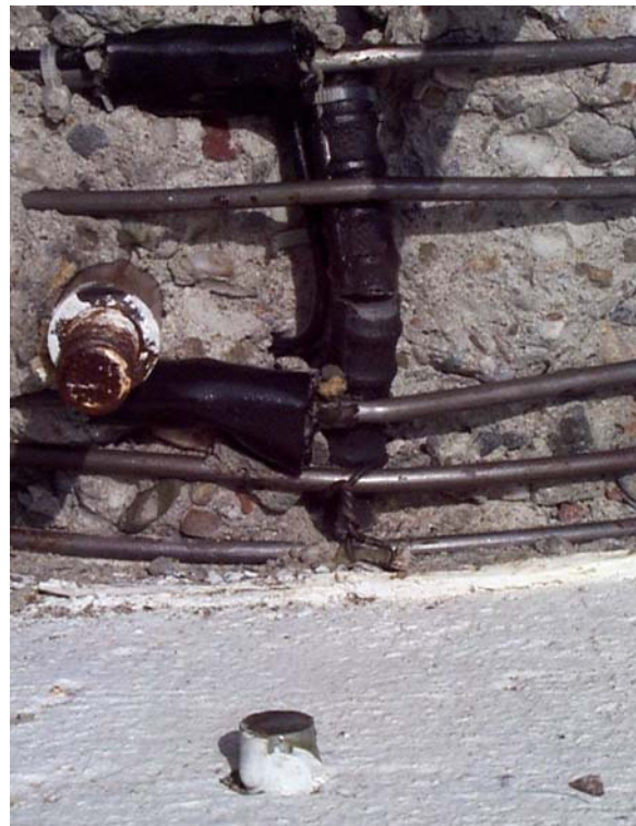
Figure C-82. Close-up on bar #9 on the west side which fractured in Run 12.
