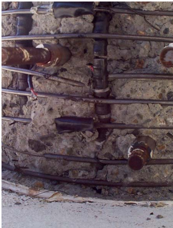
Figure C-81. Close-up on bar #3 on the east side which fractured in Run 12.
