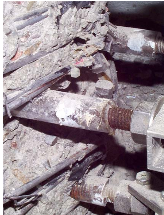
Figure C-54. Close-up on bar #9 on the west side which fractured in Run 9. The distance between the ends of the bar is caused by the residual displacement at the end of the test.
