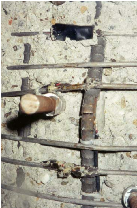
Figure C-33. Specimen A1 after Run 8. Fractured bar #3 on the east face is shown.
