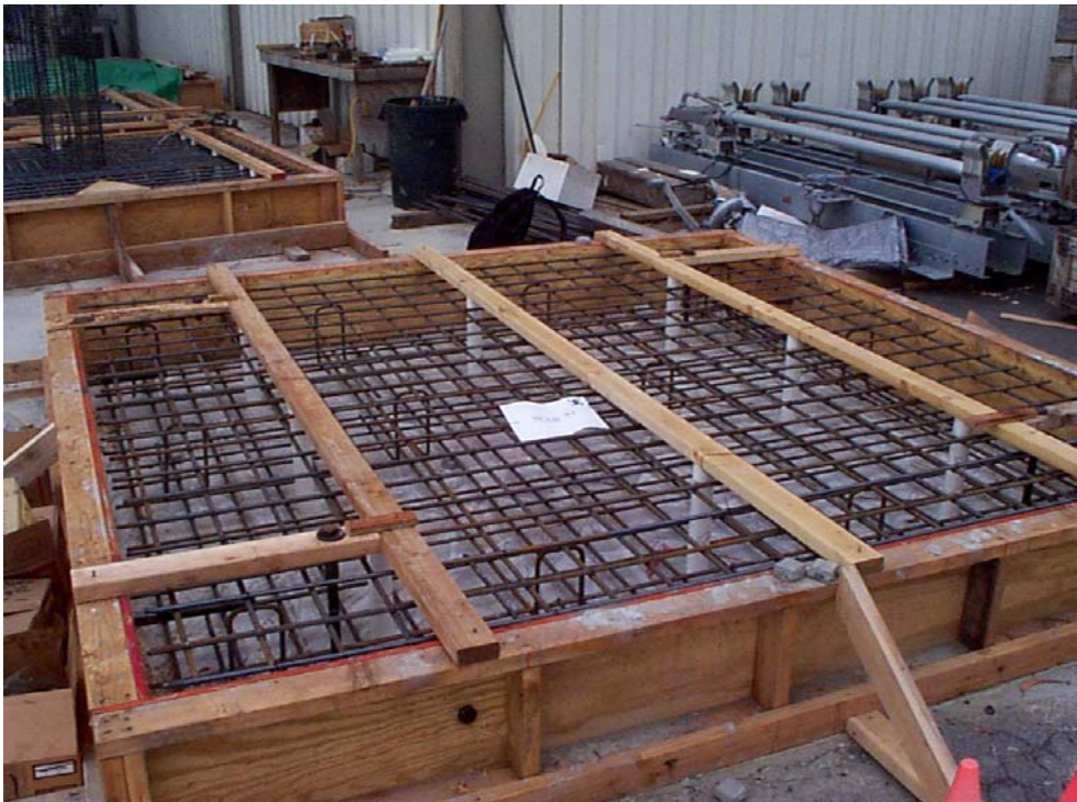
Figure 3-15. Steel details for one of the three similar weight blocks.
