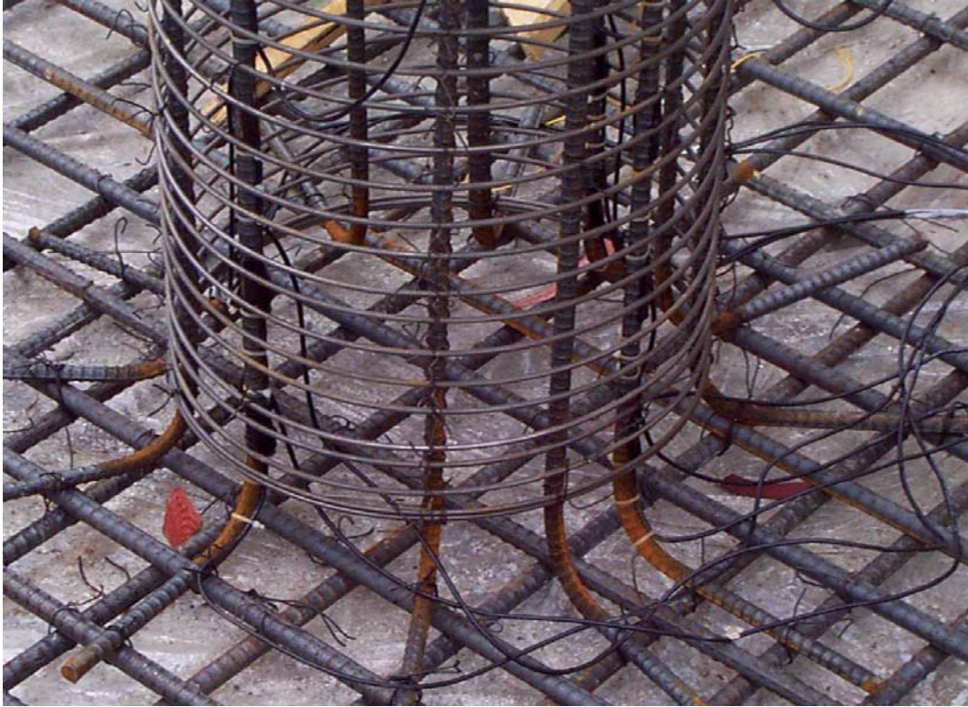
Figure 3-12. The column steel cage set on the bottom steel of the footing.
