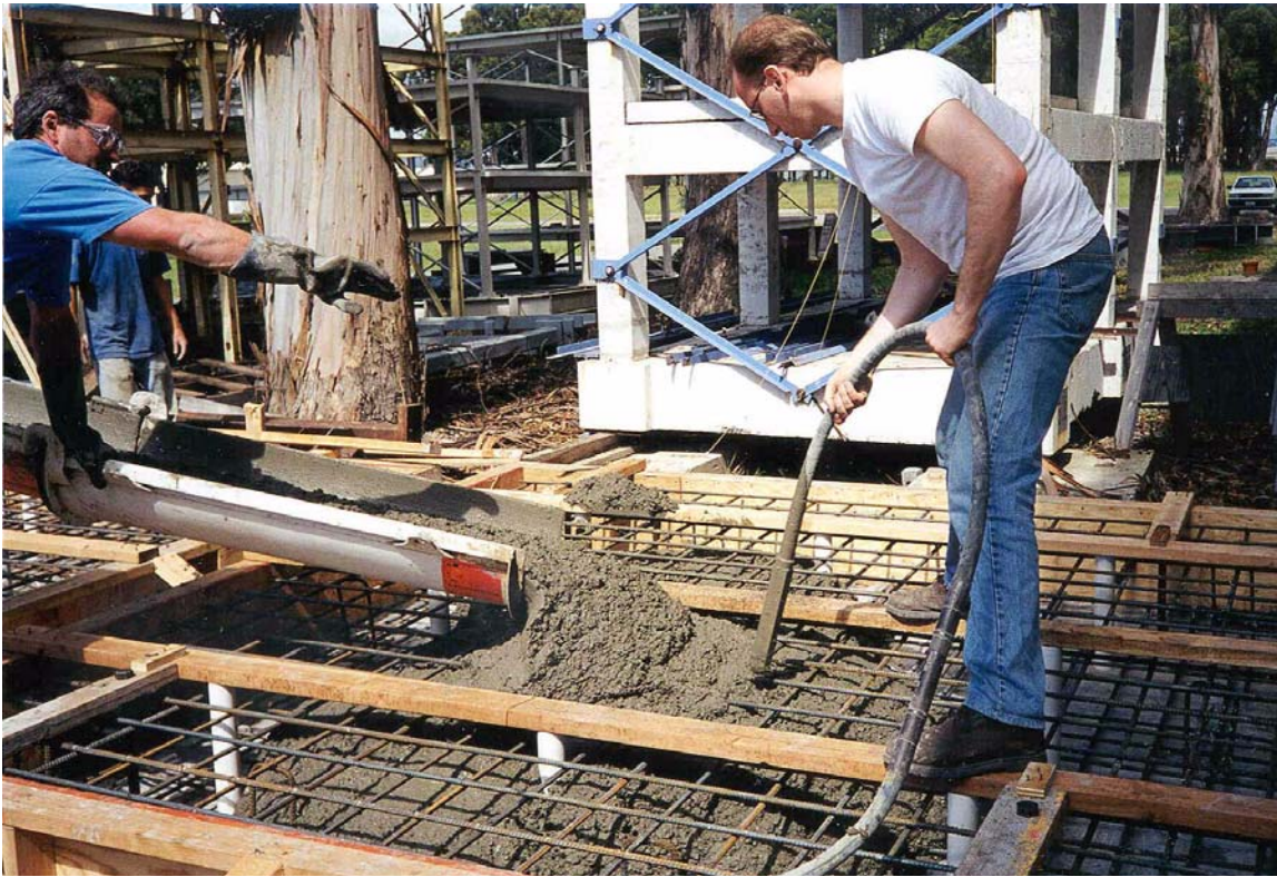
Figure 3-16. Casting the weight blocks.
