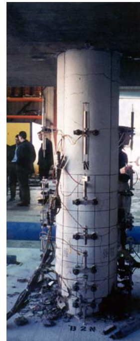
Figure C-74. Specimen B2 after Run 9 (north face).
