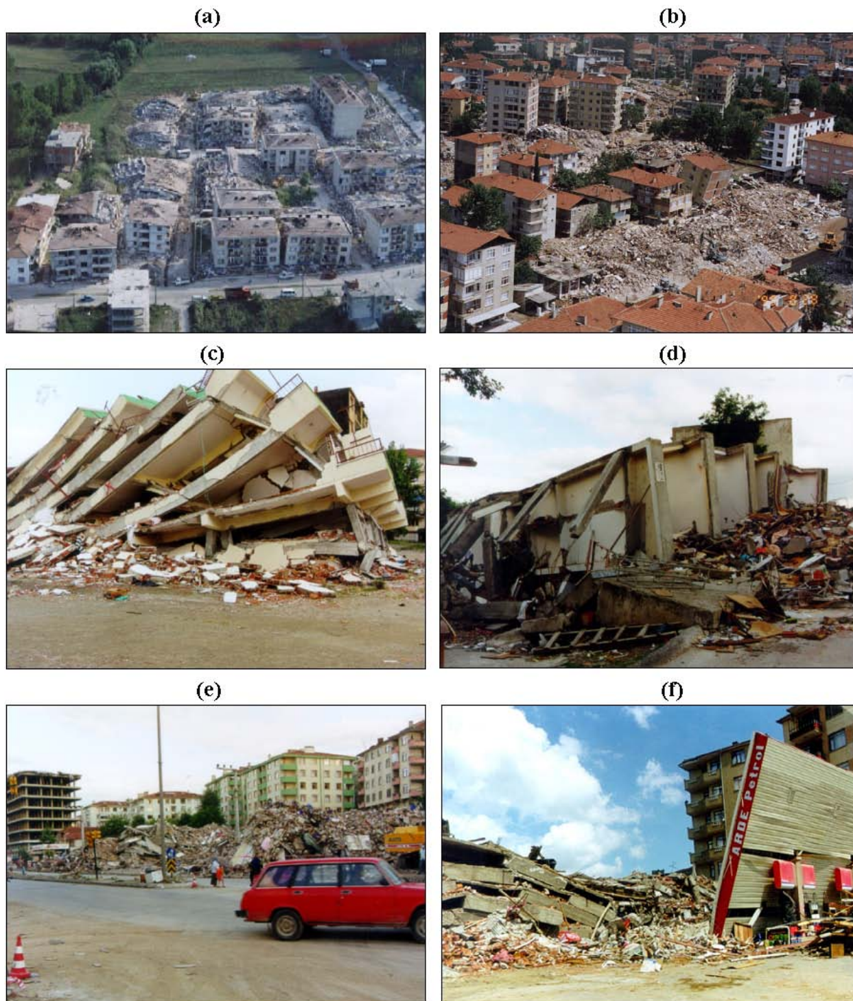
FIGURE 3-2 Photo mosaic, showing damage sustained in Golcuk and surrounding areas, during the 1999 Marmara earthquake: (a-b) aerial view of extensive apartment collapse (Courtesy of R. Andrews); (c-e) ground-based perspective of debris piles accompanying apartment collapse; (f) damage sustained by other structures, such as a gas station. Building damage such as this is recorded as changes in optical and SAR remote sensing imagery, acquired before and after the earthquake.
