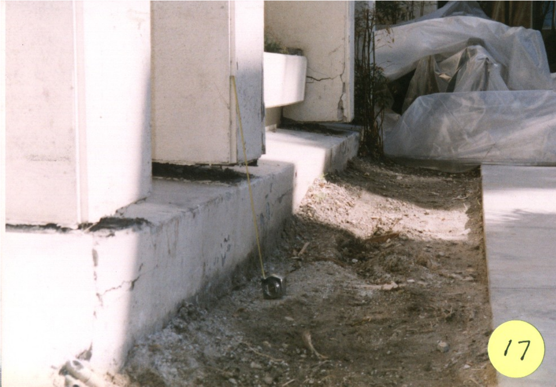
Figure 8-3 Liquefaction-Induced Settlement of On-Grade Structures Relative to Pile-Supported Hospital Building in Northridge District of Los Angeles
