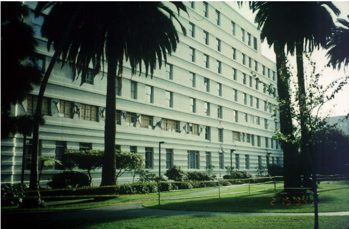
Figure 2-2 Saint John's Hospital and Health Center in Santa Monica, California, Damaged by the Northridge Earthquake in 1994
