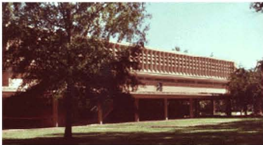
Olin Library prior to renovation and retrofit
