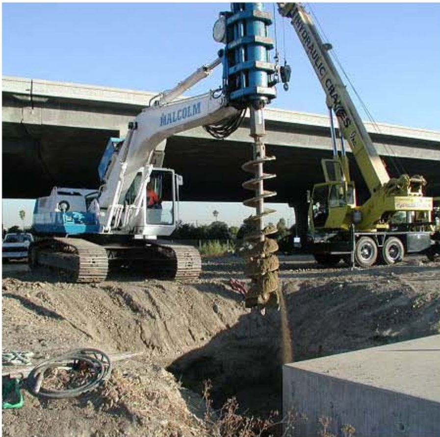
Drilling the hole for the column
