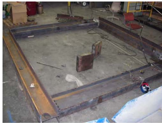
b) Frame during construction
