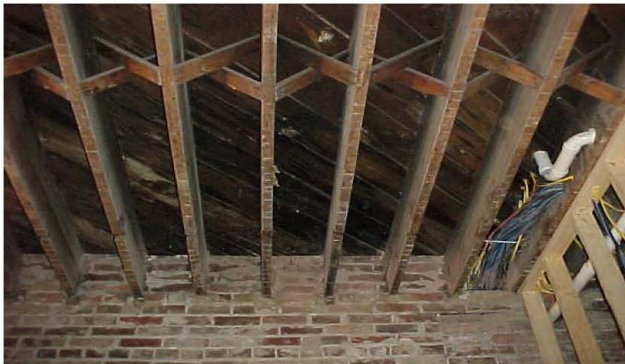
Figure 9: Floor joists connected to the supporting masonry wall
