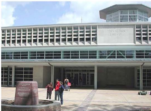
Olin Library after renovation and retrofit
