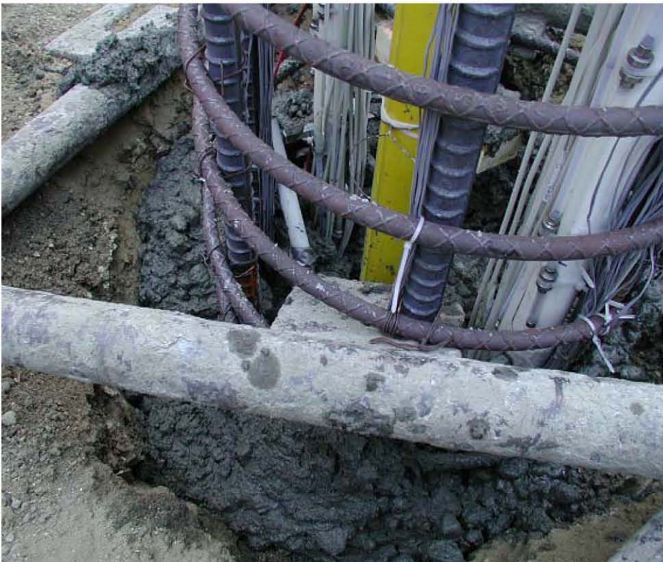
The concrete once it has been poured to the ground line.
