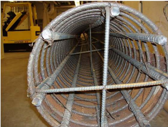
Figure 9. Empty rebar cage
