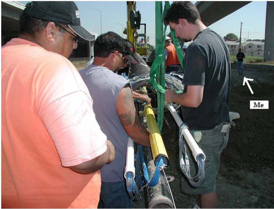
All the wires exiting at the top of the column.
