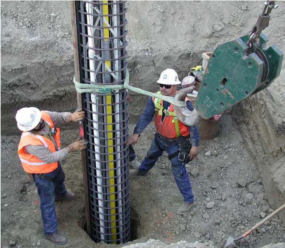
The column being inserted into the hole.
