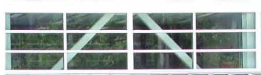
Steel cross bracing at Olin Library
