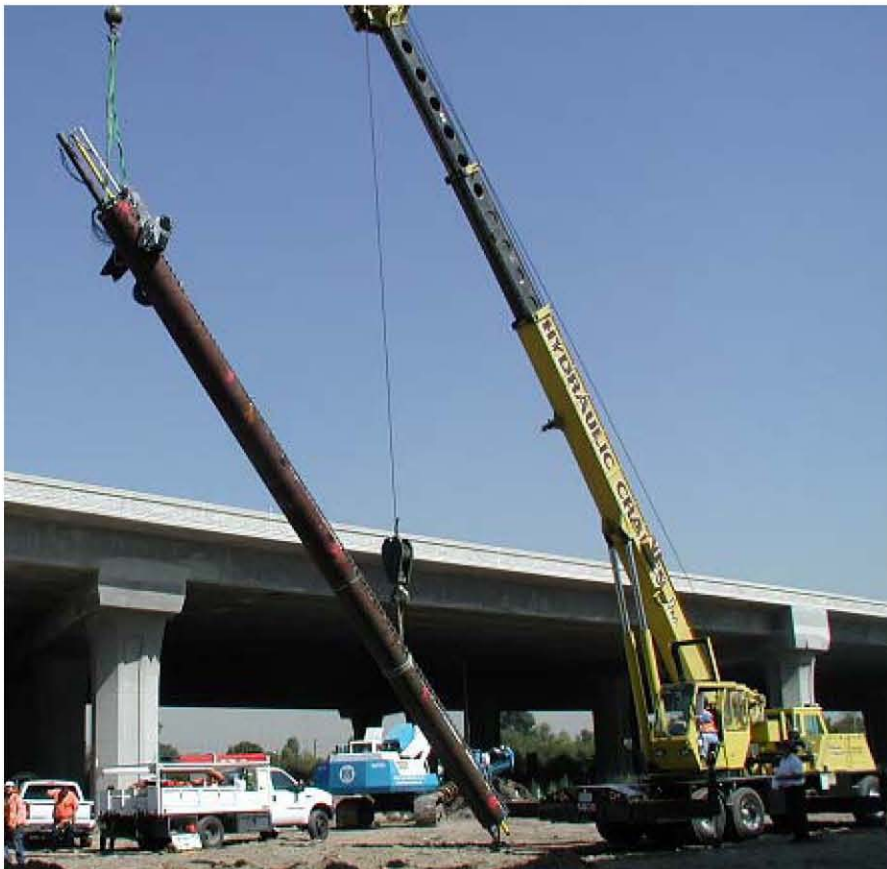
The crane lifting the column into place.
