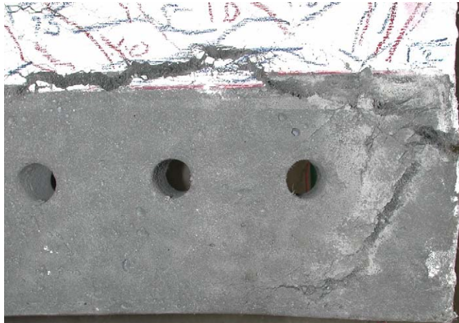
Figure 5-17. Cracking in connection region of Panel 2 after test
