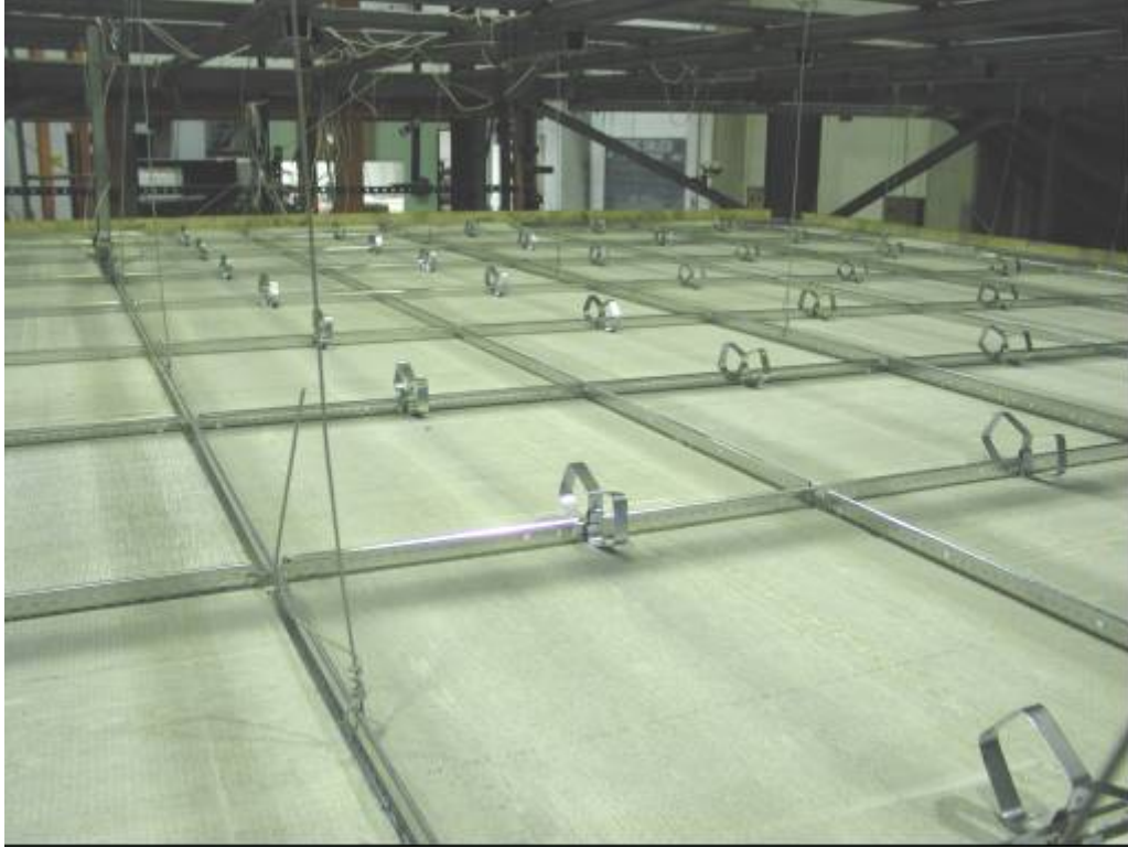
FIGURE 6-2 Configuration 2 installation, undersized tiles with retainer clips
