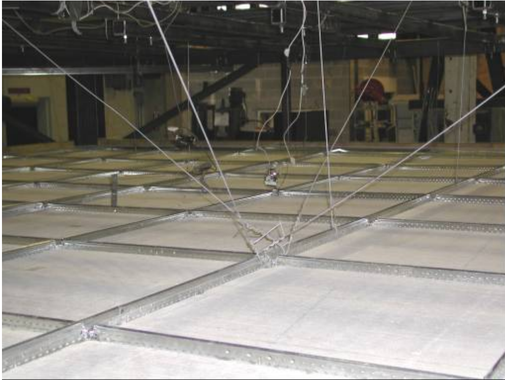
FIGURE 6-4 Configuration 6 installation, normal sized tiles without compression post
