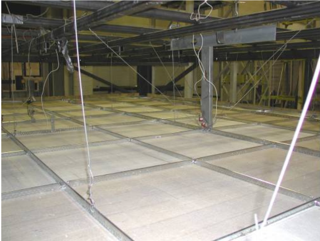
FIGURE 6-3 Configuration 4 installation, normal sized tiles
