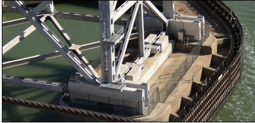
Figure 7-10. 1958 Carquinez Straits Truss Bridge showing Rocking Steel Box Beams that Provide Isolation and Damping of the Steel Braced Towers
