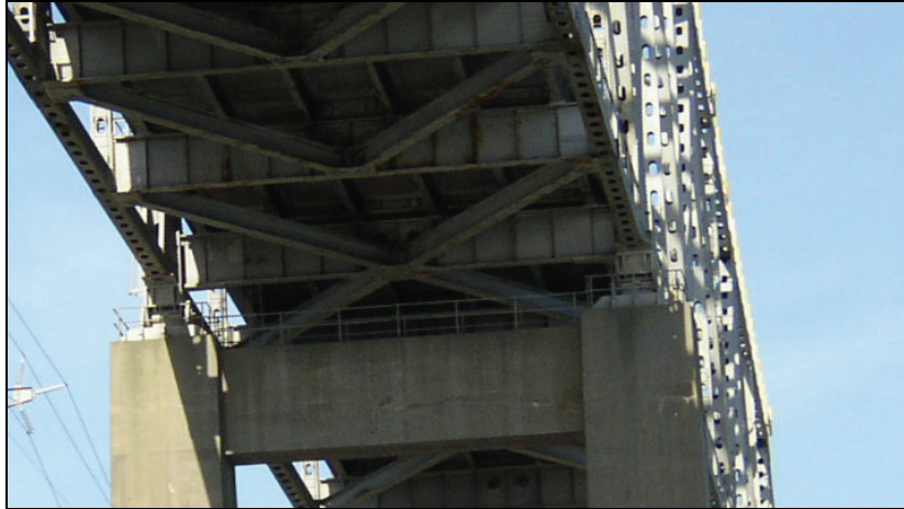
Figure 8-13. Bearings and Lateral Bracing System
