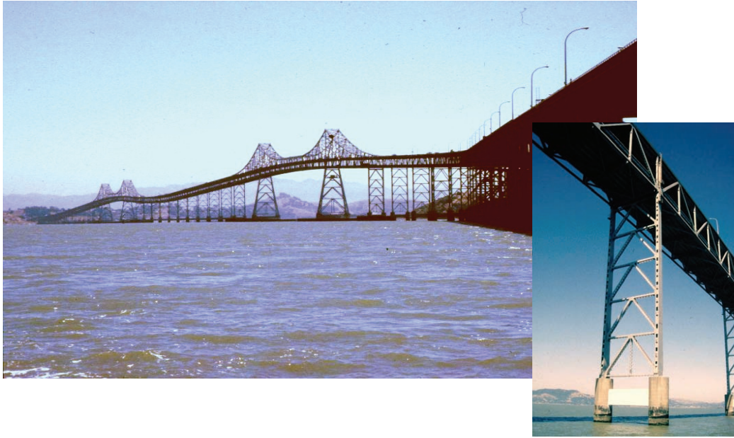
Figure 6-6. Support Towers of the Richmond-San Rafael Bridge
