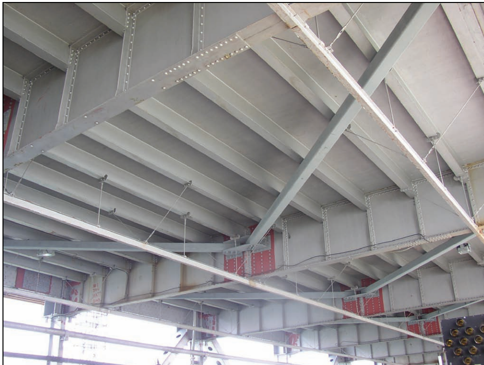
Figure 8-14. Typical Chevron Lateral Bracing Under the Deck of a Through Truss, Floor Beams and Stringers Support a Concrete Slab, the Three Rails Support a Maintenance Traveler
