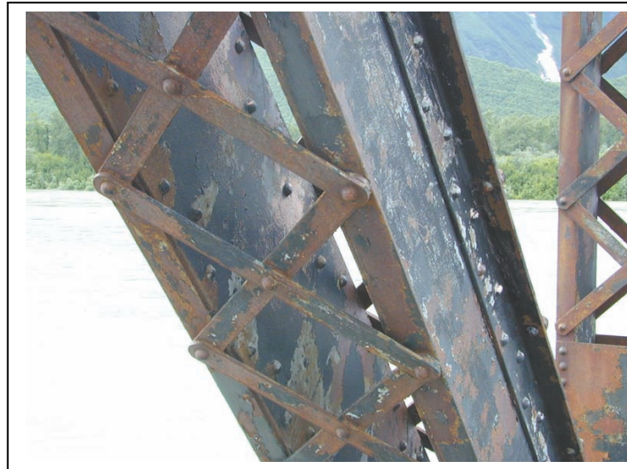
Figure 4-12. Typical Laced Member
