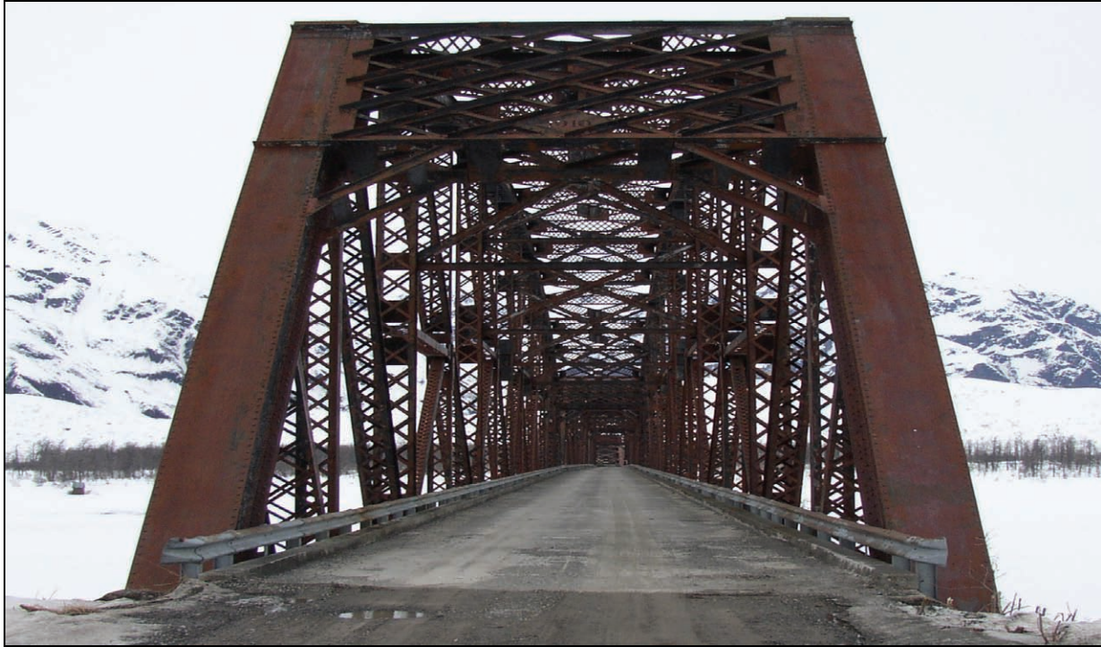
Figure 7-6. Million Dollar Bridge, Alaska, Portal Frame
