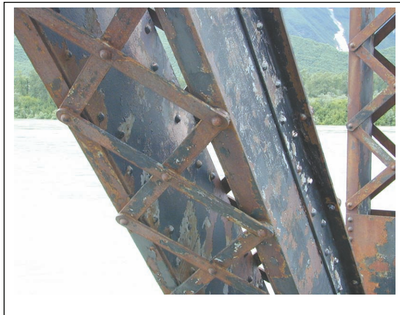
Figure 6-1. Typical Built-Up Member
