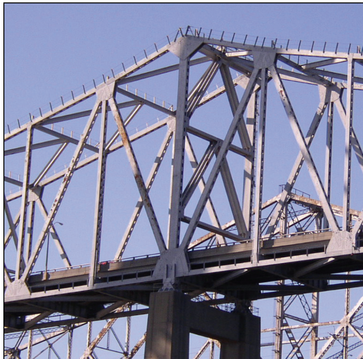
Figure 8-12. Cooper River Truss, Charleston, South Carolina, 1963 Main Tower Bearings and Vertical Lateral Bracing, Upper Chords Lateral Bracing System, and Safety Hand Railing on Upper Chords
