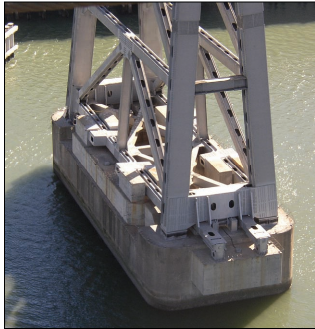
Figure 8-2. Seismic Retrofit of A-Frame Tower Rocking Supports
