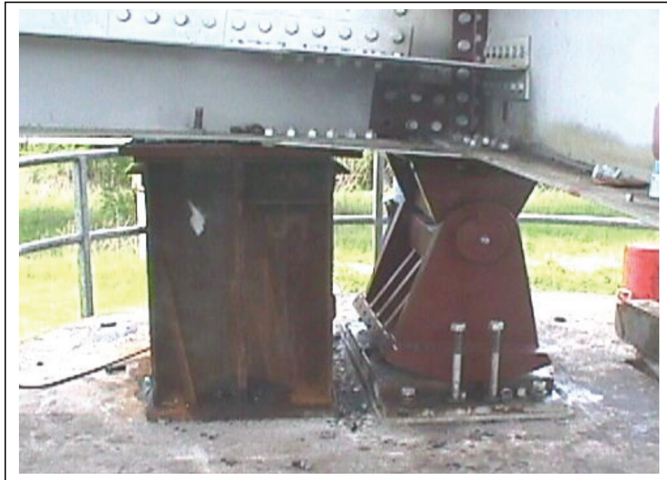
Figure 7-11. Rocker Bearing Replacement
