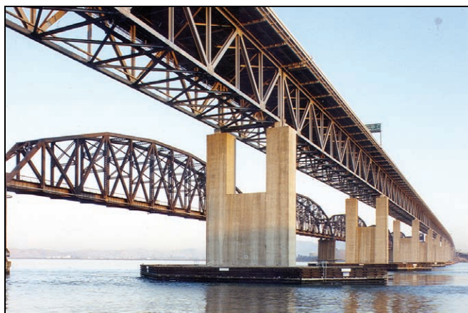
Figure 8-3. Benicia-Martinez Bridge, California, 1960; Gerber Framing, 528-ft truss Spans (1932 RR Camel-Back Truss in the Background)
