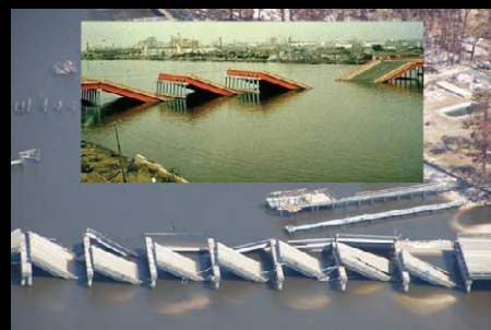
Figure 4. Bridge span collapses during Niigata earthquake (top) compared to similar damage due storm surge during Hurricane Katrina.
