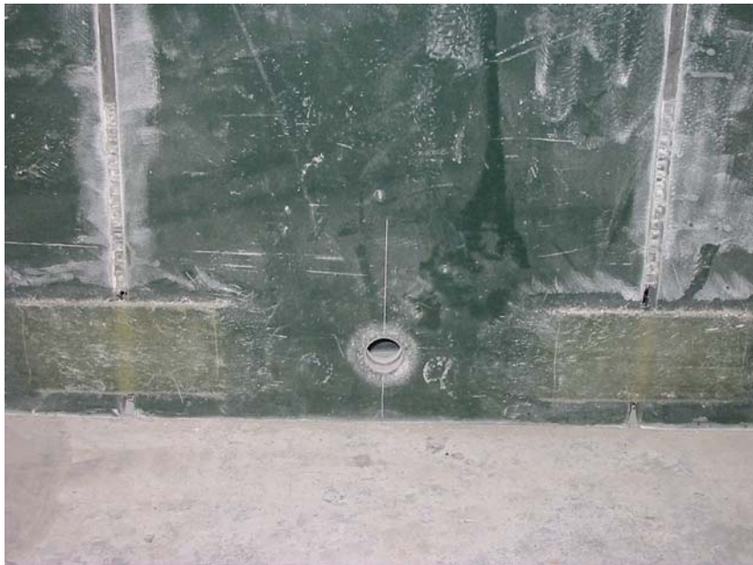
Figure 6-17 Bottom Connection of Outer Damping Panel (Pin)
