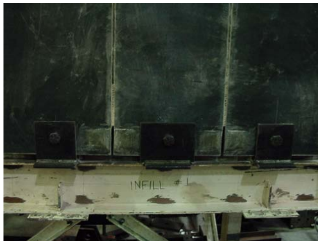
(c) Setup Outer Damping Panel to the Tested Frame by weld
