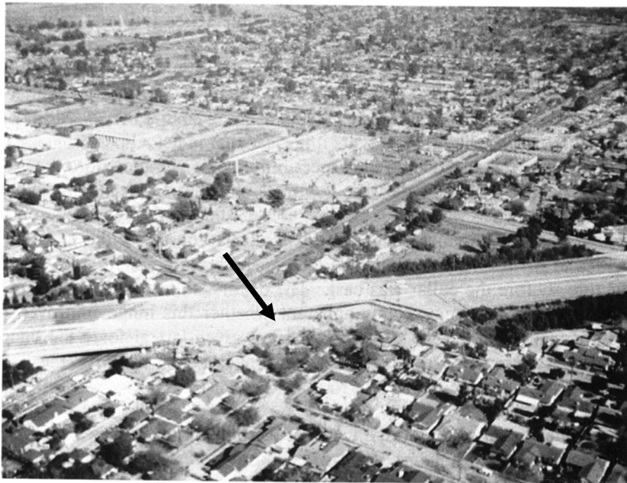
Fig. 1-2 Aerial View of the SR 118 Mission-Gothic Undercrossing Showing Collapsed Eastbound Bridge (1994 Northridge Earthquake)
