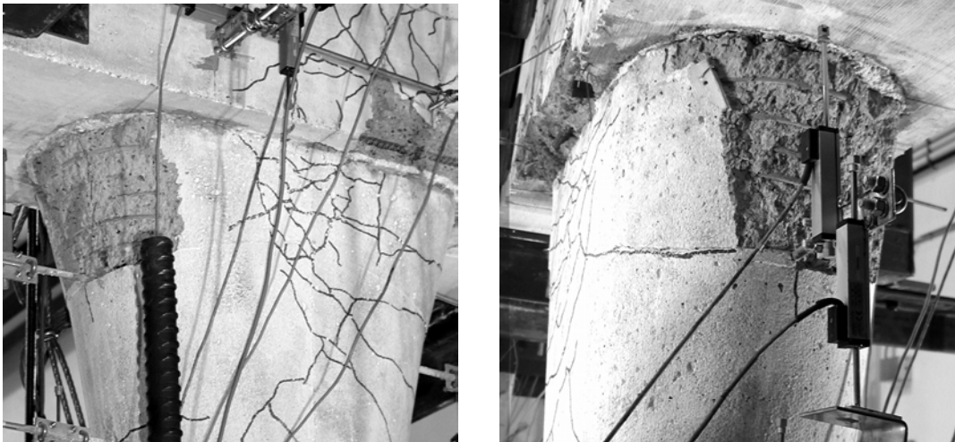
Fig. 4-104 SFCD1, Concrete Spalling at Top of the Flare
