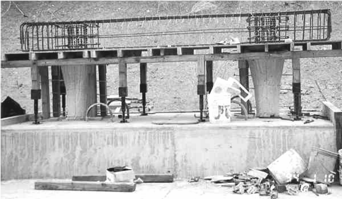
Fig. 3-5 Typical Beam Reinforcements
