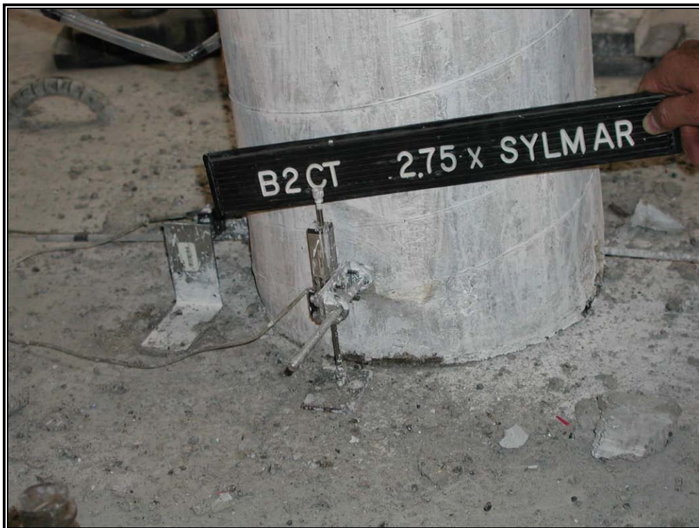
Fig. 4-61: West Side of East Column Base
