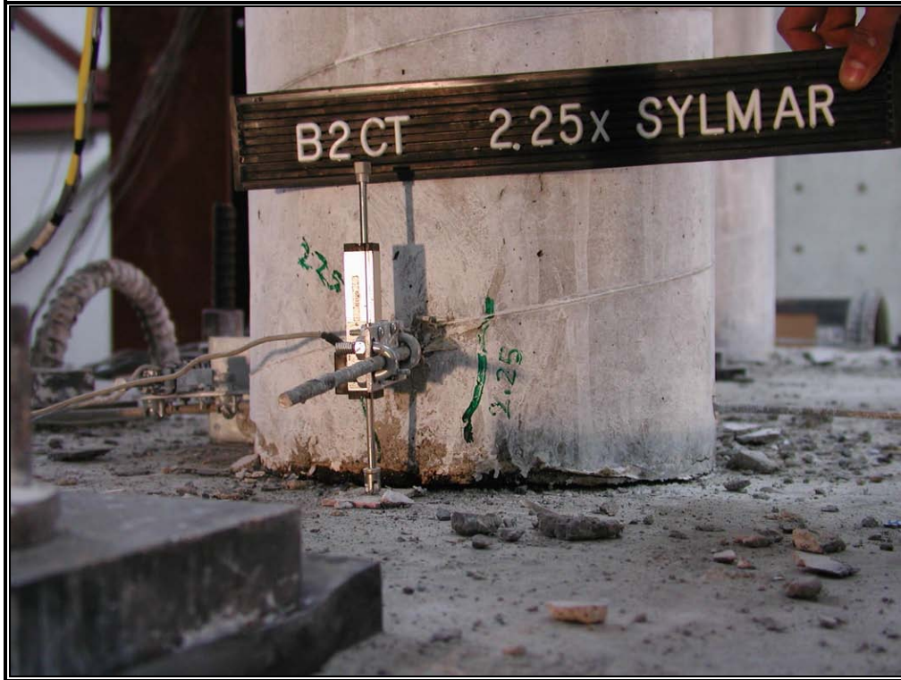
Fig. 4-52: Concrete Cracking on West Side of West Column Base
