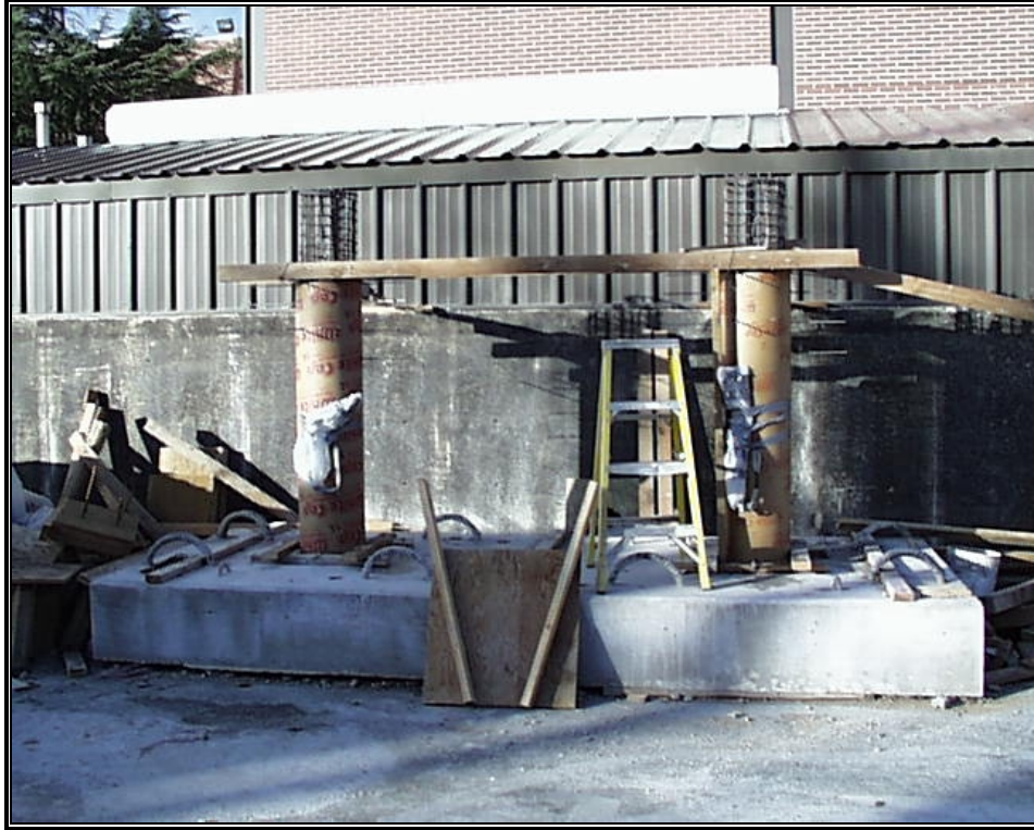
Fig. 3-13: Formwork of Medium Specimen Columns
