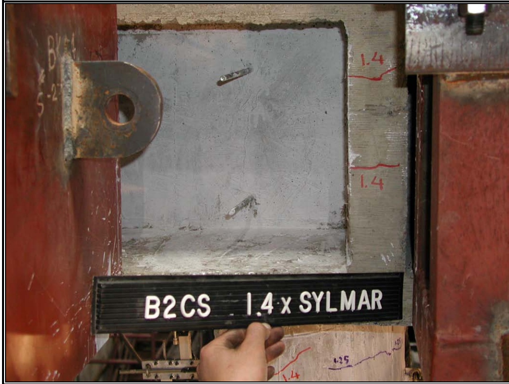
Fig. 4-6: Shear Cracks in West Column
