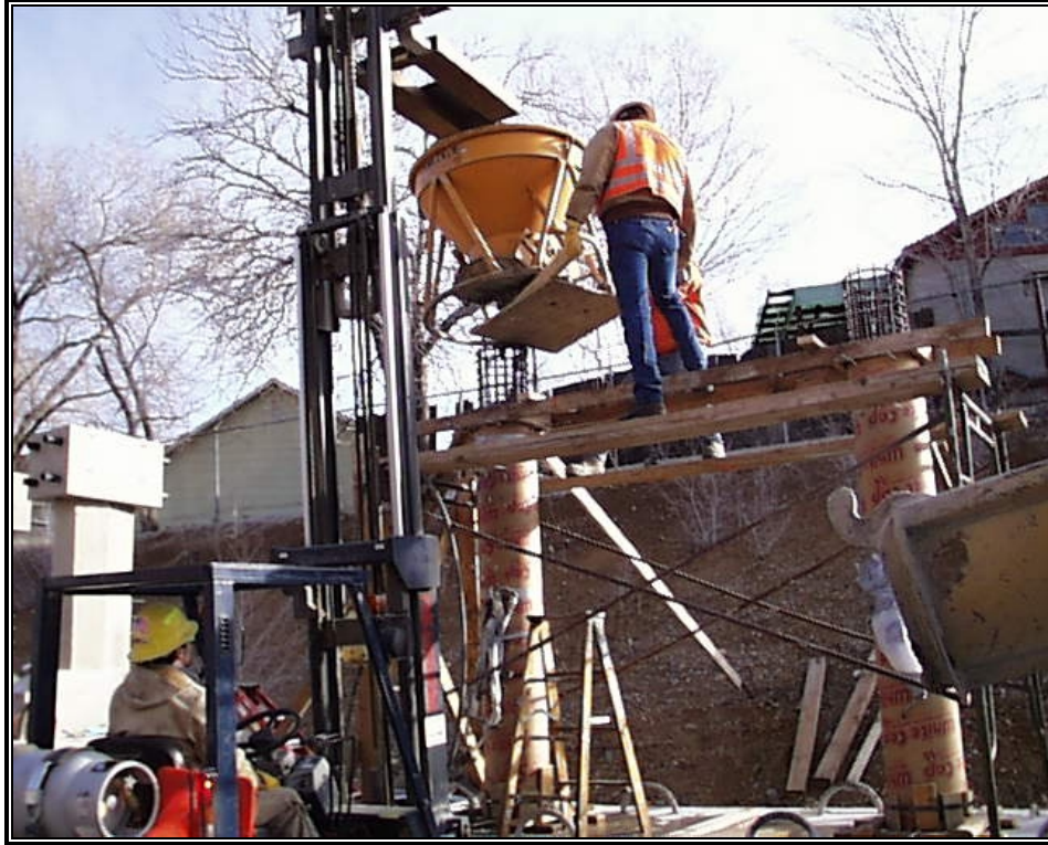
Fig. 3-15: Concrete Casting of Tall-Specimen Columns
