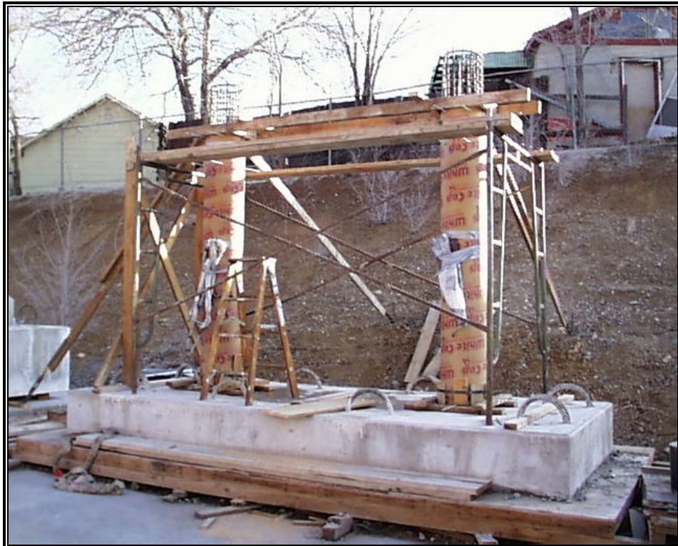
Fig. 3-14: Formwork of Tall Specimen Columns
