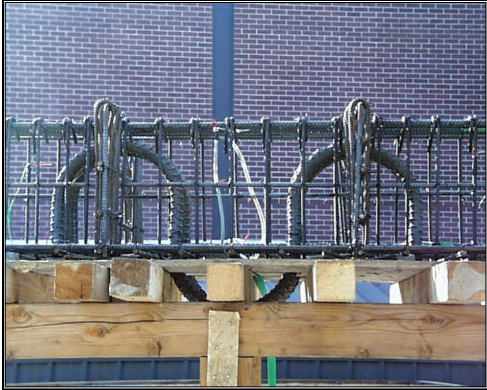
Fig. 3-21: Bent-Cap Reinforcement Details
