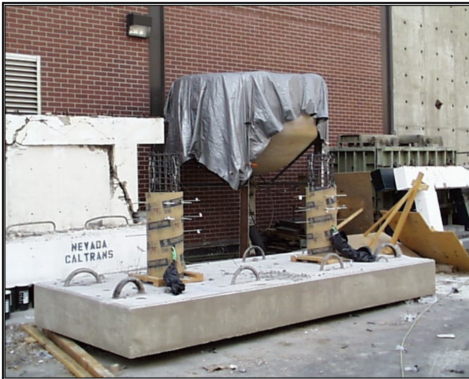
Fig. 3-12: Formwork of Short Specimen Columns
