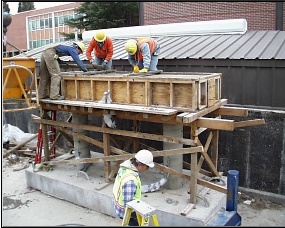
Fig. 3-23: Concrete Casting for Middle Specimen Beam
