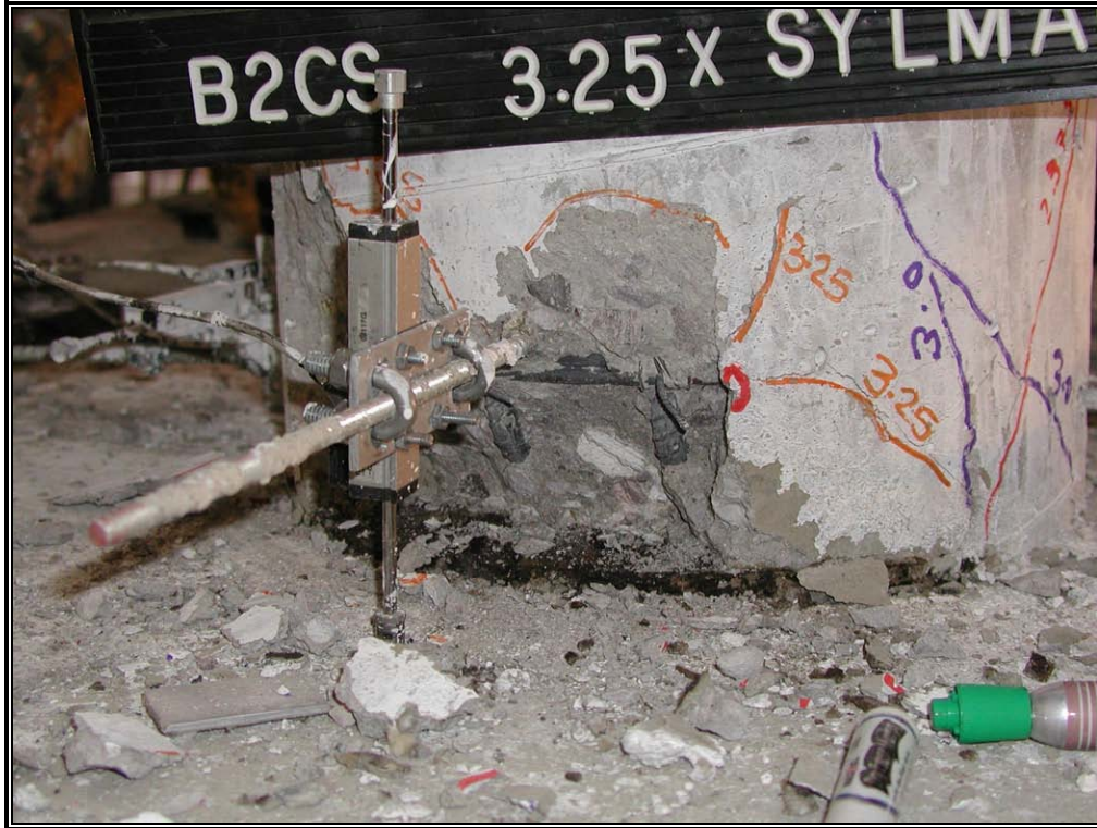
Fig. 4-12: Base Damage in West Column
