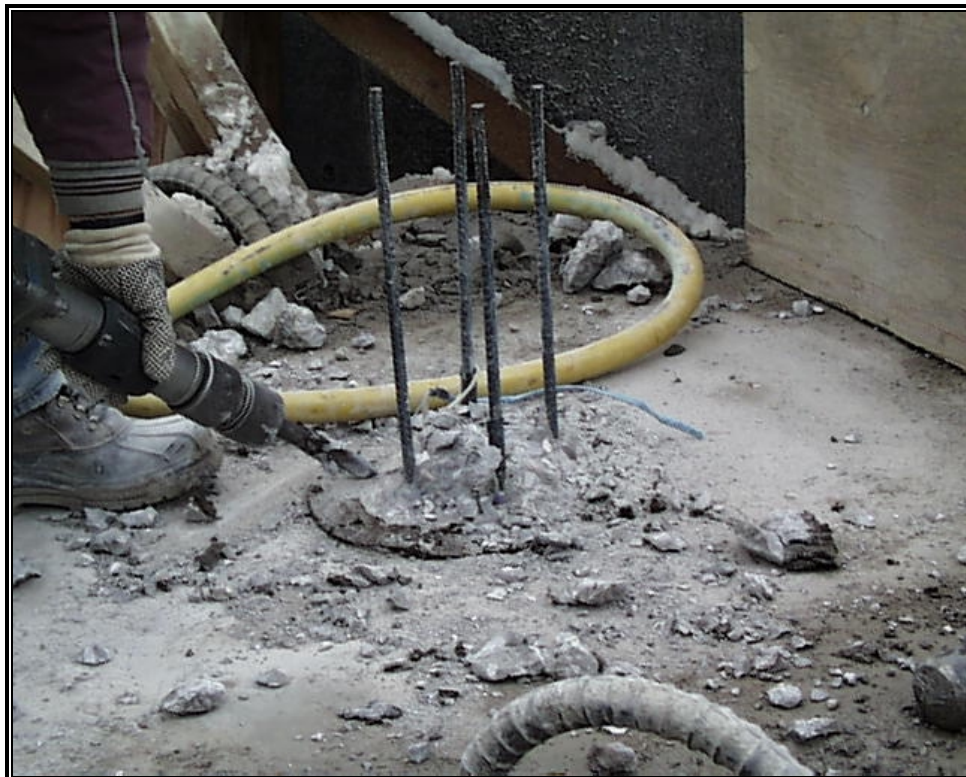
Fig. 3-18b: Removing Damaged Parts
