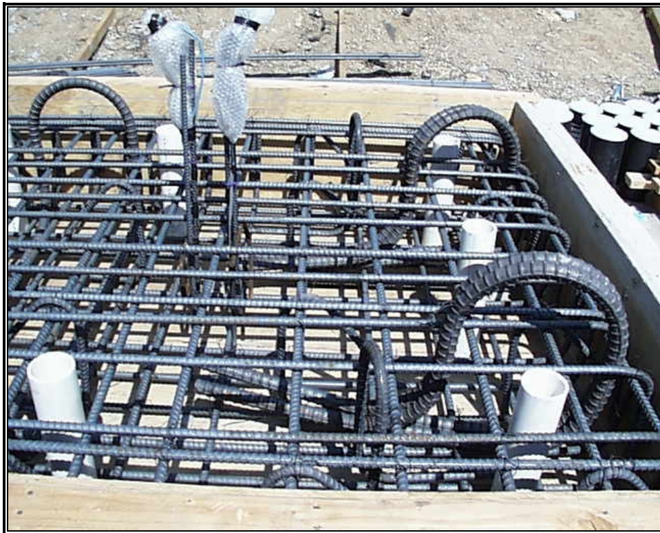
Fig. 3-4: Footing Hooks and Dowels
