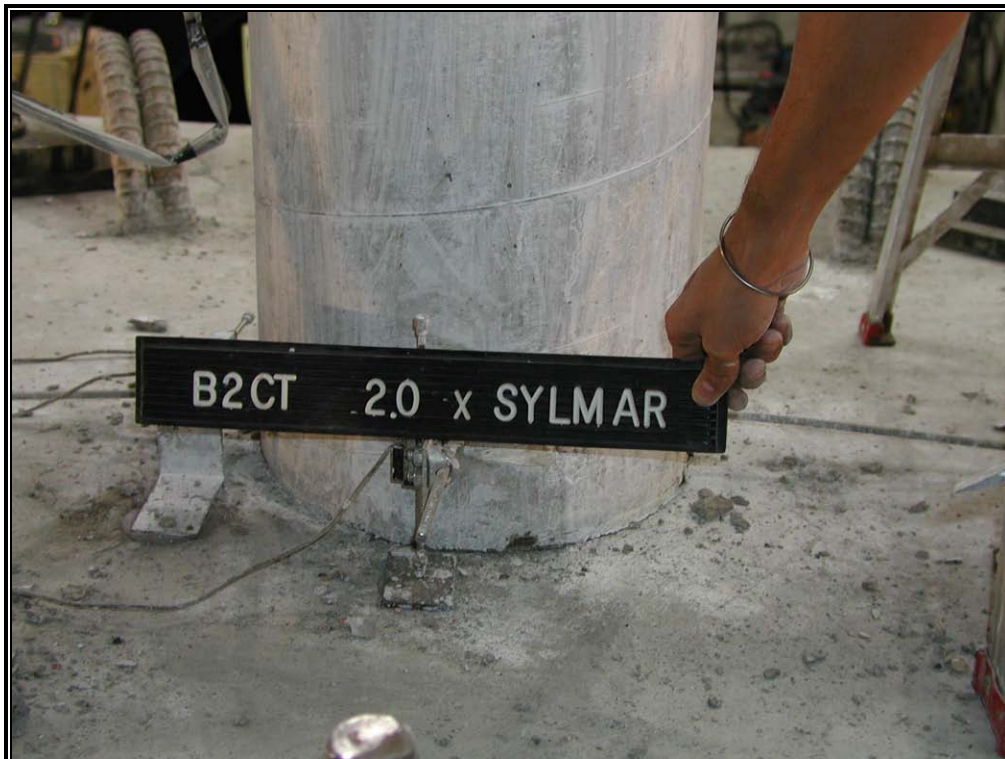
Fig. 4-49: West Side of East Column Base after 2.0 x Sylmar
