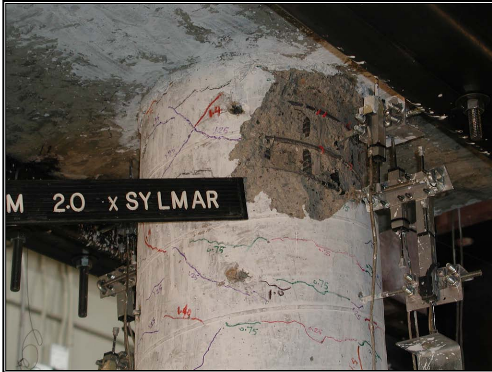
Fig. 4-30: Transverse and Long. Reinf. Exposure in West Column
