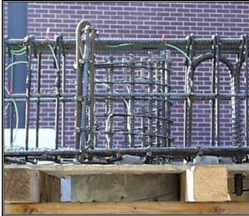
Fig. 6-1: Reinforcement Details of the Beam-Column Joint
