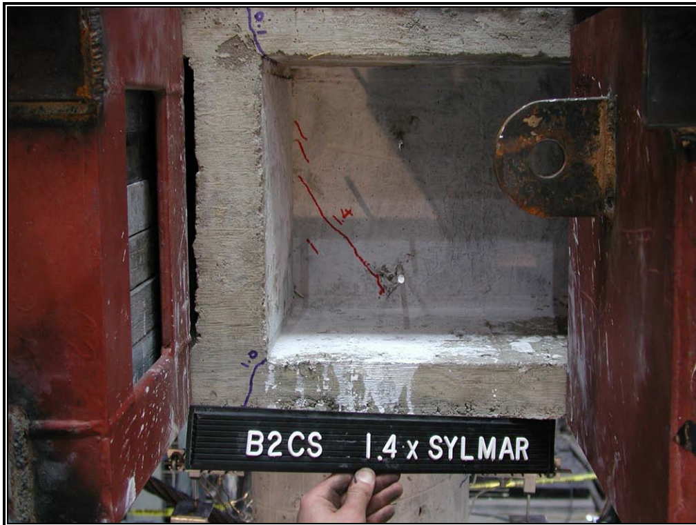
Fig. 4-7: Shear Cracks in East Beam-Column Joint
