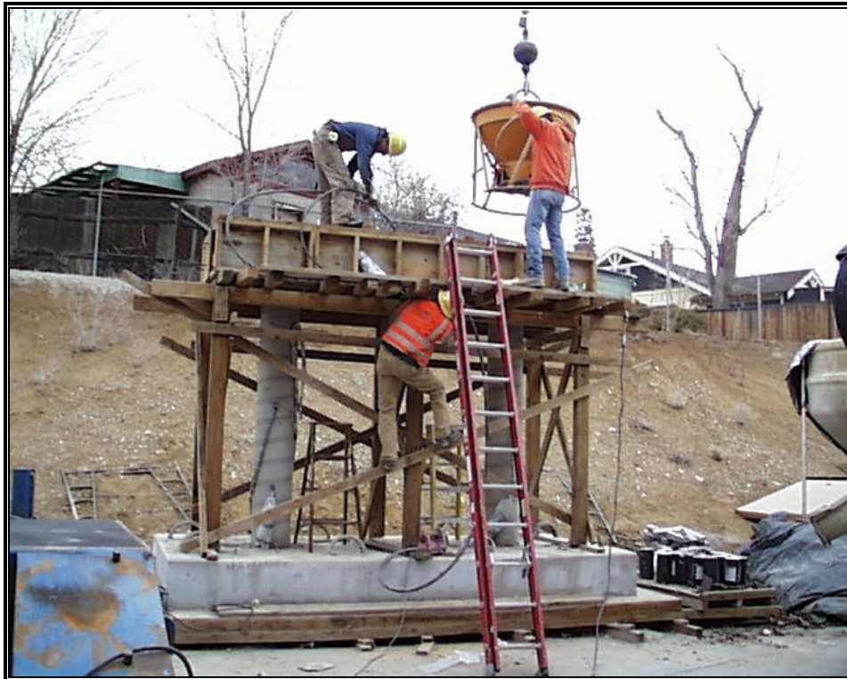
Fig. 3-24: Concrete Casting for Tall Specimen Beam
