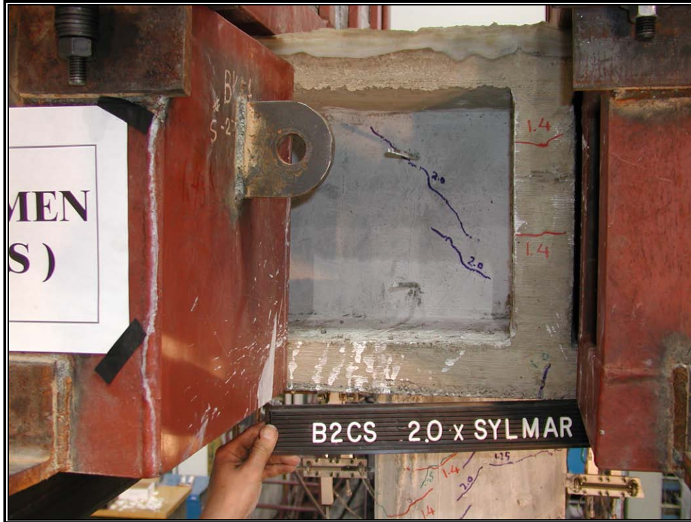
Fig. 4-8: Shear Cracks in West Beam-Column-Joint
