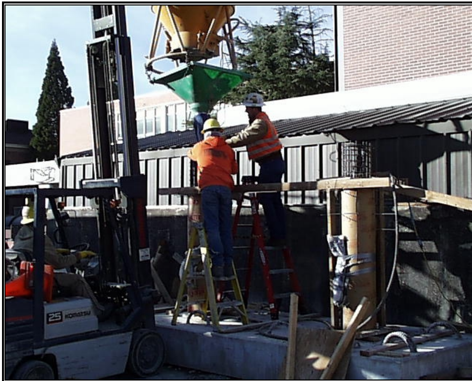
Fig. 3-16: Concrete Casting of Medium-Specimen Columns
