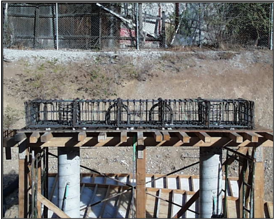
Fig. 3-20: Bent Cap Reinforcement
