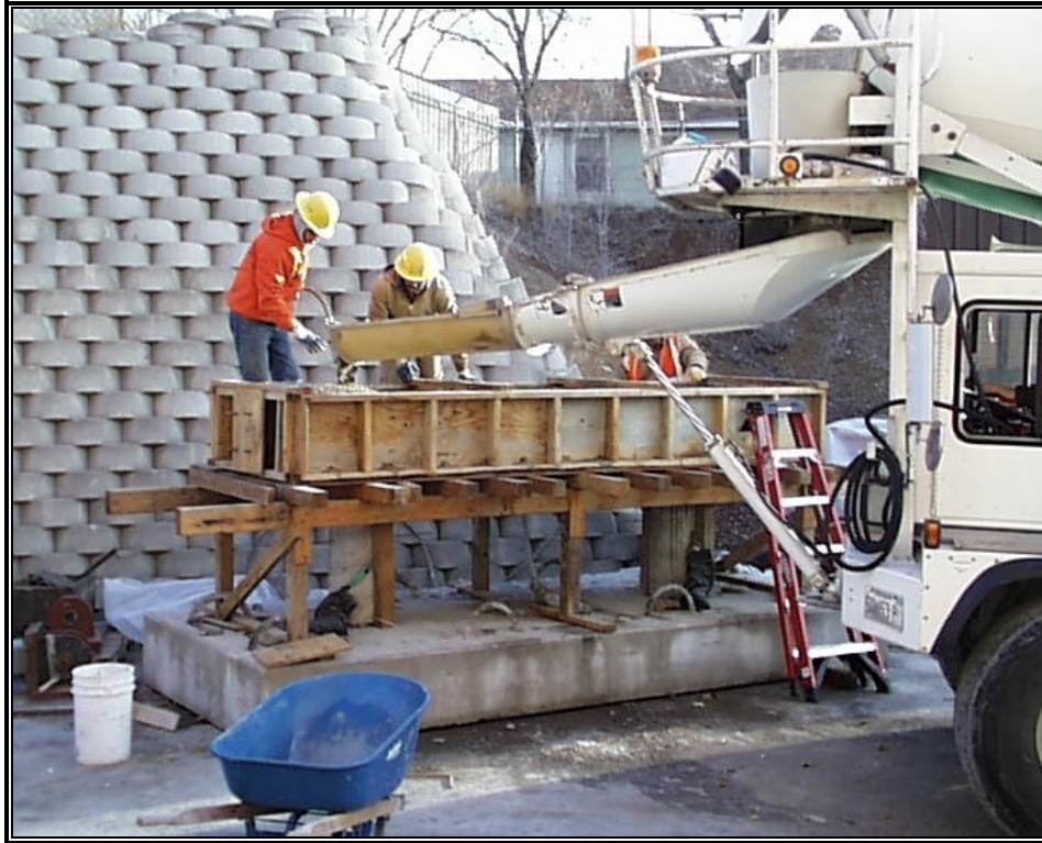
Fig. 3-22.a: Concrete Casting for Short Specimen Beam
