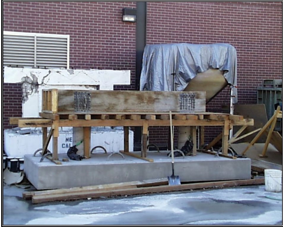
Fig. 3-19: Formwork of Bent Cap Beam
