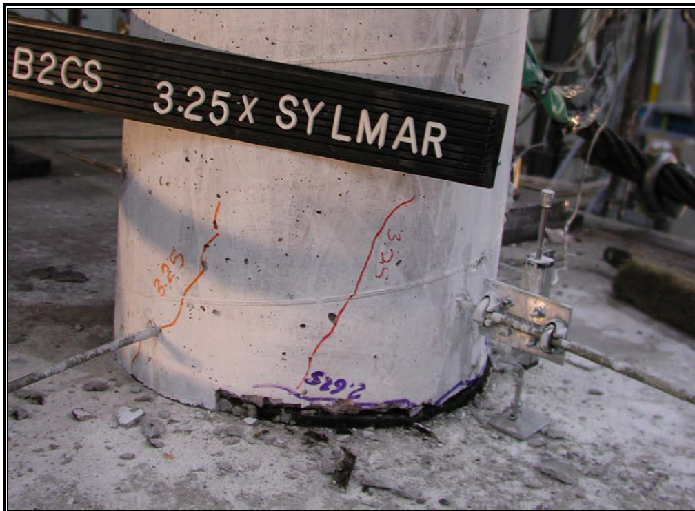
Fig. 4-13: Base Slippage in East Column
