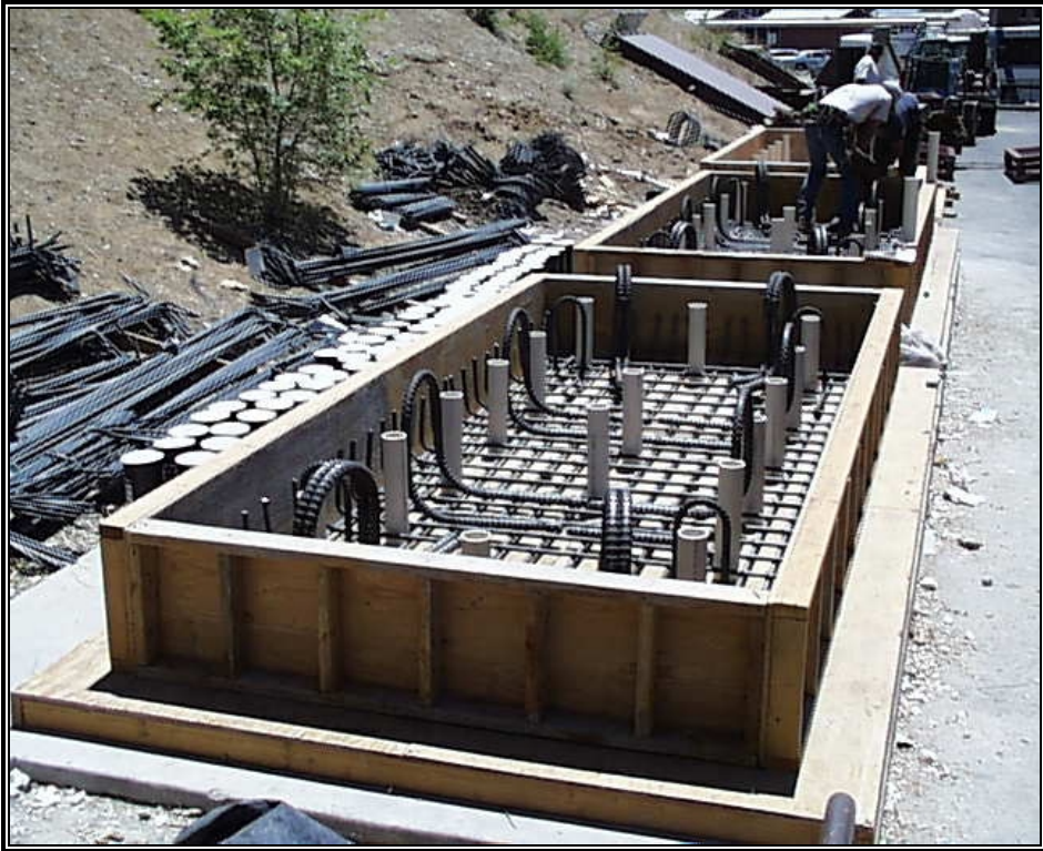
Fig. 3-2: Footing Bottom Reinforcement
