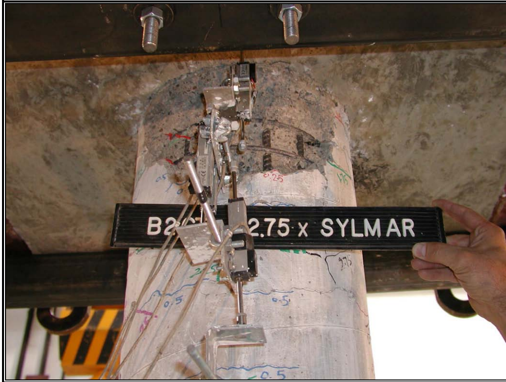
Fig. 4-58: Deep Concrete Spalling on West Side of East Column
