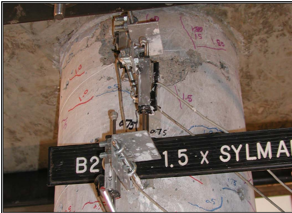
Fig. 4-47: Concrete Spalling on East Side of West Column
