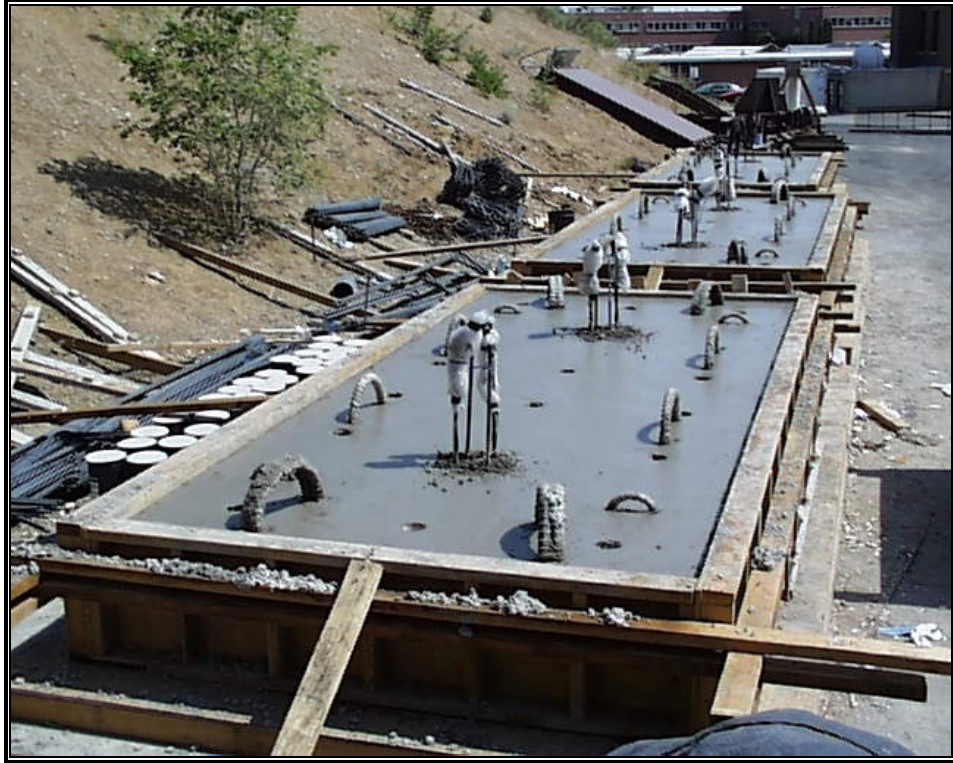
Fig. 3-5: Concrete casting of all Footings
