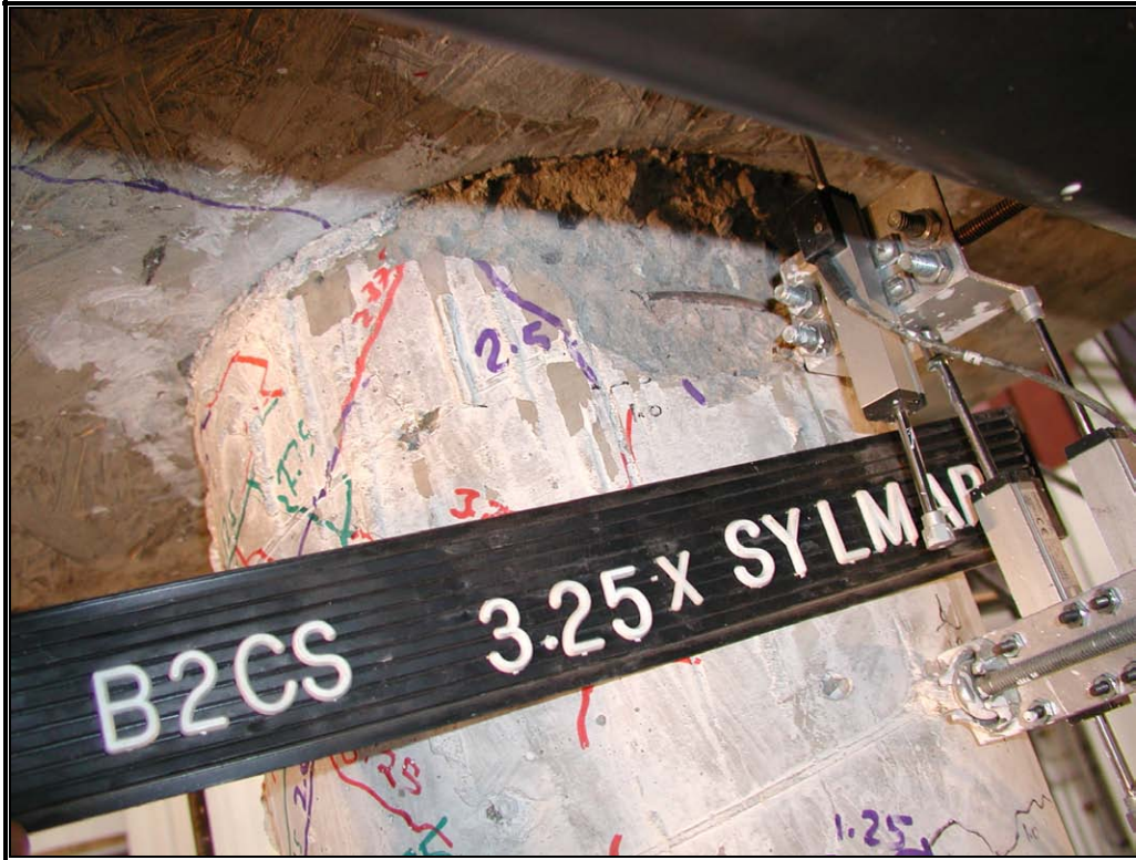
Fig. 4-16: Lateral Reinf. Exposure in East Column
