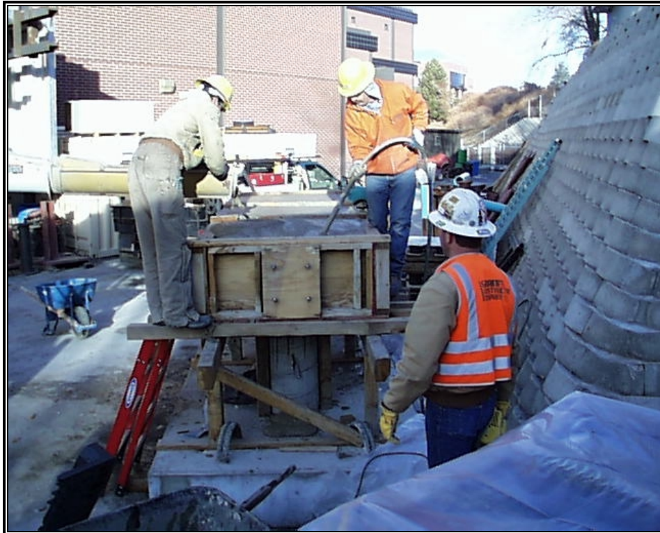
Fig. 3-22.b: Concrete Casting for Short Specimen Beam
