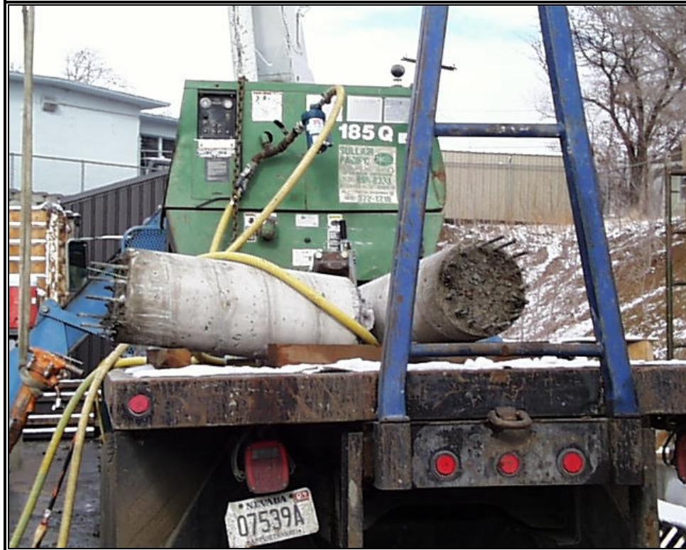
Fig. 3-18a: Removing of both Tall and Medium Columns
