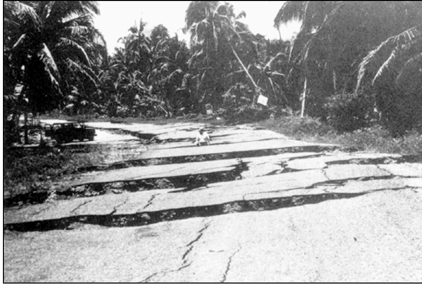
Figure 6-8. Extensional fissures in flexible pavement caused by lateral spread of floodplain deposits toward Rio Viscaya during the 1991 Costa Rica earthquake.
