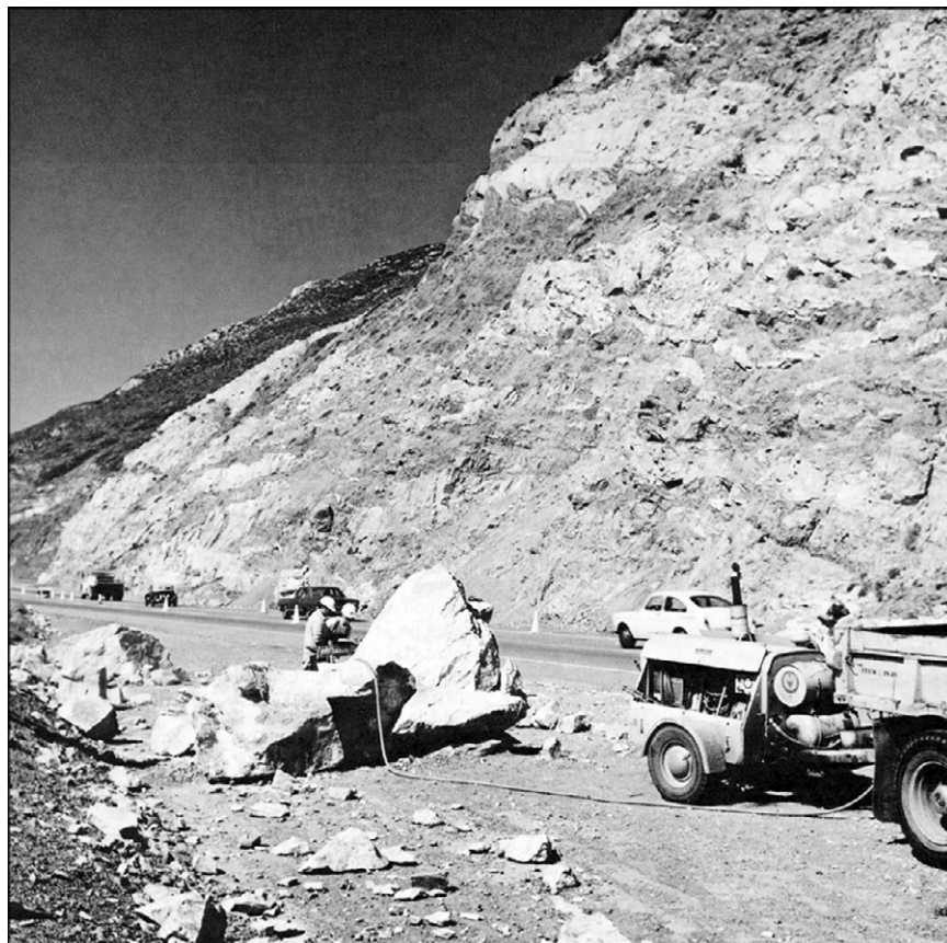
Figure 3-3. Rock falls along the Pacific Coast highway caused by the 1973 Point Mugu earthquake.
