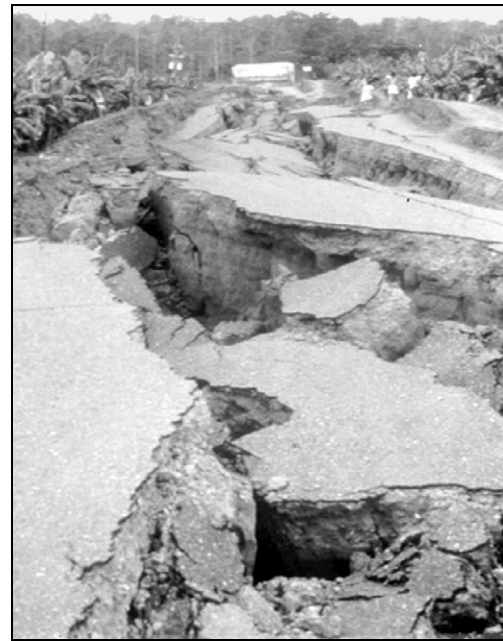
Figure 6-4. Failure mechanism beneath embankments that split, settle, and spread due to liquefaction of foundation soils.
