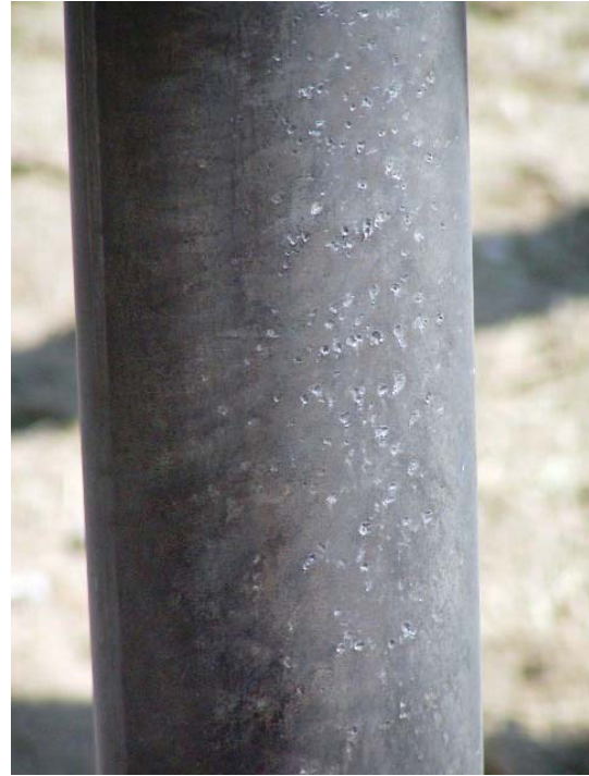
Figure 5-9 Column Surface of Column B1-C4 after Test 3
