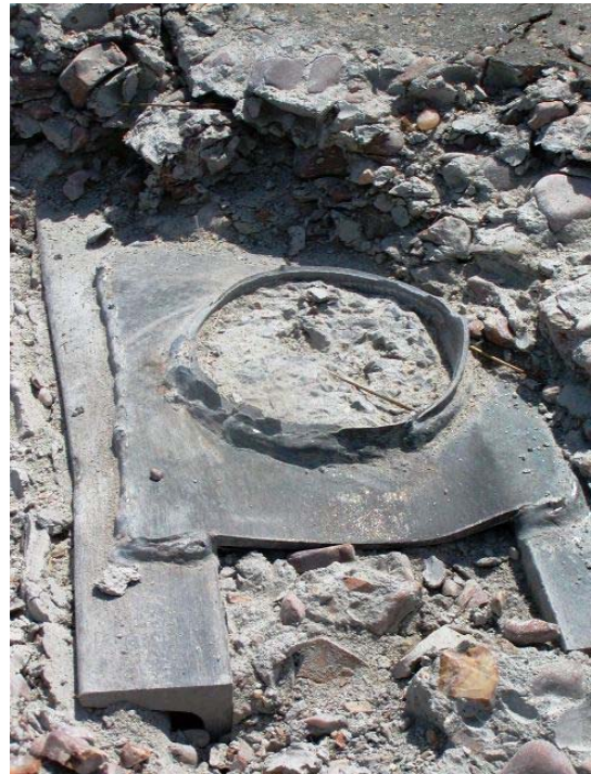
Figure 5-40 Foundation after Removal of Rubble (Column B2-C4, Test 7)
