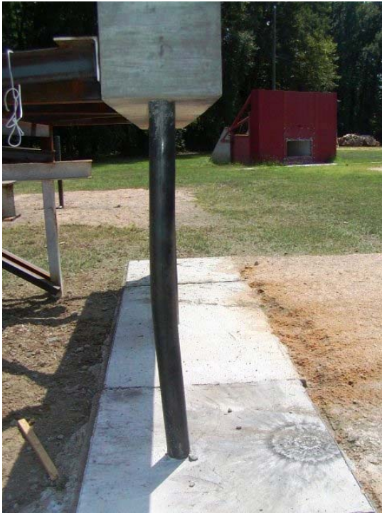
Figure 5-6 Column B1-C4 after Test 3
