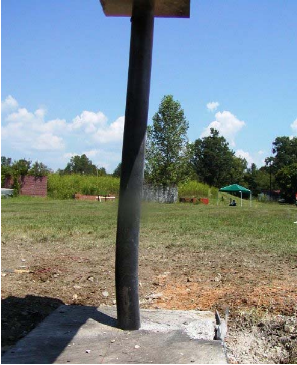
Figure 5-27 Column B2-C4 after Test 6
