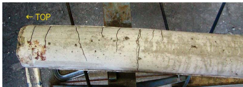
Figure 5-58 Core Concrete of Column B2-C6 after Test 9
