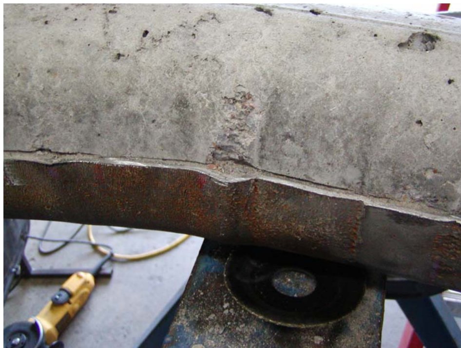
Figure 5-68 Core Concrete at Steel Buckling of Column B2-C5 after Test 10
