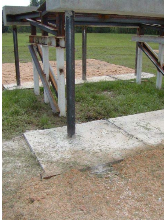
Figure 5-2 Column B1-C4 after Test 1
