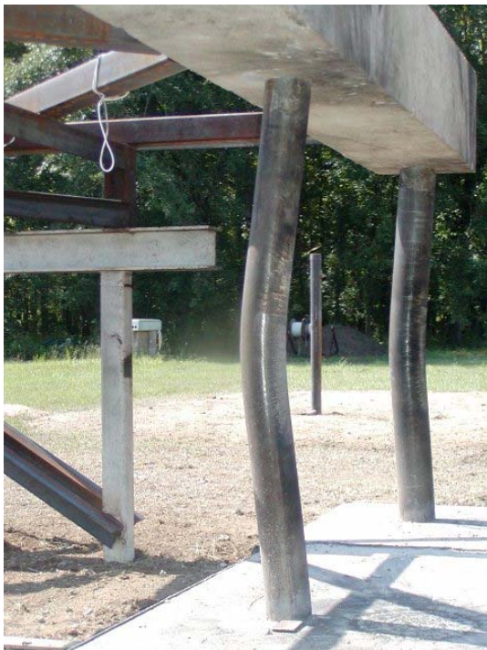
Figure 5-19 Column B1-C5 after Test 5
