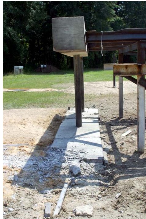
Figure 5-33 Disappearance of Column B2-C4 after Test 7
