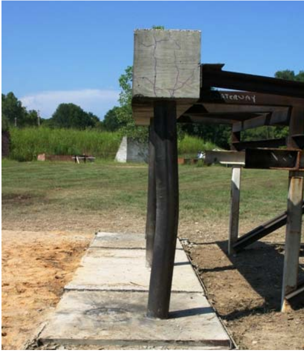
Figure 5-11 Column B1-C6 after Test 4
