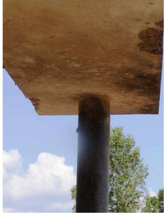
Figure 5-31 No Damage at Cap-beam of Column B2-C4 after Test 6
