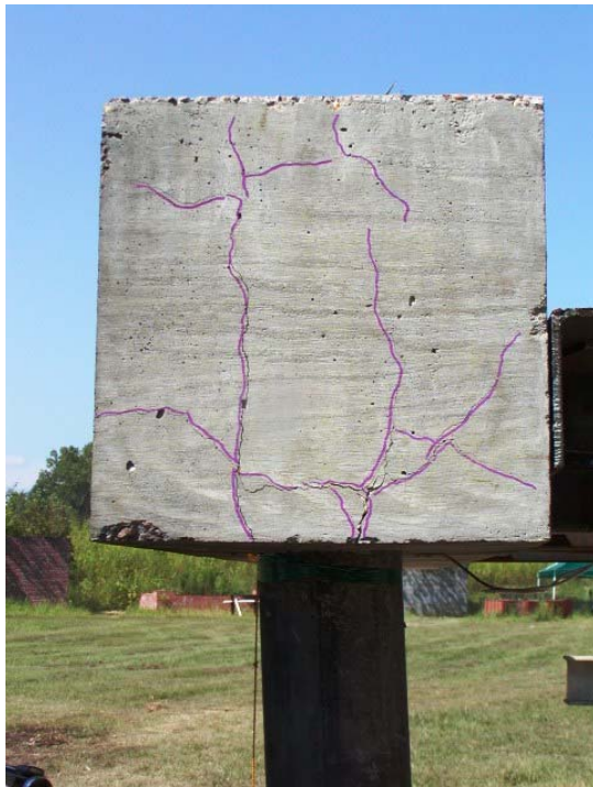
Figure 5-16 Cracking at Cap-beam of Column B1-C6 after Test 4
