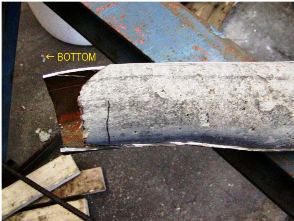
Figure 5-46 Bottom of Column B2-C4 after Test 7
