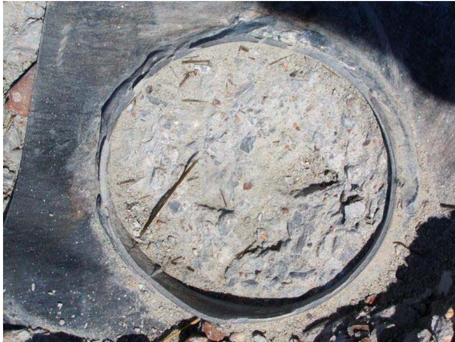
Figure 5-41 Fracture Surface of Column in Foundation (Column B2-C4, Test 7)
