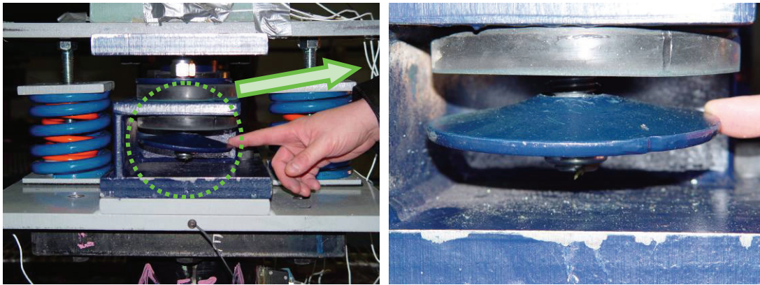
Figure 6-12 Damage in Vertical Restraint Component of 1.0 g Design I/R Systems at the End of Seismic Test TS2-S8a
