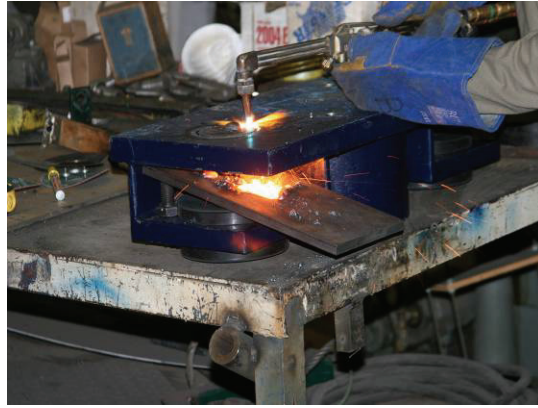
(b) Torching Holes in Base Plate
