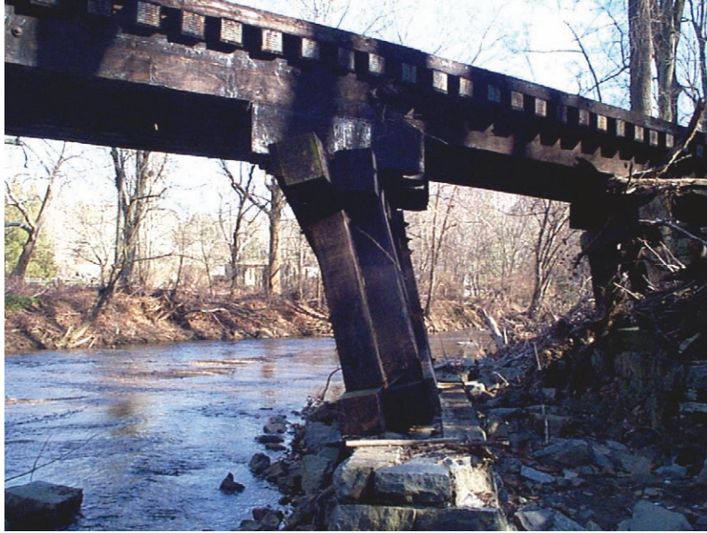
Figure 1-2. Timber pile bent that experienced damage in an out-of-plane failure mode.
