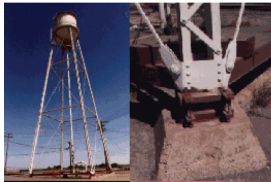
b. An application of FP bearing with uplift restrainer in an elevated water tank ( http://www.earthquakeprotection.com )
