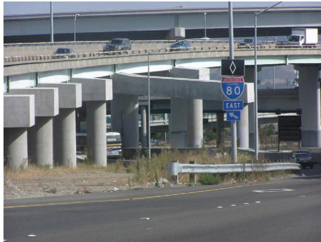
FIGURE 2-1 Reinforced Concrete Moment-Resisting Frame Construction
