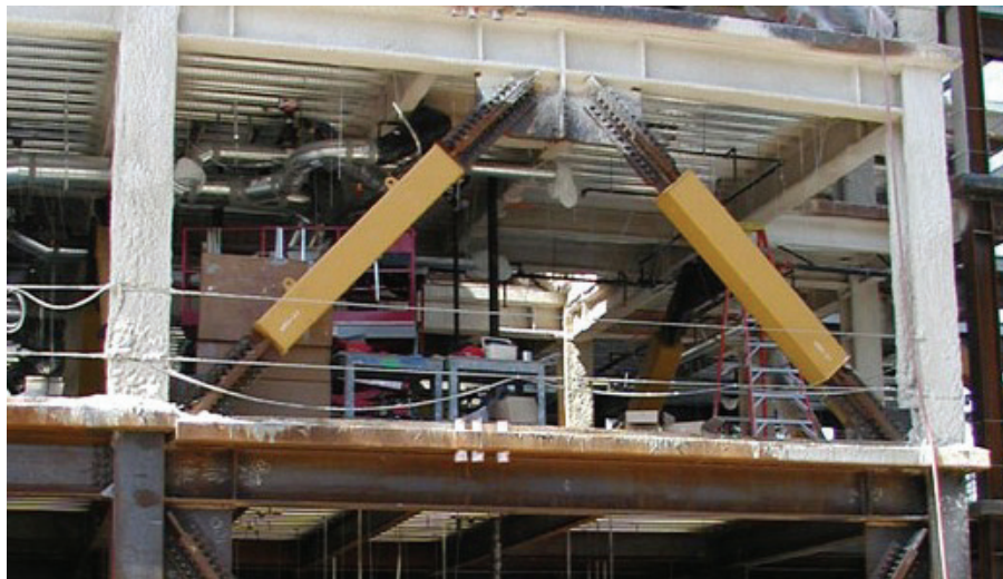
FIGURE 11-2 Chevron Brace Installation of Buckling Restrained Braces
