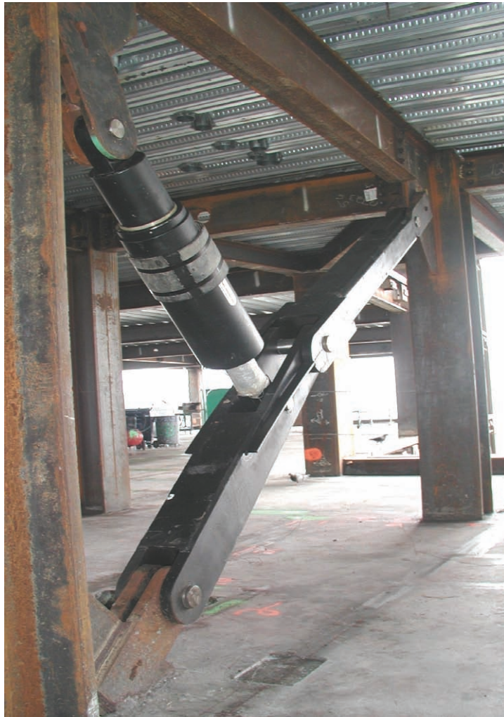
FIGURE 11-6 Reverse-toggle Brace Installation
