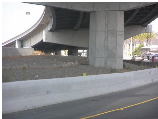
FIGURE 2-2 Reinforced Concrete Pier-Bent Cap Construction
