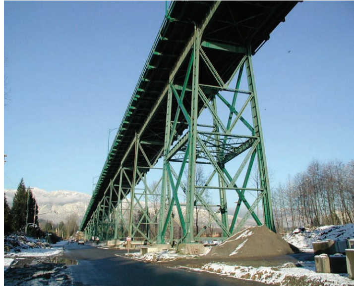
FIGURE 11-1 Braced Steel Piers
