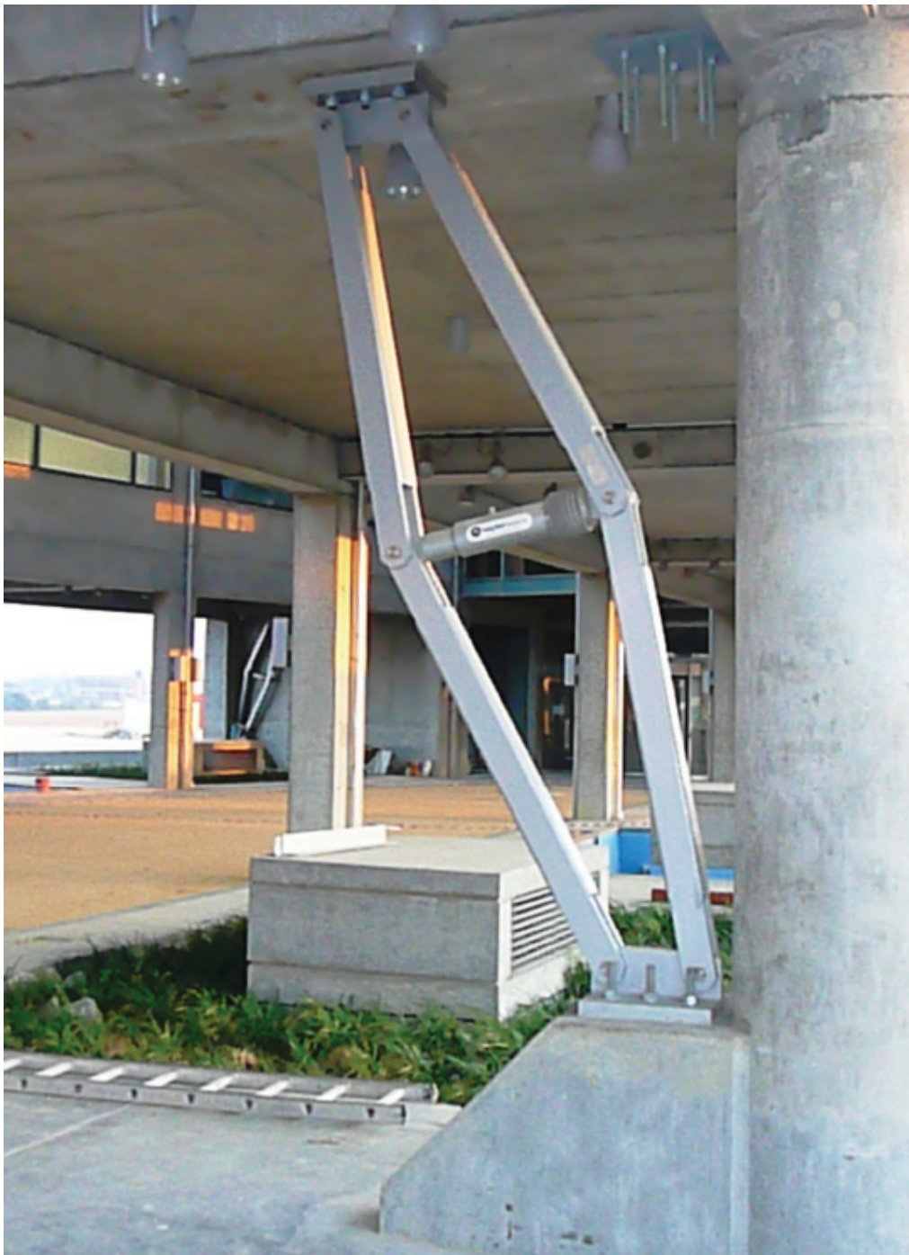
FIGURE 11-7 Scissor-jack Assembly Installation
