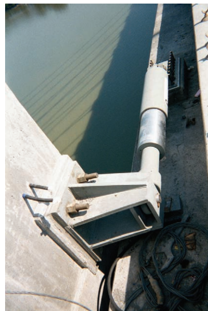
b. damper installation
