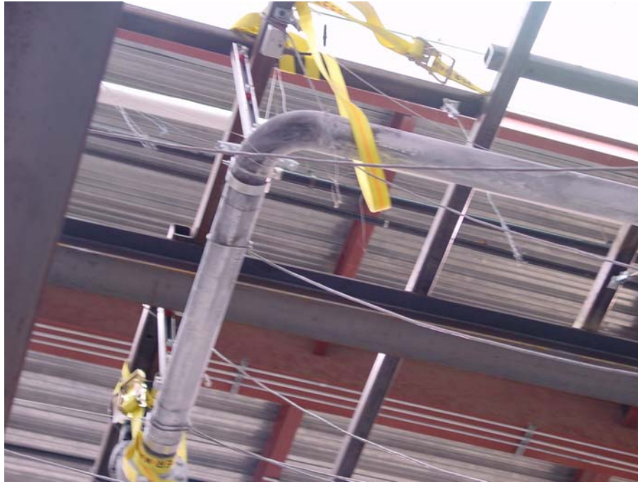
Figure 3-13 Failure of Brace B6
