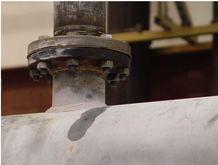
Figure 3-43 Initial Leak On Heat Exchanger Connection
