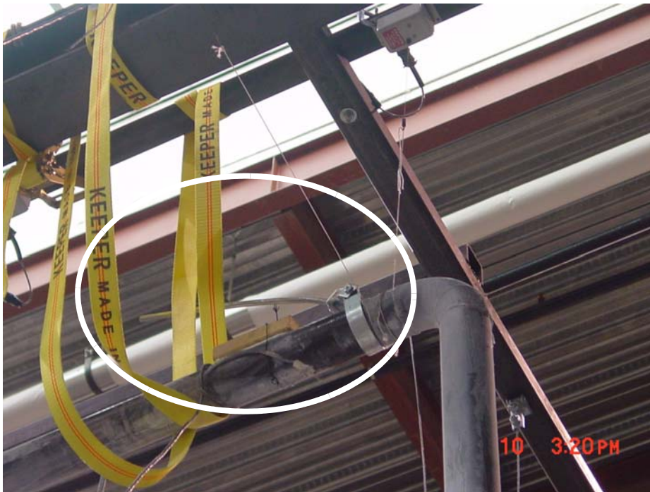
Figure 3-29 Failure of Hanger B1
