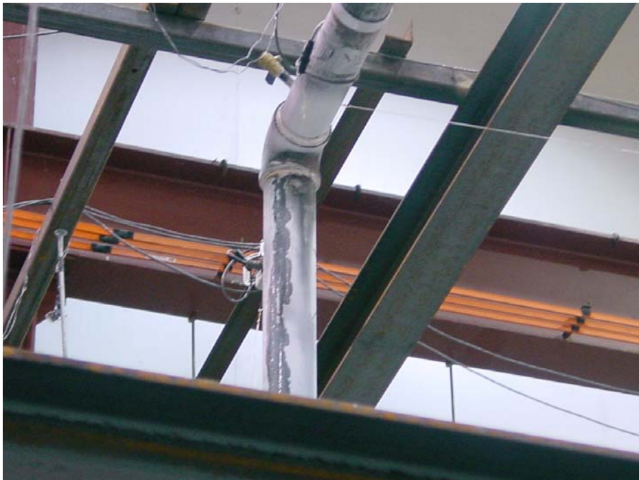
Figure 3-62 Elbow Above Heat Exchanger Leakage
