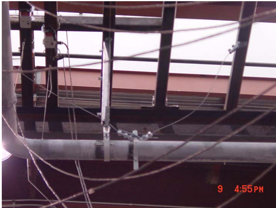
Figure 3-15 Permanent Offset of Brace B5
