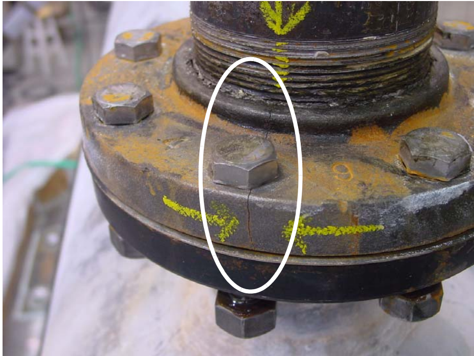
Figure 3-46 Fracture of the Flange
