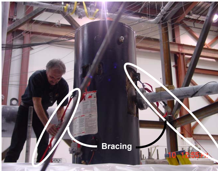
Figure 2-17 Bracing Water Heater to Table
