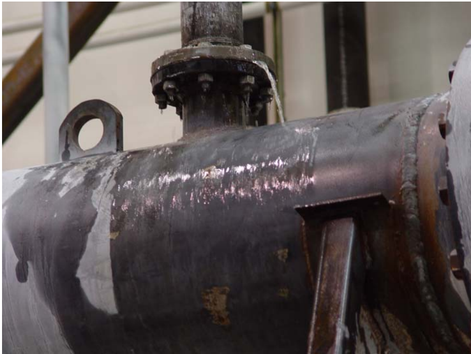
Figure 3-45 Water Flowing Out of Heat Exchanger Connection
