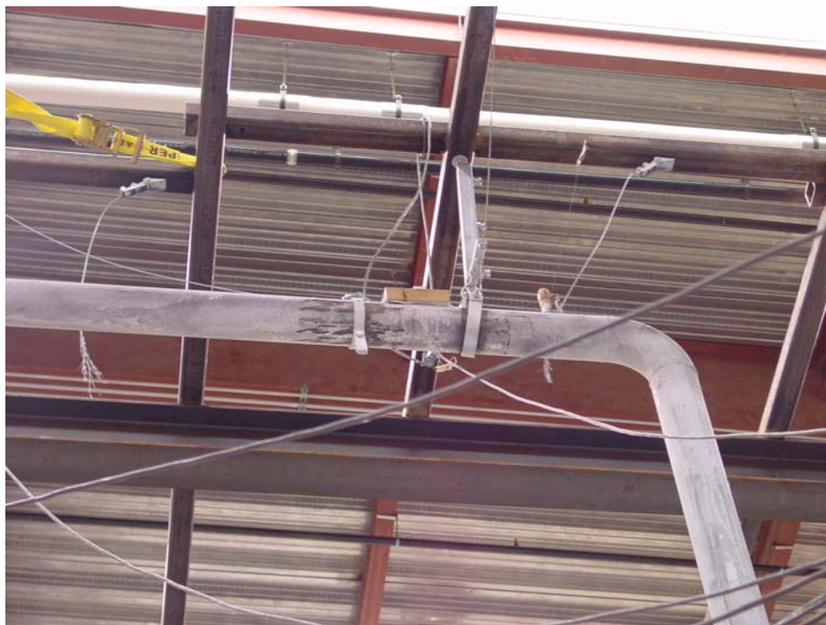
Figure 3-14 Failure of Longitudinal Portion of Brace B7
