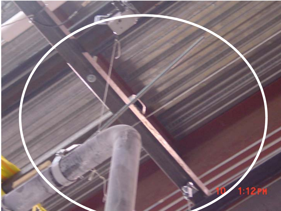
Figure 3-28 Failure of Hanger B2
