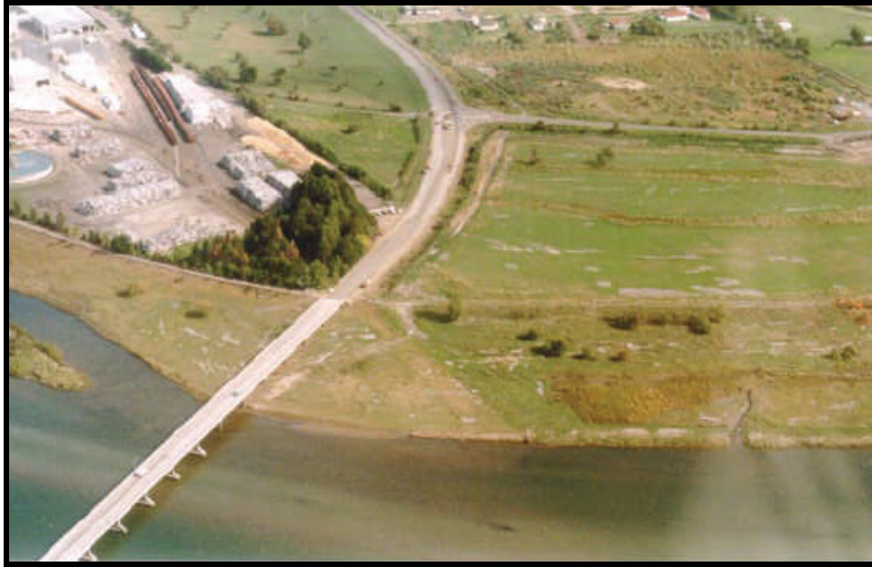
Figure 1.9: The Landing Road Bridge, after the 1987 Edgecumbe earthquake, New Zealand (Berrill et al., 2002)
