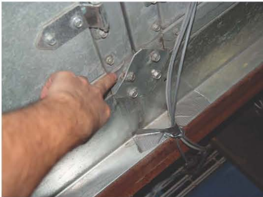
(a) Damaged Connection Plate between Base Rail and Test Specimen Housing
