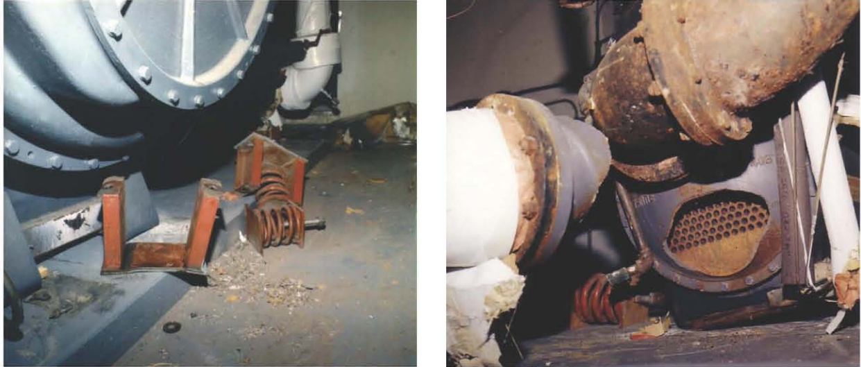
Figure 3-2 Pipe Rupture Resulting from Vibration-Isolator Supports Failure during Northridge Earthquake (Lloyd, 2003)
