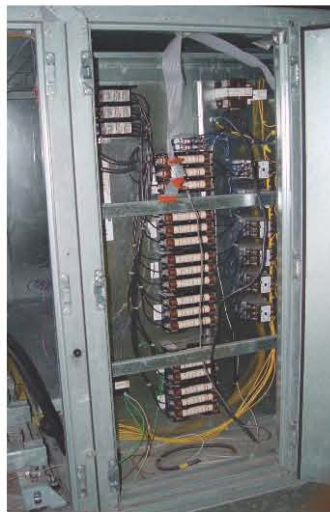
(c) Electric Heat Coil Module
