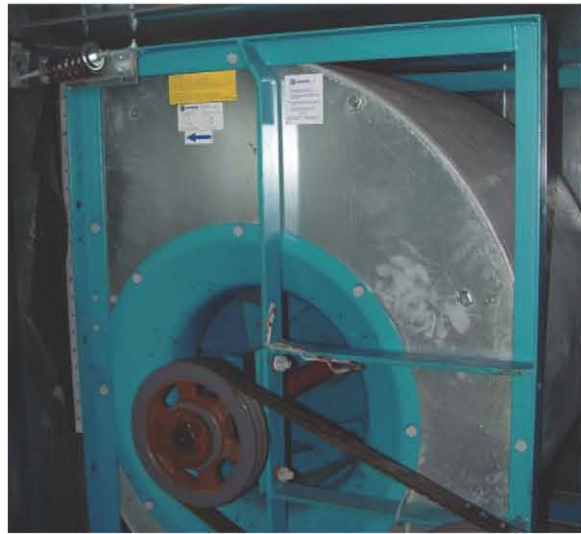
(b) Unrestrained Vibration Isolator between Fan Case and AHU Housing (Circled with Dotted Line)
