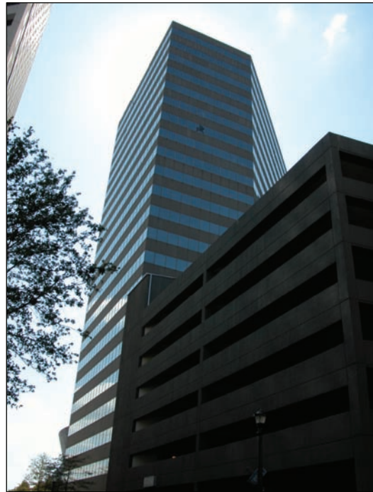
(b) North Facade
