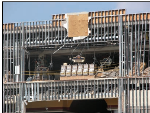
(b) Damage to Barge
