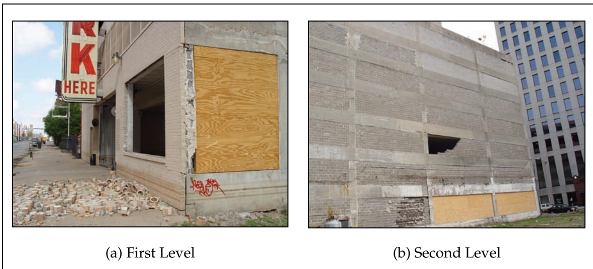
Figure 4-4. Masonry infill damage.
