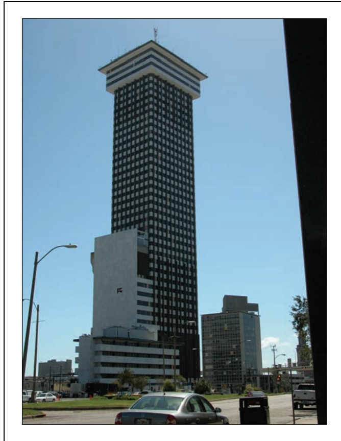
Figure 3-10. Office building in the New Orleans Business District at a distance from other high-rise structures.
