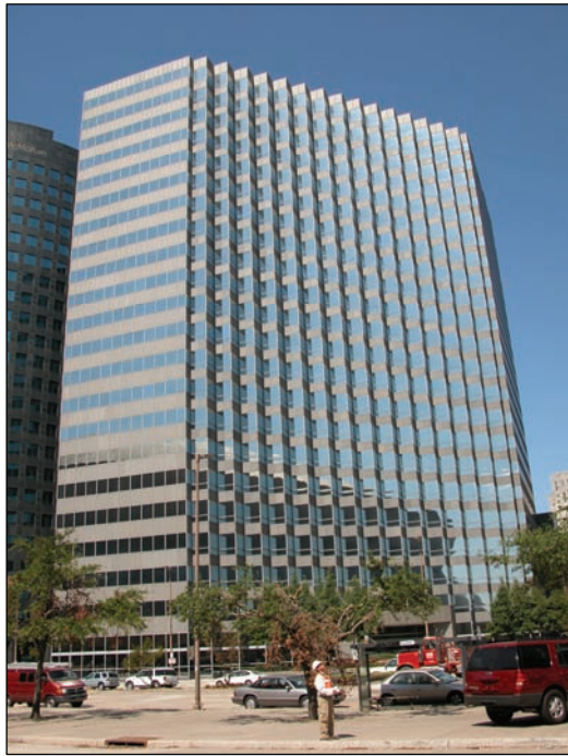
(a) South Facade
