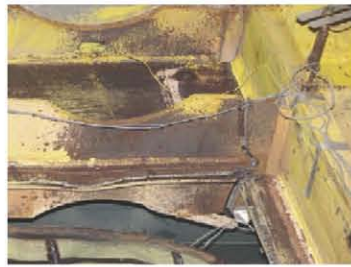
Figure 4. Ruptures at the north end of intermediate beam
