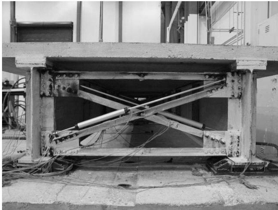
FIGURE 2-11 “Heavy” end cross frames at the north end in the bridge model
