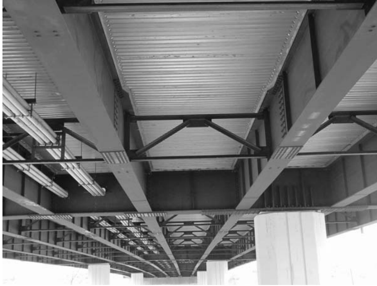
FIGURE 1-1 Typical K-brace cross frame
