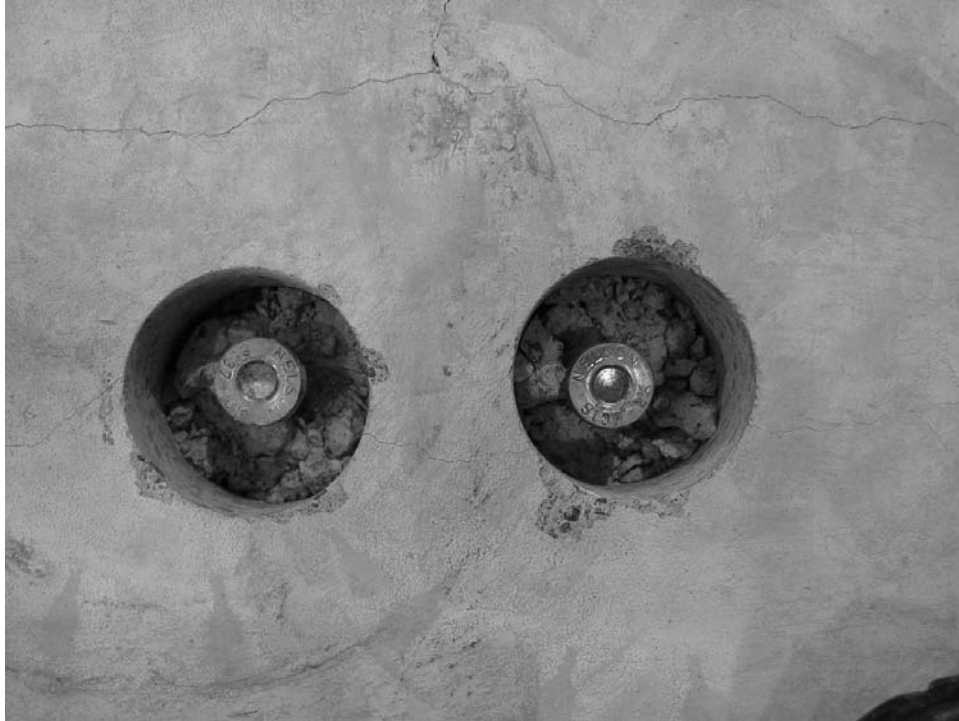
FIGURE 3-29 Effect of shear studs removed by through the deck slab around the studs
