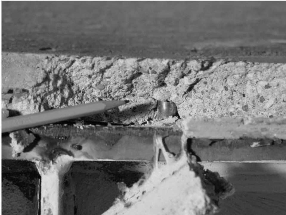
FIGURE 3-4 RSHXB - Failure of shear stud at north end of bridge model
