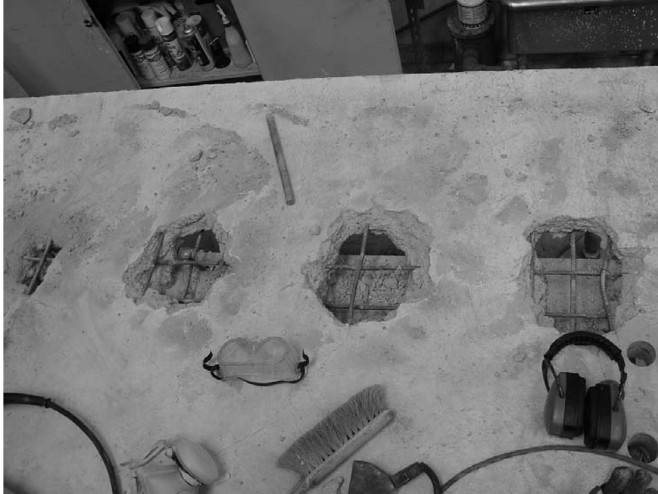
FIGURE 3-5 Removal of concrete for rehabilitation of shear studs at north end of bridge model
