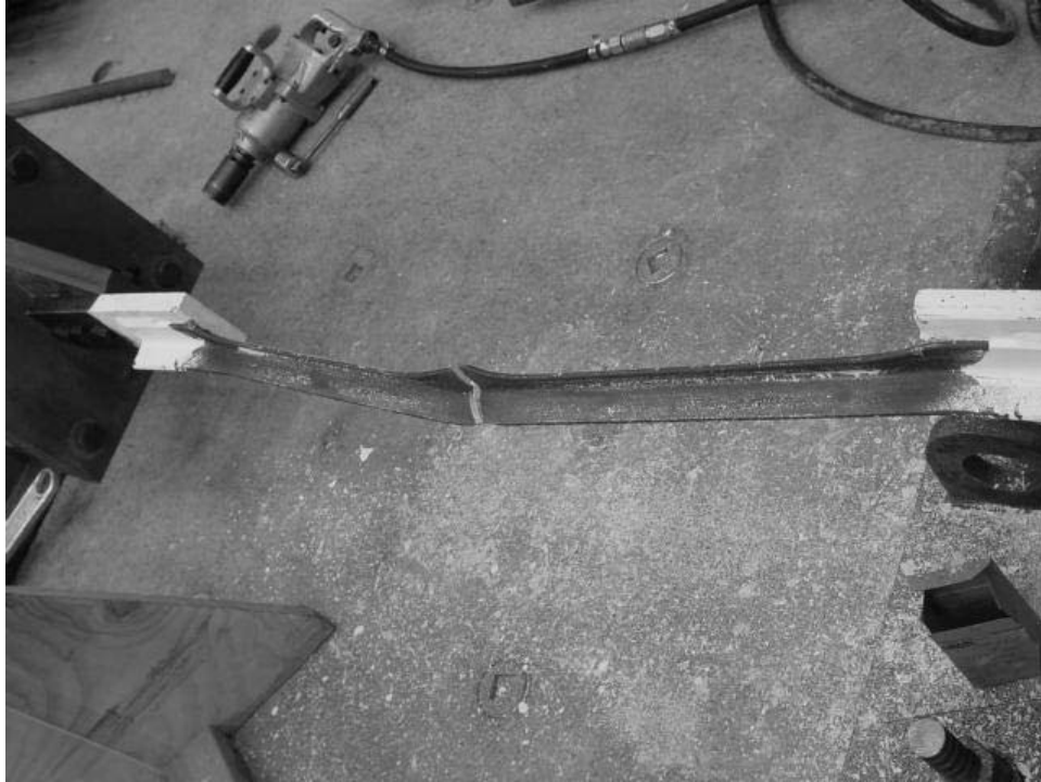
FIGURE 3-8 Failure of single angle with welded connection
