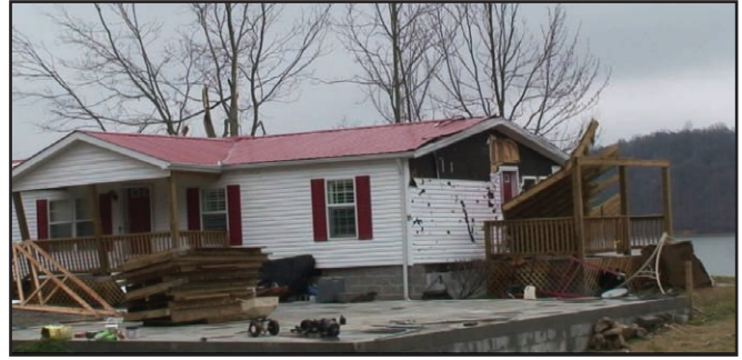
Figure 15. An example of damage consistent with EF-0 rating near McKinnon, TN (Houston County). From Table 7, loss of awnings and siding is expected for DOD 2, with an expected wind speed of 79 mph. The image was taken looking west with Tennessee River in the background.
