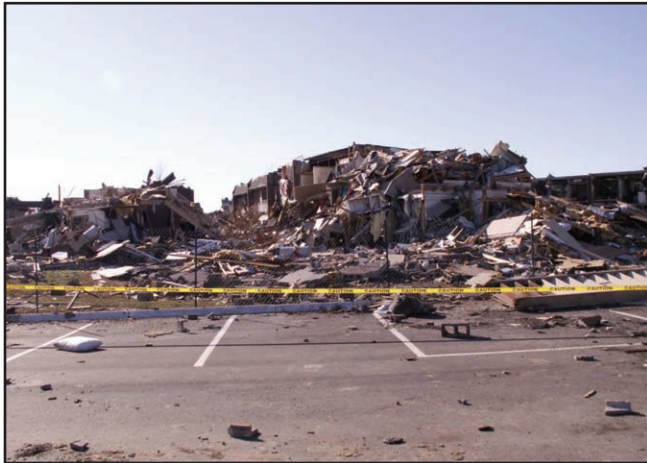
Figure 23. Worst damage to residence halls on Union University campus. Taken at approximately the center of campus looking west.
