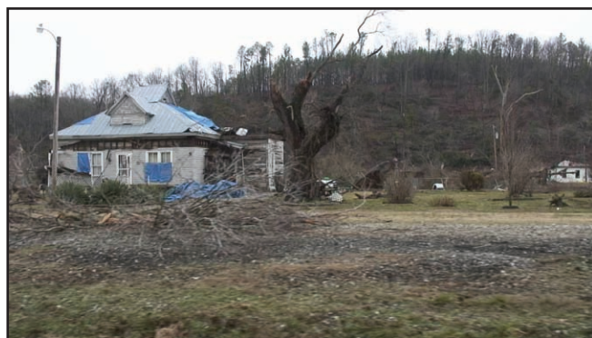
Figure 13. Older construction with damage to roof covering and windows. An overhanging porch has also been removed (Faxton, TN, Benton County).
