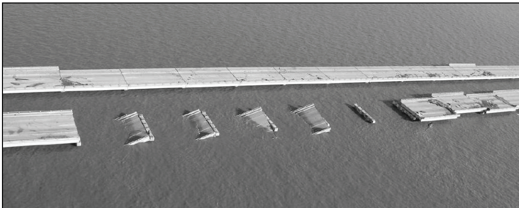
Figure 6-1. Dislodged Spans of I-10 Twin Spans, Lake Pontchartrain, Louisiana, Hurricane Katrina
