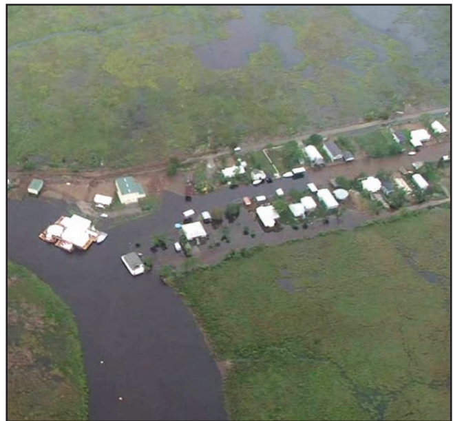
Figure 7. Lacombe, LA - example of flooded urban area.
