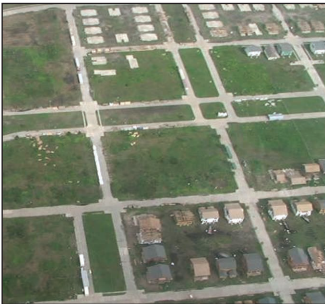
Figure 6. New Orleans 9th Ward - Minor wind-induced damage.
