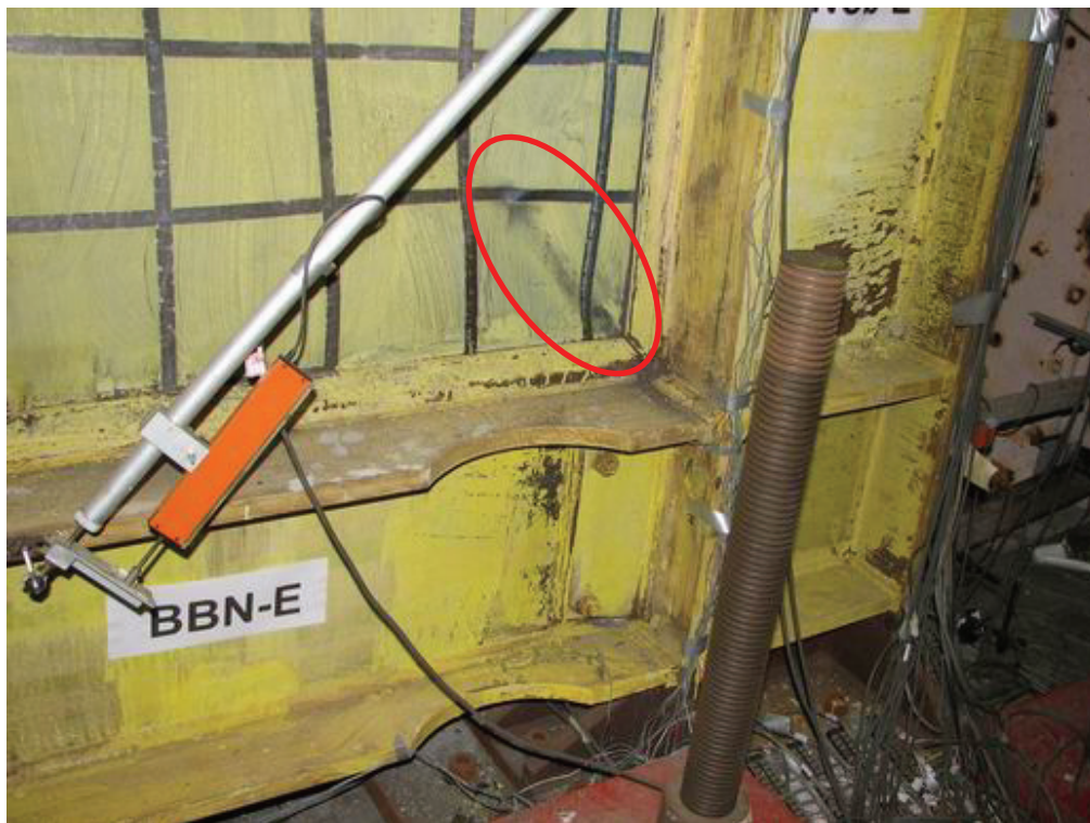
(a) Lower North Corner of The First-Story Panel
