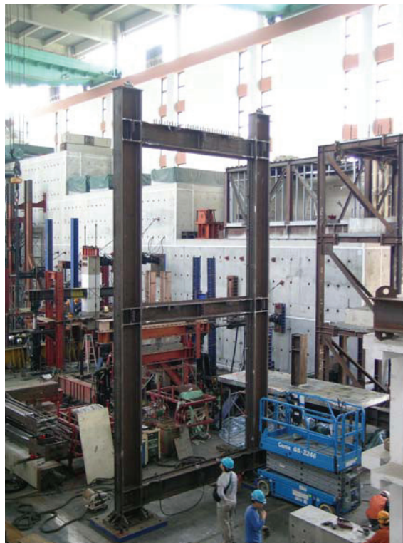
FIGURE 3-8 Installation of HBEs (Photo Courtesy of C.H.Lin and K.C.Tsai, NCREE)
