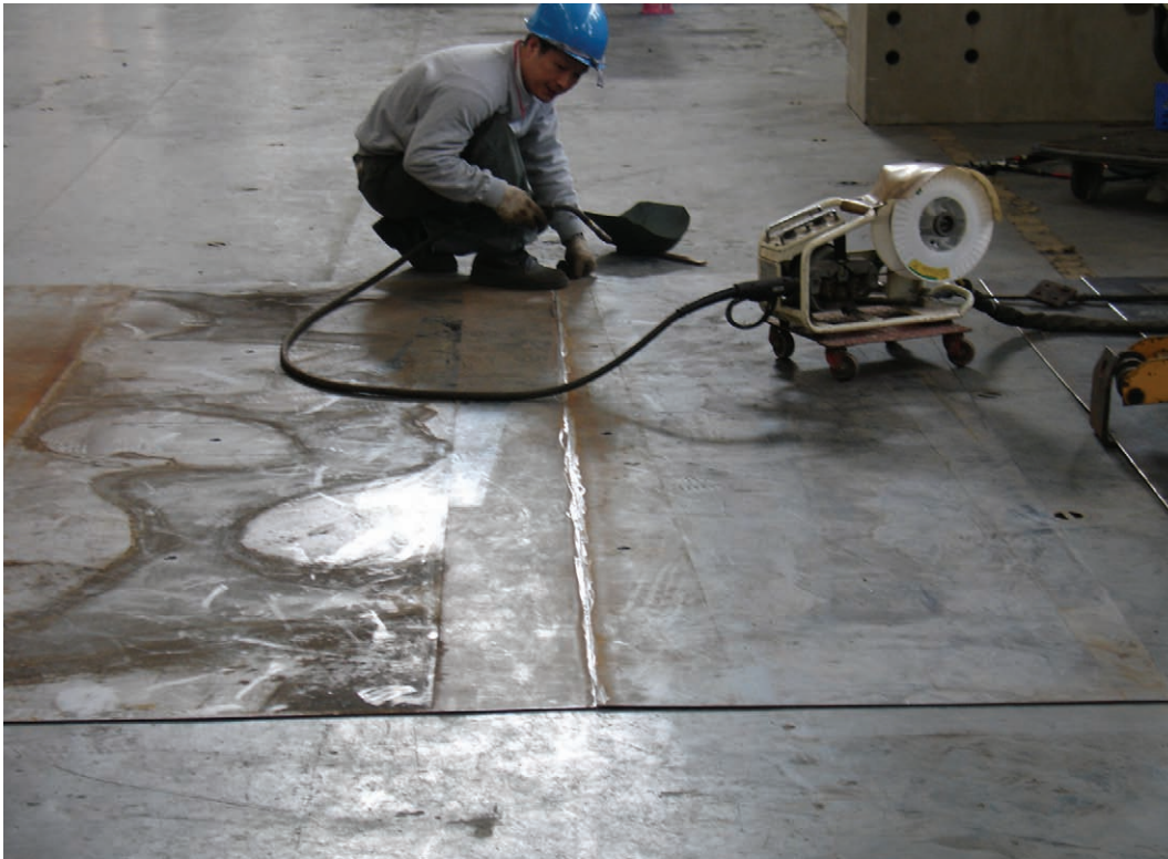
FIGURE 3-9 Manual Welds along Small Plate Segment Edges (Photo Courtesy of C.H.Lin and K.C.Tsai, NCREE)
