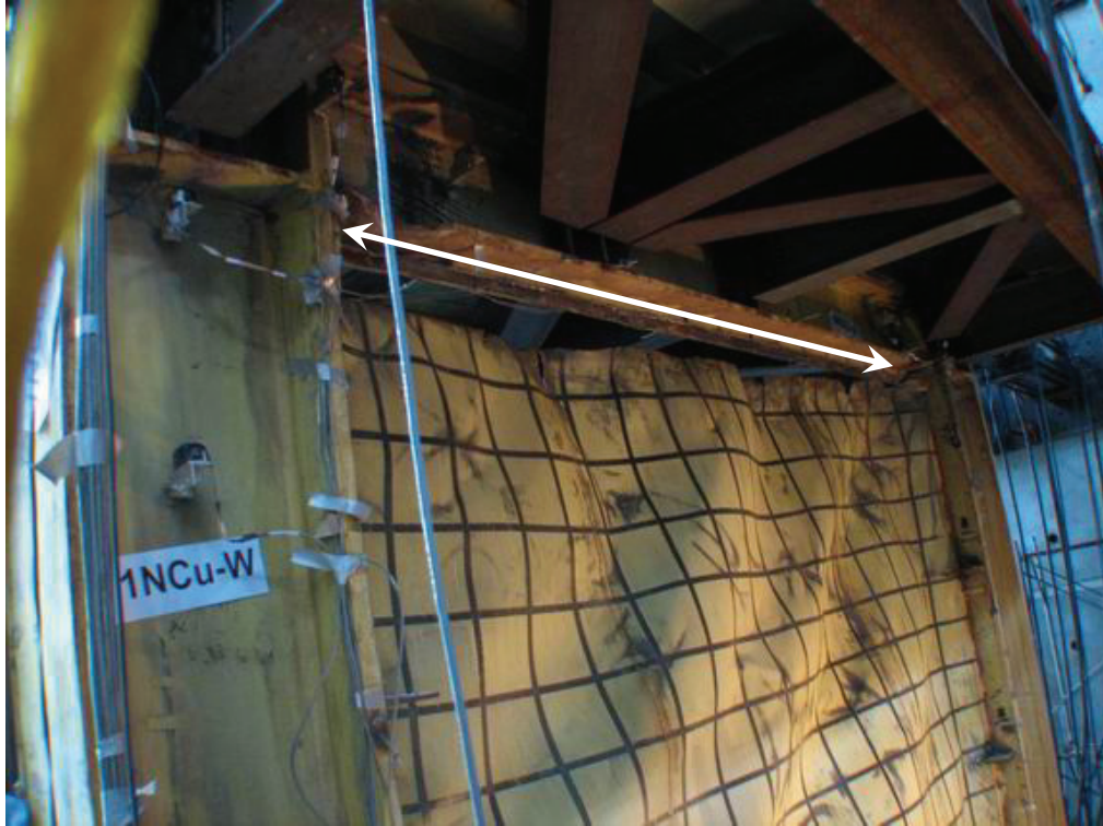
FIGURE 4-57 Plate Tear at the Upper North Corner of the First-Story Infill Panel (During Cycle 14)
