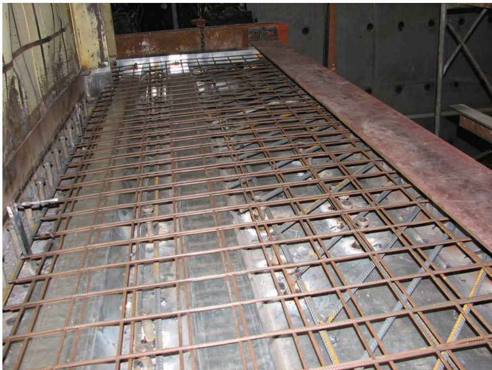
(b) Rebar Layout of the Intermediate Slab
