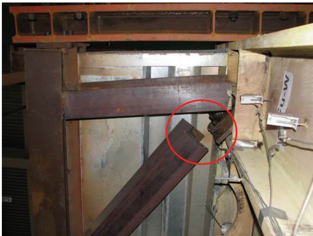
(b) Fractures of the Truss Member Connected to the End of the Top HBE
