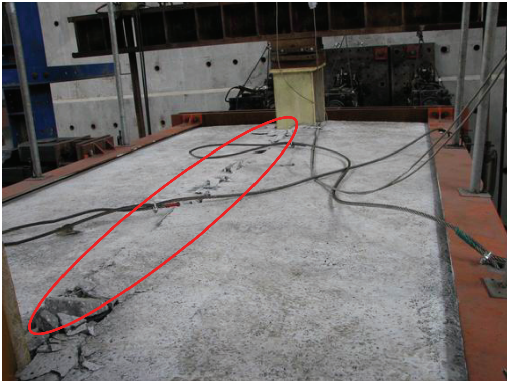
FIGURE 4-60 Crack in the Top Concrete Slab
