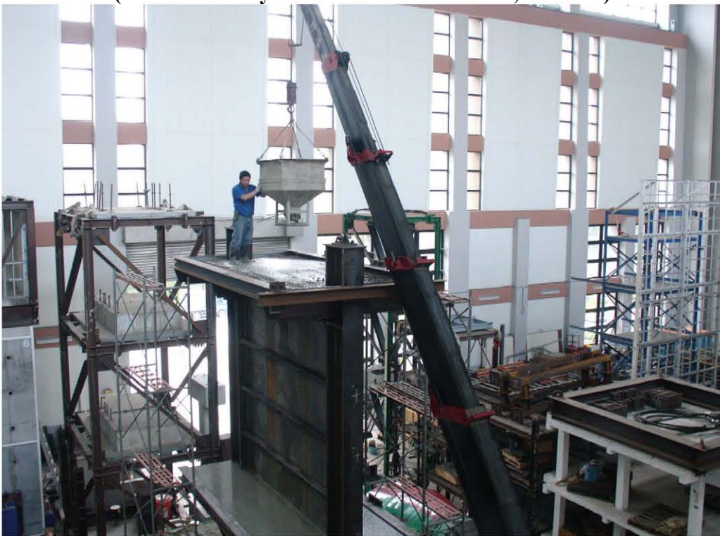
FIGURE 3-14 Casting Concrete Slab (Photo Courtesy of C.H.Lin and K.C.Tsai, NCREE)
