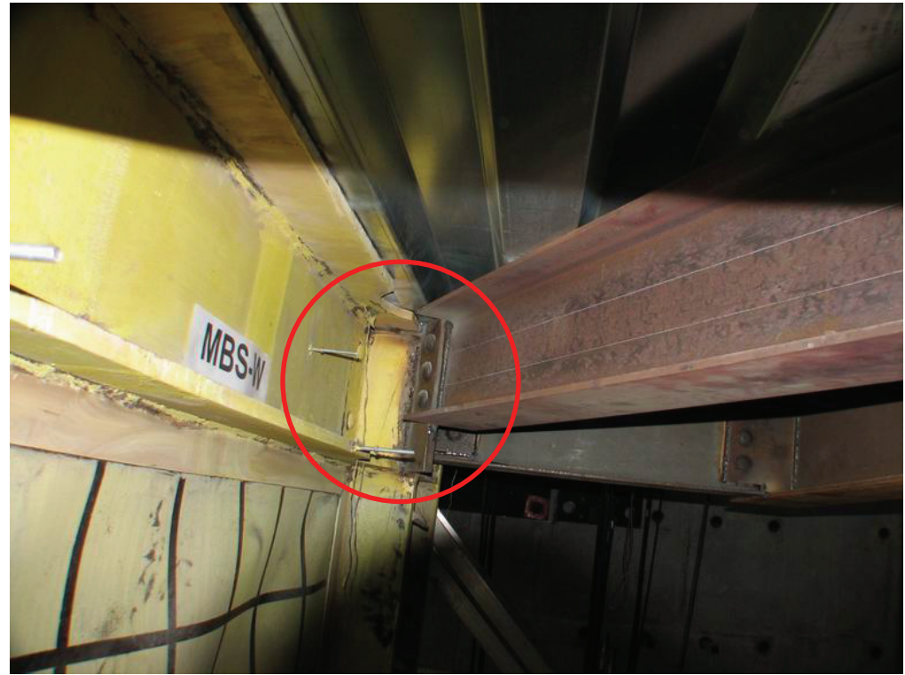
FIGURE 4-12 Typical Floor-Truss-Member-to-Intermediate-HBE Connection
