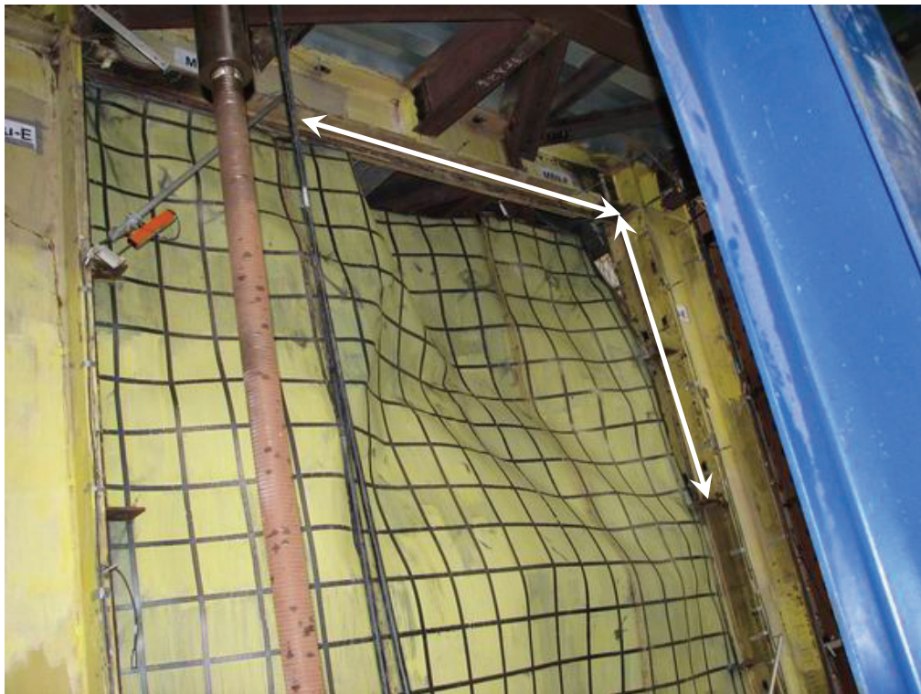
FIGURE 4-56 Plate Tear at the Upper North Corner of the First-Story Infill Panel (During Cycle 13)
