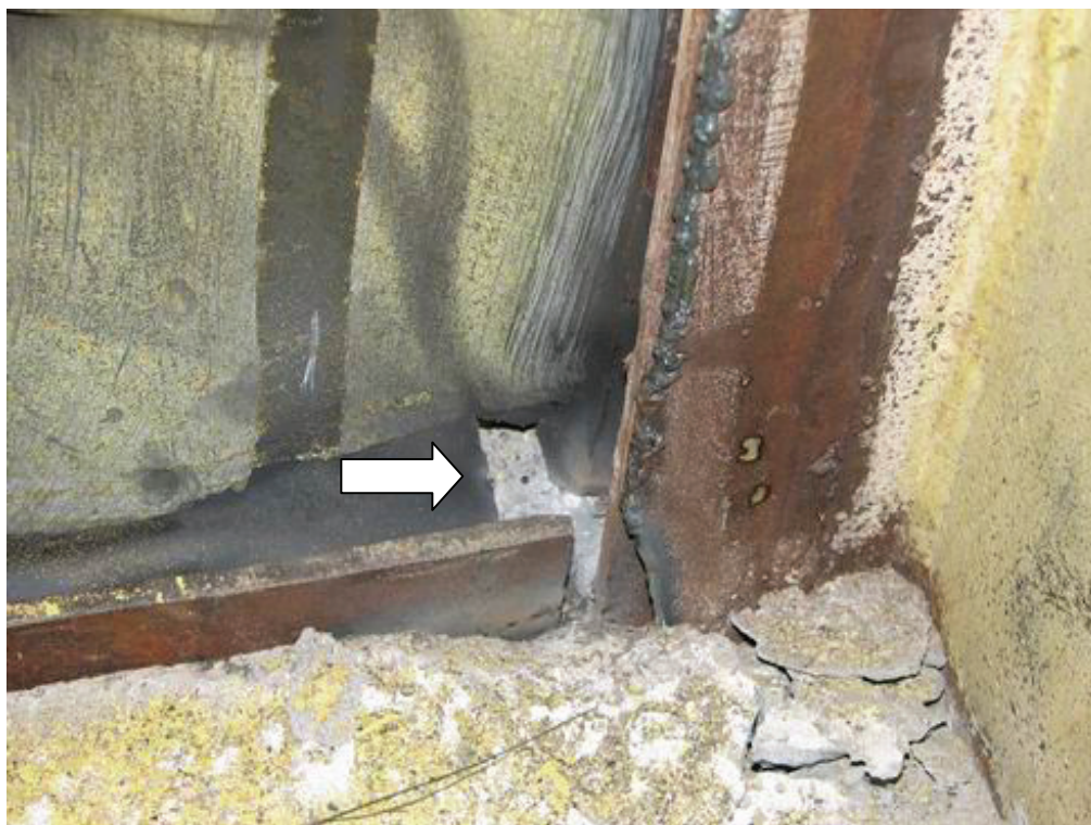
(b) Development of the Panel Tear
