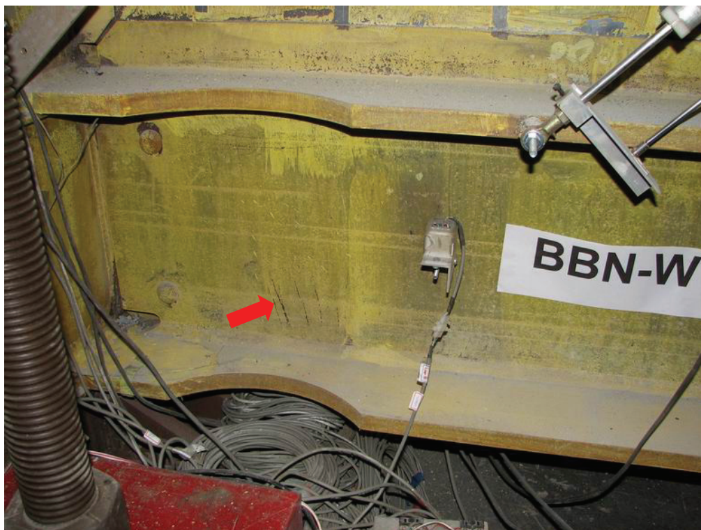
(b) North End of the Bottom HBE – West Side
