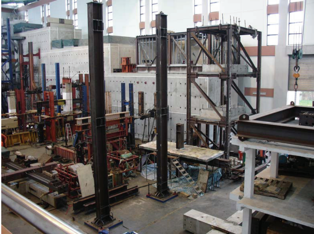
FIGURE 3-7 VBE Erection (Photo Courtesy of C.H.Lin and K.C.Tsai, NCREE)
