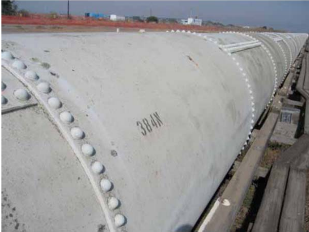
Figure 5.9 Riveted Steel Pipeline (after American Lifelines Alliance, 2005)
