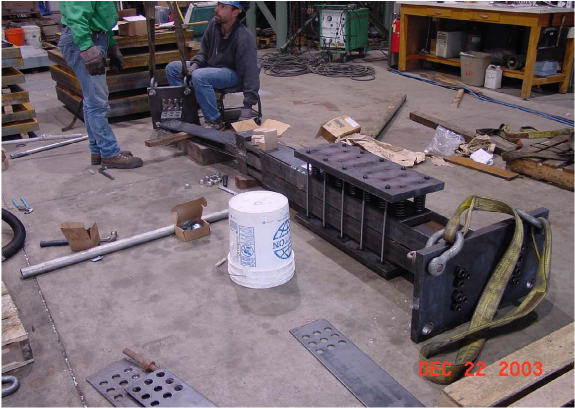
Figure 2-3 Assembling friction damper
