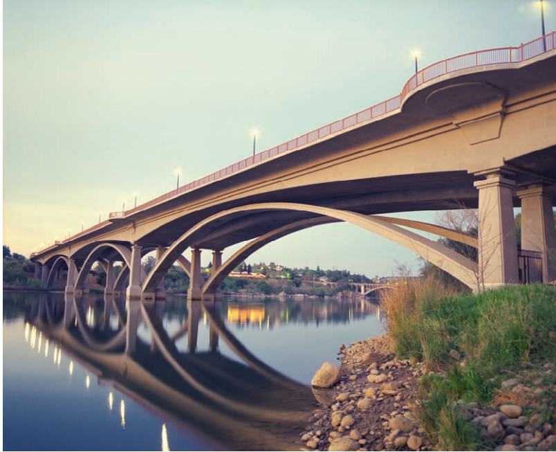
Figure 1-5 The American River Bridge, City of Folsom, California (courtesy of Earthquake Protection Systems)
