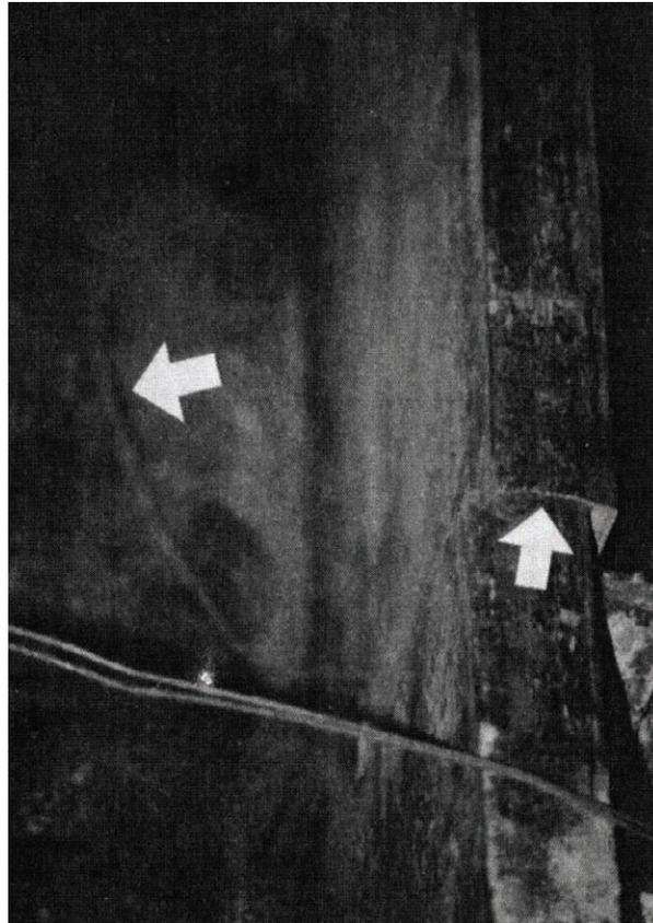
Figure 1-3 Typical Connection Damage in the Northridge Earthquake (Bruneau et al. 1998)
