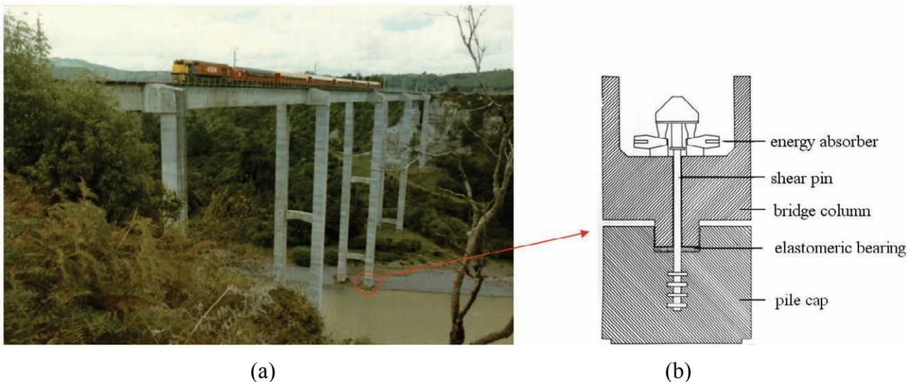
Figure 2-1 Rangitikei Railway Bridge (a) Overall View (b) Rocking Pad (Cormack 1988)
