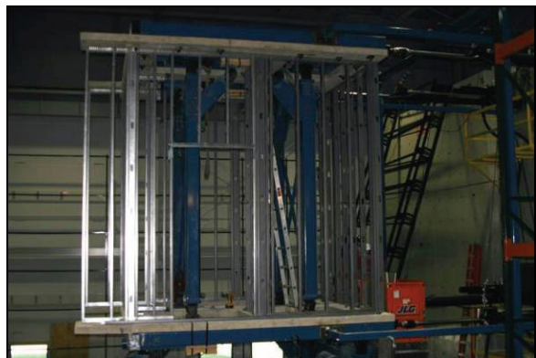
Figure 5.15. General view of steel stud framing
