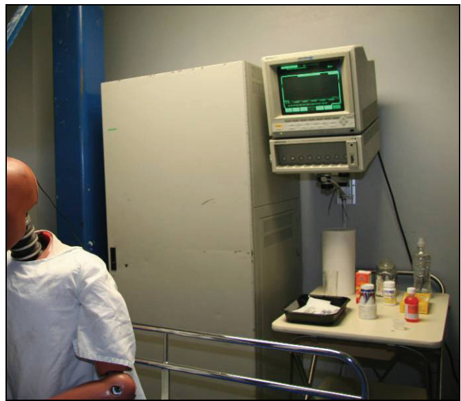
Figure 5.43. General view of exterior of video equipment rack
