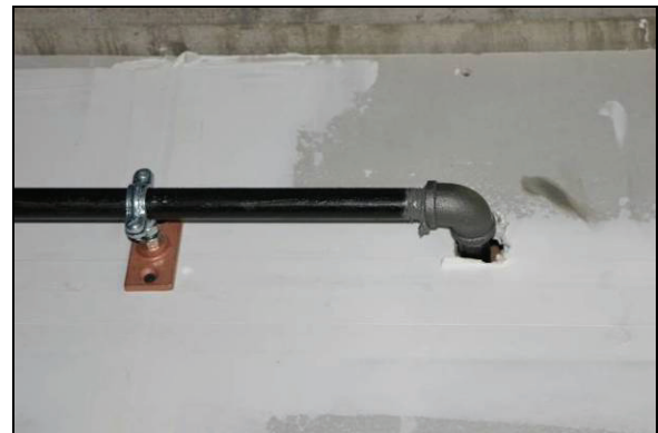
Figure 5.26. Detail of sprinkler run crossing partition wall
