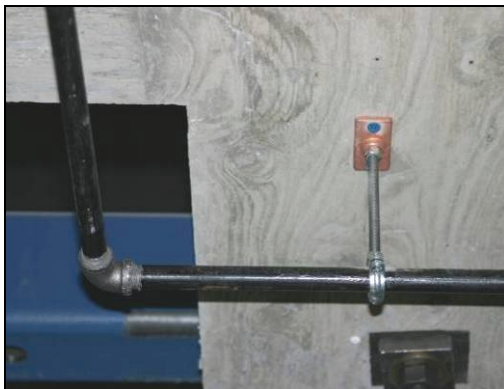
Figure 5.27. Vertical rod hanger detail
