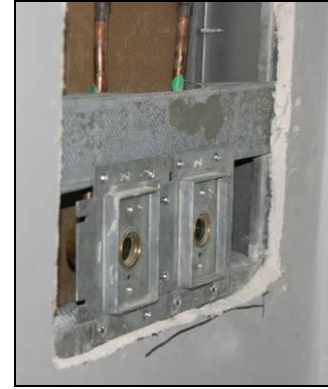
Figure 5.33. In-wall outlets mounting detail
