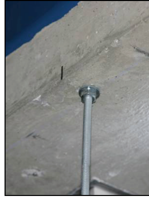
Figure 5.32. Connection hanger to top concrete slab
