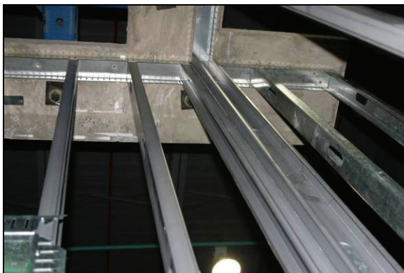
Figure 5.14. Top track connection detail
