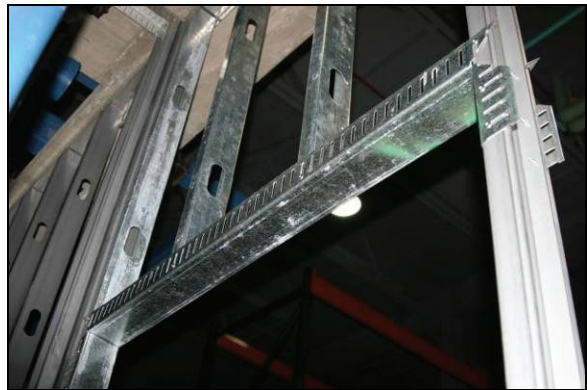
Figure 5.13. General view of door opening frame
