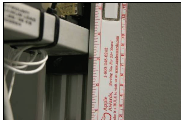
(b) Permanent vertical displacement of mounting arm of Monitor 4
