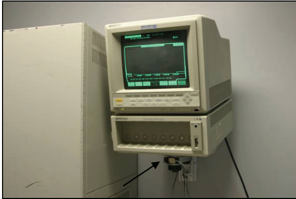
Figure 5.55. Detail of instrumentation at the base of wall mounted vital sign monitors. In the photo: accelerometers M1AVb, M1ANSb and M1AEWb
