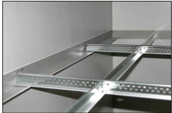
Figure 5.20. Ceiling grid and wall molding detail
