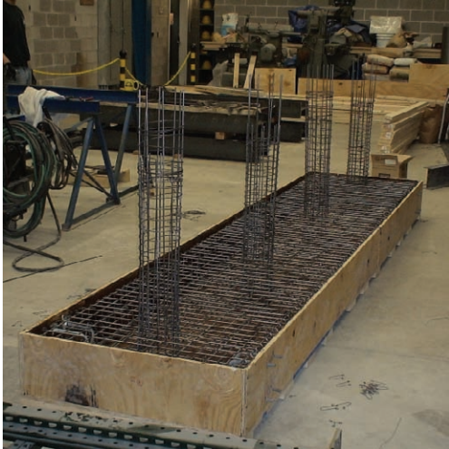
(a) Footing Reinforcement
