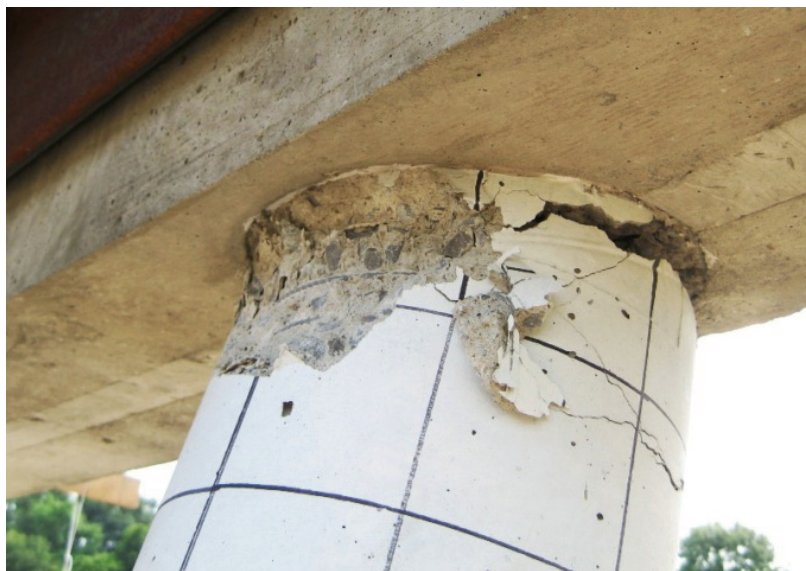
Figure 3-42 Back Diagonal View of Column RC1 at Top (Test 1)
