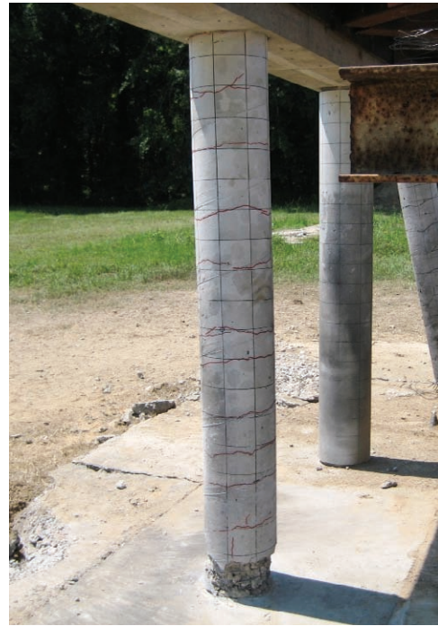
Figure 3-45 Back Diagonal View of Column RC2 (Test 2)
