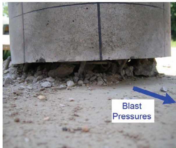
Figure 3-60 Back Diagonal View of Column SJ2 at Bottom (Test 3)
