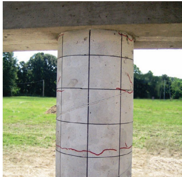
Figure 3-53 Back View of Column RC2 at Top (Test 2)
