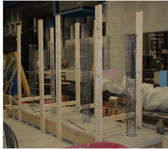
(b) Column Reinforcement after casting footing concrete
