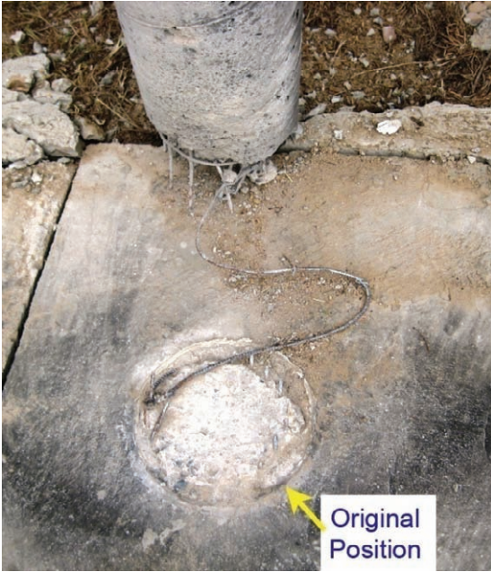
Figure 3-32 Column RC1 at Bottom (Test 1)
