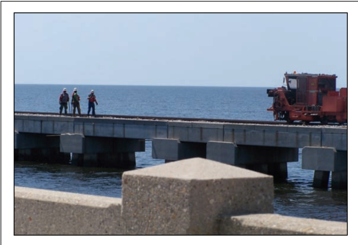
Figure 2-138. Norfolk-Southern had a crew relaying track about a week after the storm.
