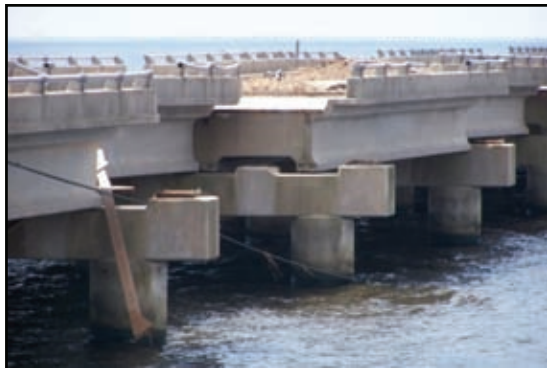
Figure 2-132. Span units are relatively intact.
