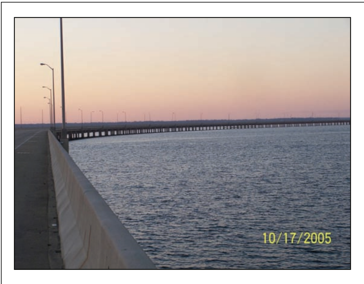
Figure 2-23. This bridge, connecting the Pascagoula Naval Station to the mainland performed well.
