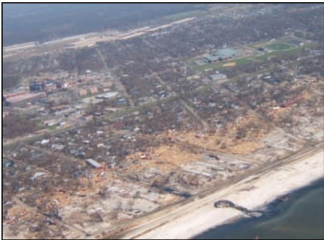
(w) Surge destroyed most things near the beach.
