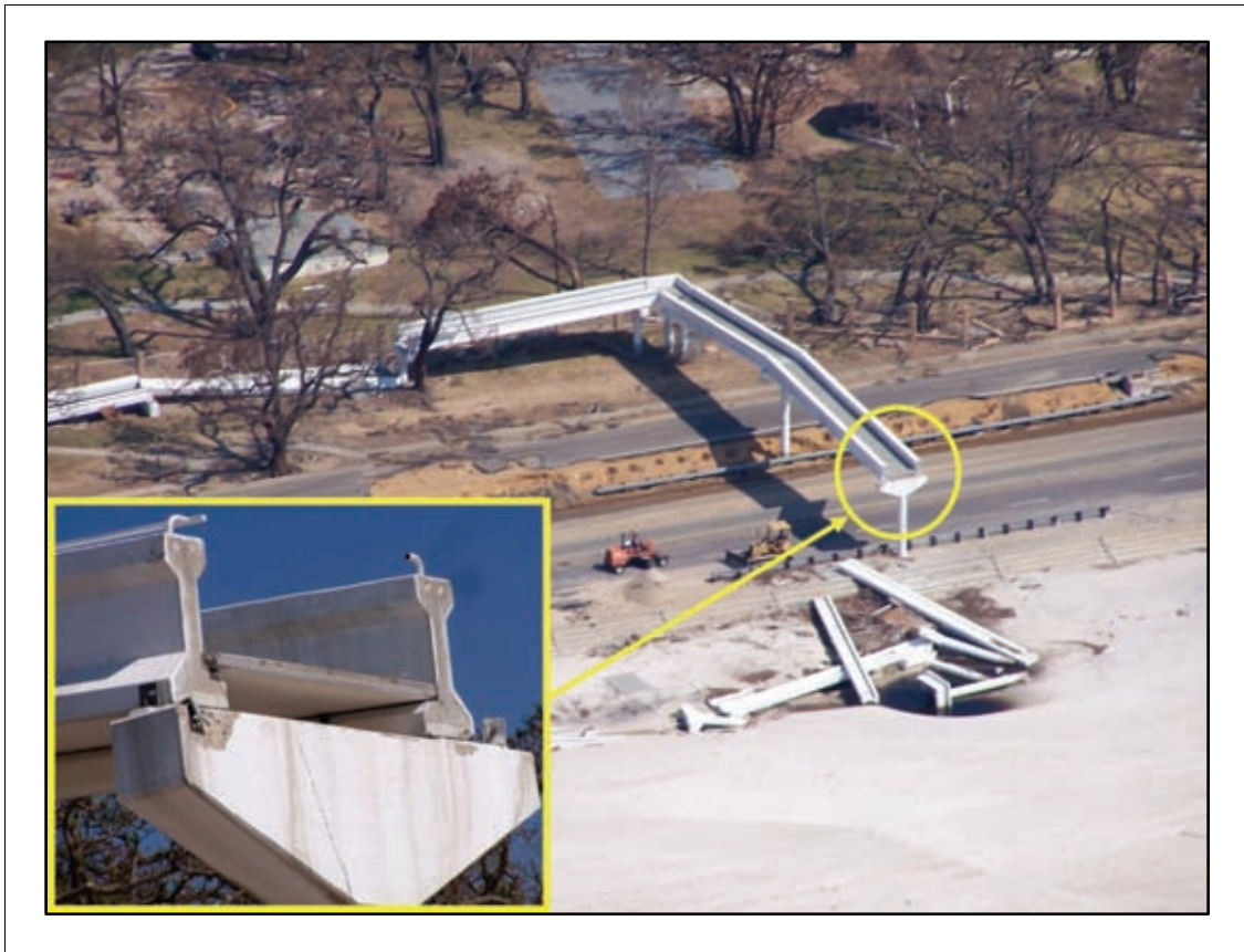
Figure 2-84. This pedestrian bridge utilized precast construction shown in the inset.
