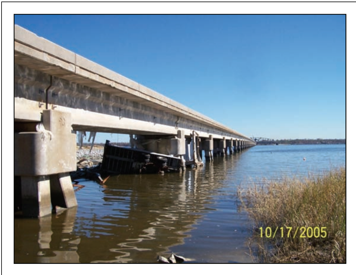
Figure 2-53. CSX railroad bridge, looking east from the west abutment.
