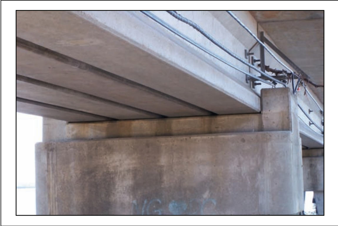
Figure 2-54. Pier and superstructure configuration of the CSX railroad bridge.
