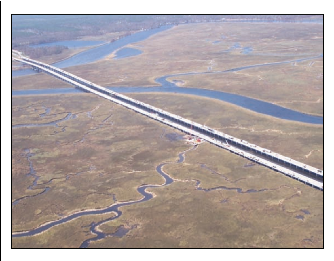
Figure 2-25. I-10 traverses a large salt bayou near Moss Point. It was hit and damaged by a stray barge.
