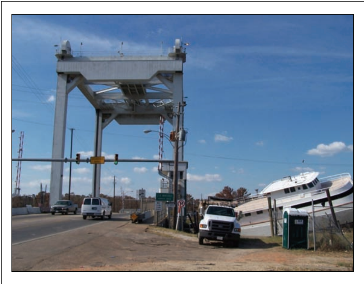
Figure 2-6. The boat on the right hit this lift bridge. The control room was also flooded.
