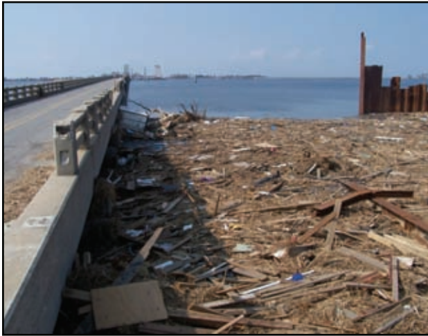
(g) Debris fields made walking hazardous.
