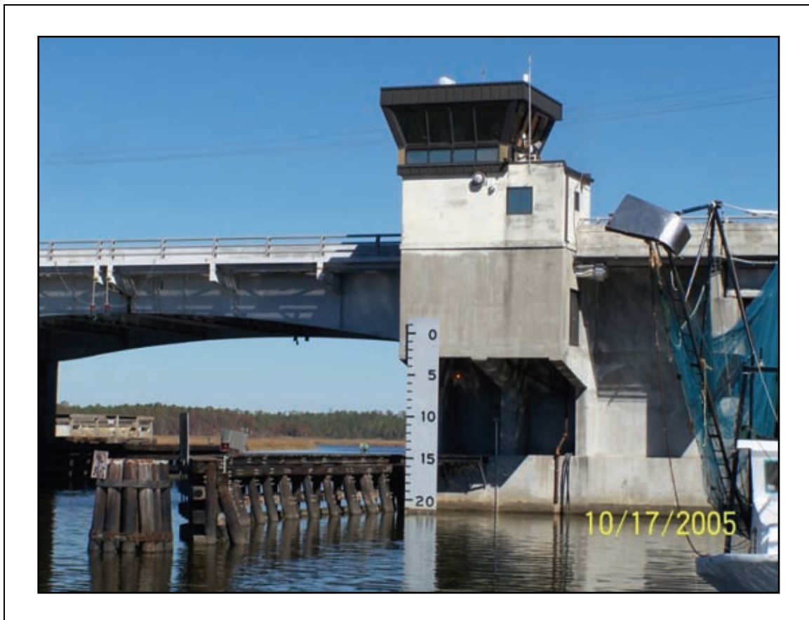
Figure 2-67. The mechanical room of this moveable bridge flooded, making the bridge inoperable.
