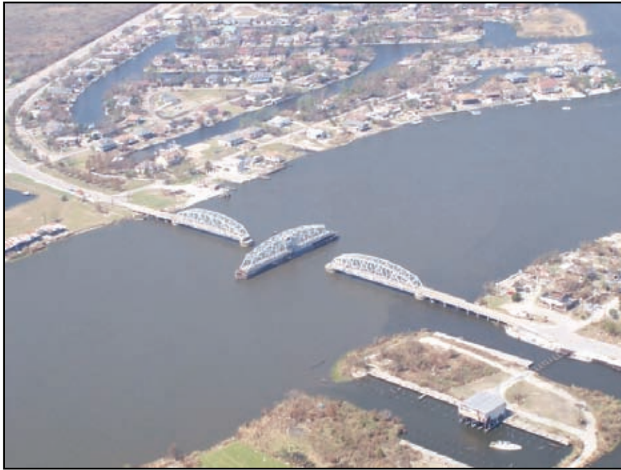
Figure 2-148. Facing NW. The swing span became inoperable.
