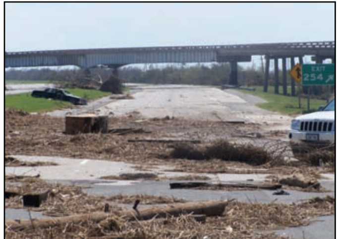
(l) Debris covered highways.
