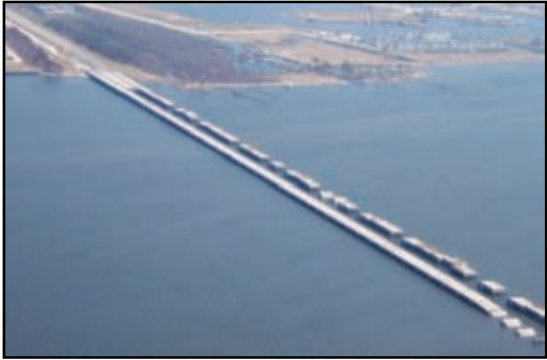
Figure 2-129. This view is looking SE so the EB bridge is on the far side. On this section of the bridge, the EB side lost many more spans.
