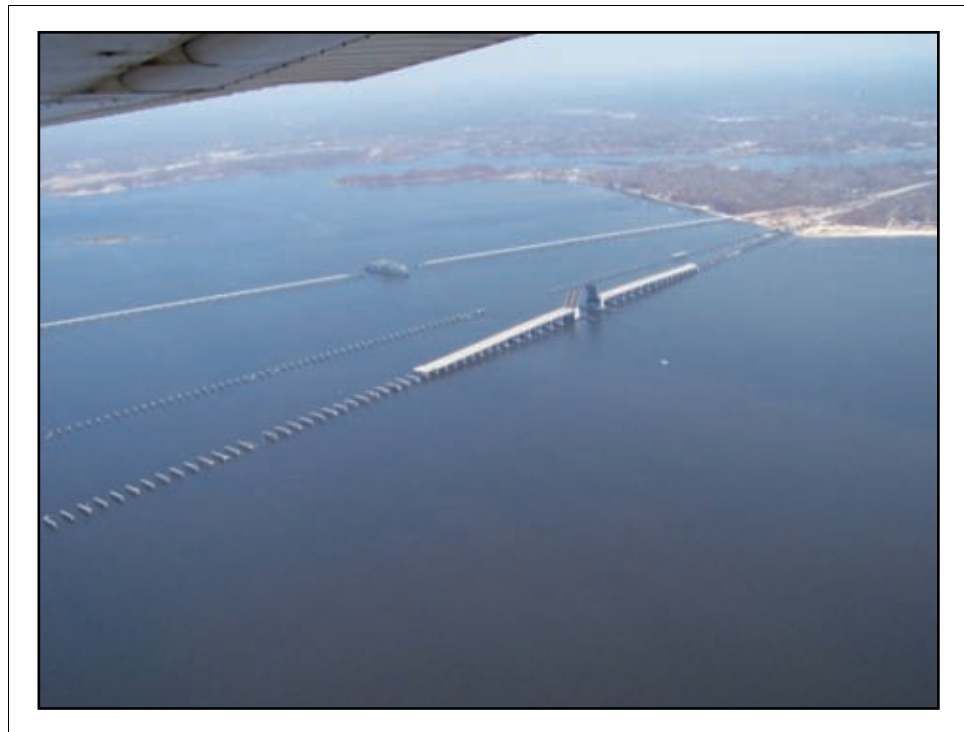
Figure 2-33. This Post-Katrina photograph (taken 9/11/05) shows the three bay crossings from Biloxi facing east toward Ocean Springs. Many spans are missing.
