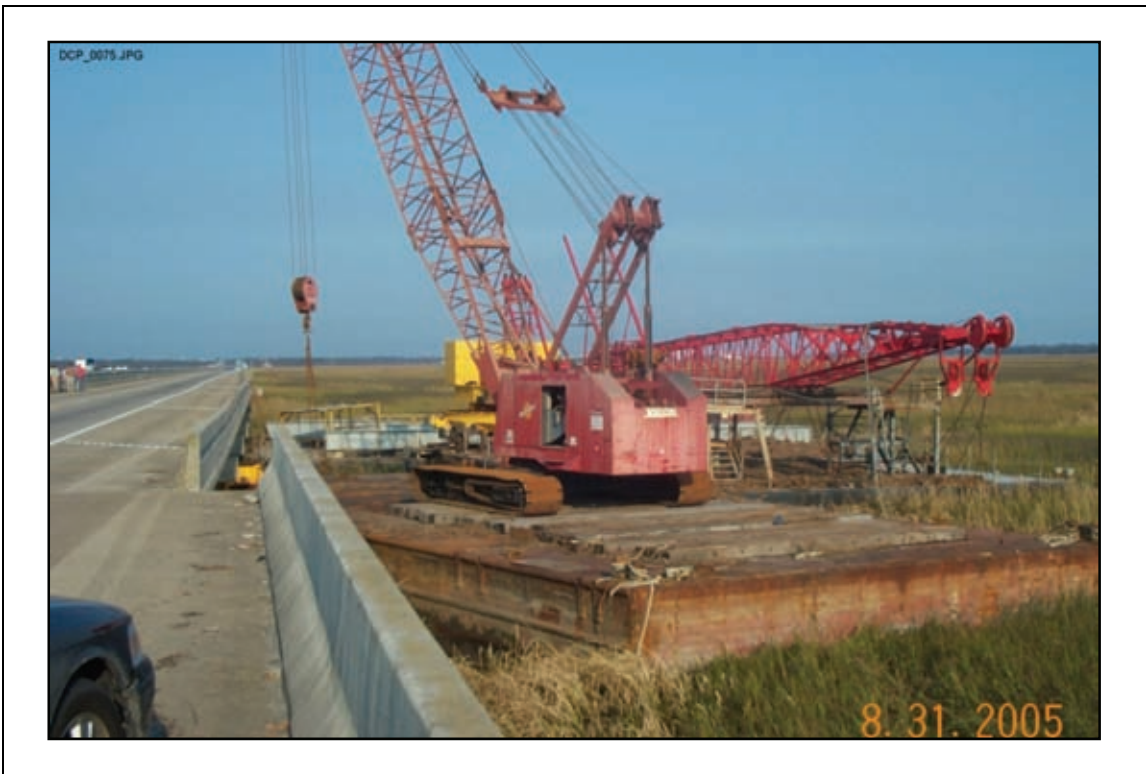
Figure 2-28. I-10 EB was hit by this barge and pushed four feet to the north.
