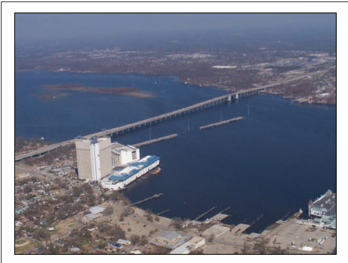
Figure 2-69. This photograph was taken facing NW. A hotel and floating casino are shown in the foreground. Near it is the bridge referred to as old route 110, with several sections missing. I-110 at the top of the picture was hit by a barge and debris but remained functional.
