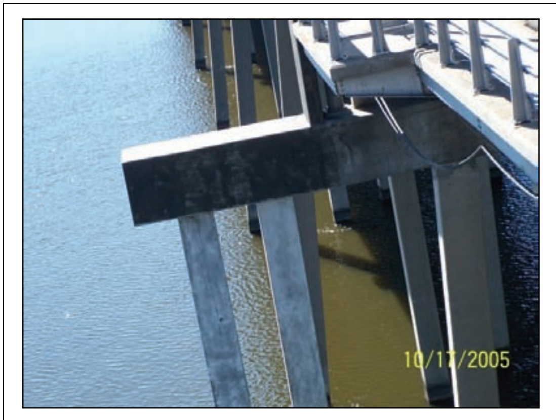
Figure 2-73. Repairs were made within a few weeks, allowing the bridge to be returned to full service.
