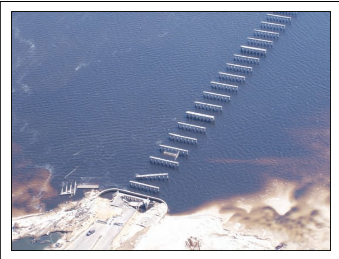
Figure 2-88. Western terminus of US-90 over St. Louis Bay, facing east.
