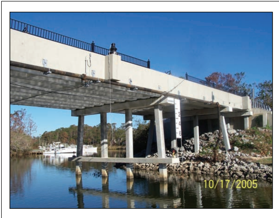
Figure 2-64. The Shearwater bridge is very close to Biloxi Bay and was submerged under water.
