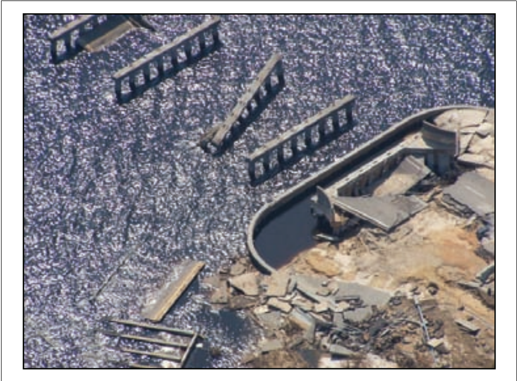
Figure 2-92. West abutment, looking SE, with an overturned span in the foreground.
