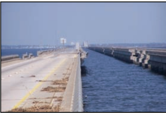
Figure 2-125. WB bridge is on the left.
