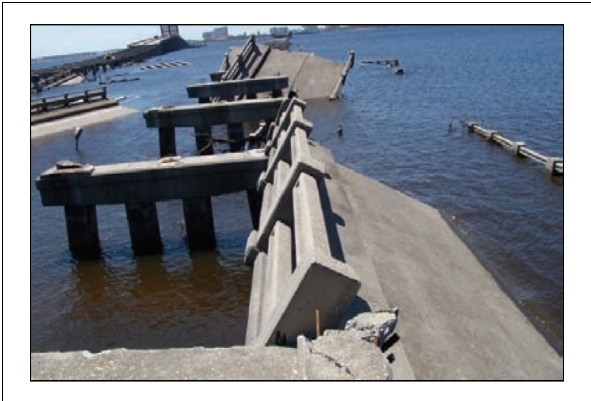
Figure 2-50. Looking west from the east abutment. US-90 is on the left.
