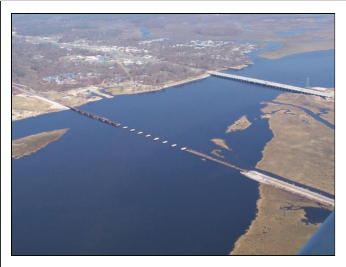
Figure 2-22. CSX railroad bridge lost the tracks and superstructure. US-90 is in the background.
