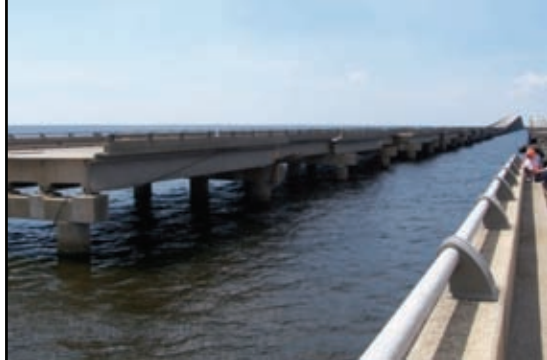
Figure 2-130. This view is looking SW from the deck of the WB bridge. Spans not dropped into the water completely were displaced to the south.
