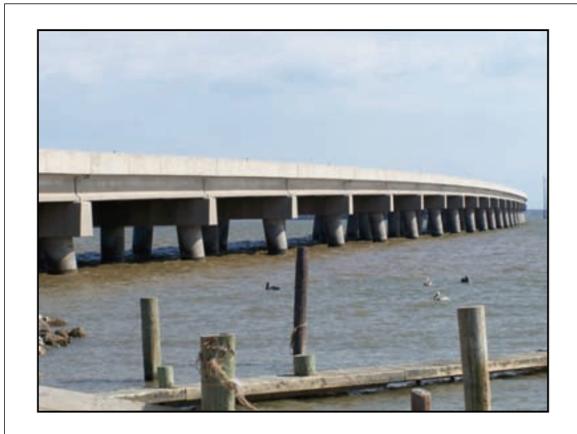
Figure 2-3. The Route 193 bridge to Dauphin Island, facing south.
