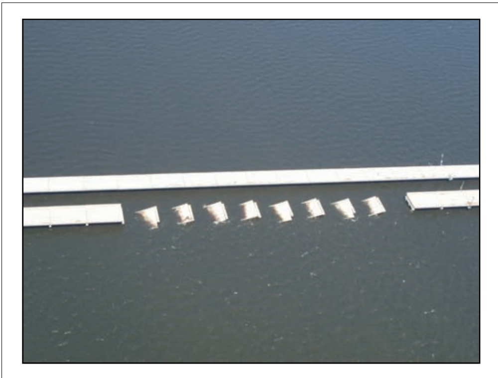
Figure 2-118. The missing span on the far right seems to have slid out, causing the others to topple.
