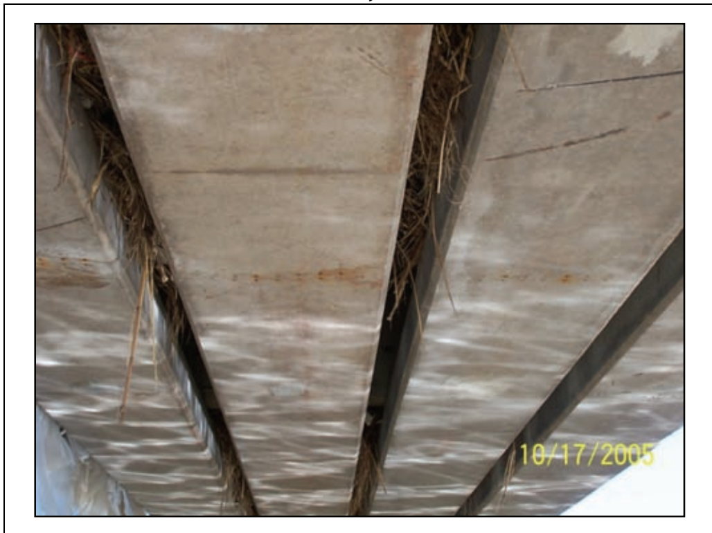
Figure 2-59. Tightly spaced prestressed beams with concrete diaphragms.
