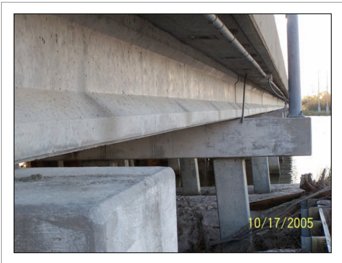
Figure 2-21. P/S concrete beams on concrete piers.
