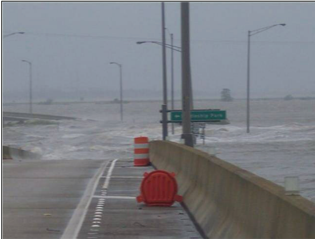
Figure 2-14. Several spans washed out the day of the storm. This photo faces east.
