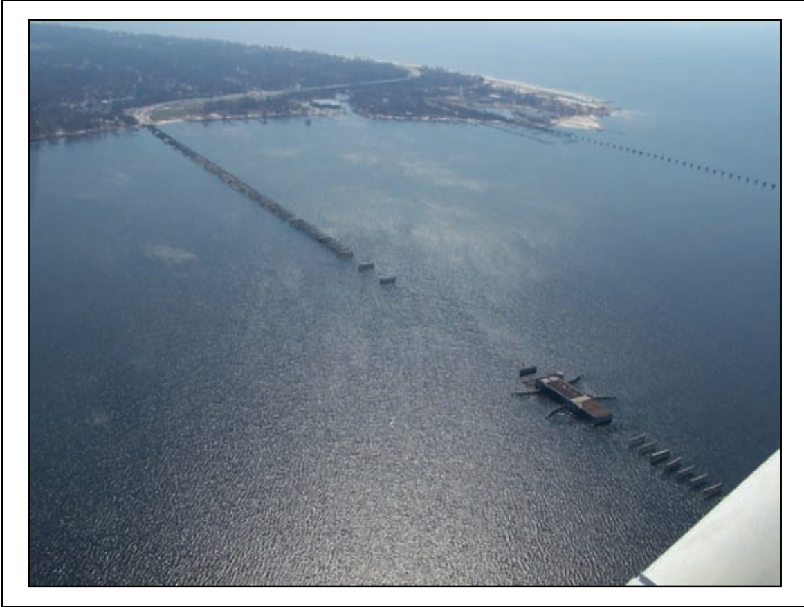
Figure 2-87. US-90 over St. Louis Bay, facing SE. The CSX railroad bridge is on the right.
