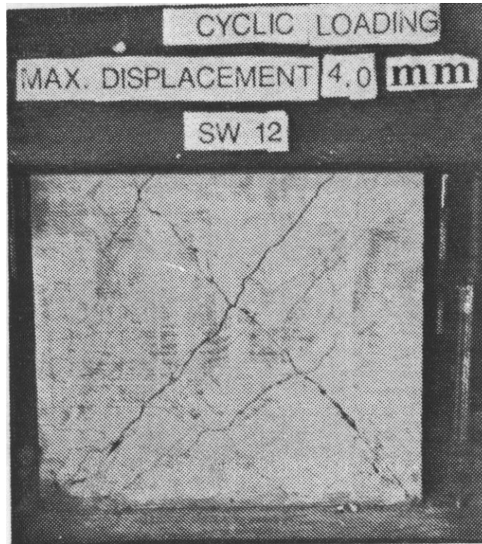
Figure C-108 Condition of wall SW12 at 0.81% drift [Lopes and Elnashai (1991)]
