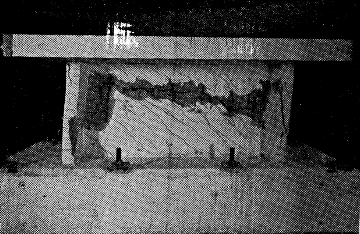
Figure C-268 Condition of wall B2-1 at the end of the test (drift > 8%) [Barda et al. (1977)]
