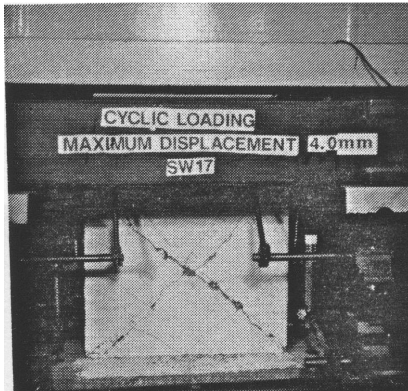
Figure C-147 Condition of wall SW17 at 0.81% drift [Lopes and Elnashai (1991)]
