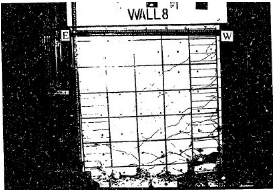
Figure C-179 Condition of wall 8 at -3.36% drift [Mohammadi-Doostdar (1994)]
