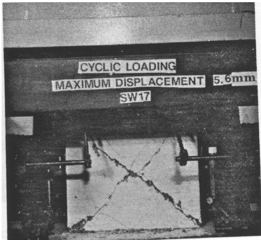
Figure C-149 Condition of wall SW17 at 1.13% drift [Lopes and Elnashai (1991)]
