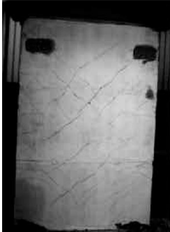
Figure C-187 Condition of wall MSW6 at the end of the test (maximum drift = 1.57%) [Salonikios et al. (1999)]
