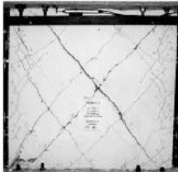
Figure 1-2 Diagonal tension failure of wall 27 tested by Hidalgo et al. (2001)
