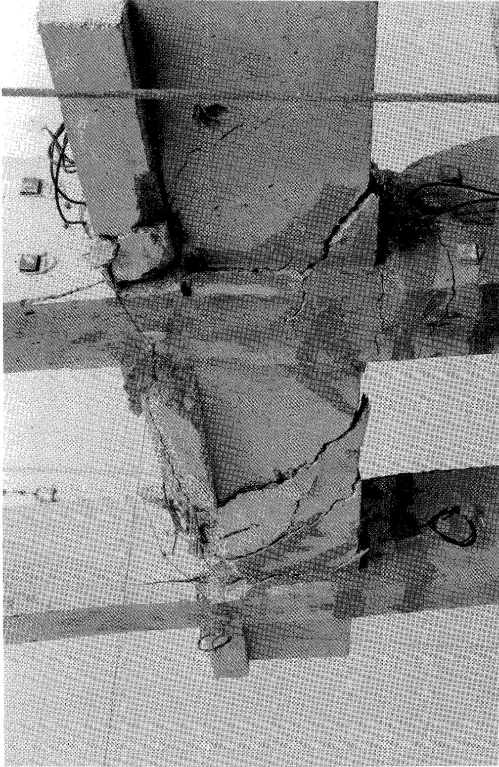
Fig. 4.33 TRANSVERSE GIRDER WHICH "FAILED" DUE TO FRACTURE OF REINFORCEMENT.
