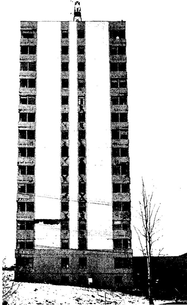
FIG. 4.5 MCKINLEY BUILDING: EARTHQUAKE DAMAGE IN NORTH END WALL
