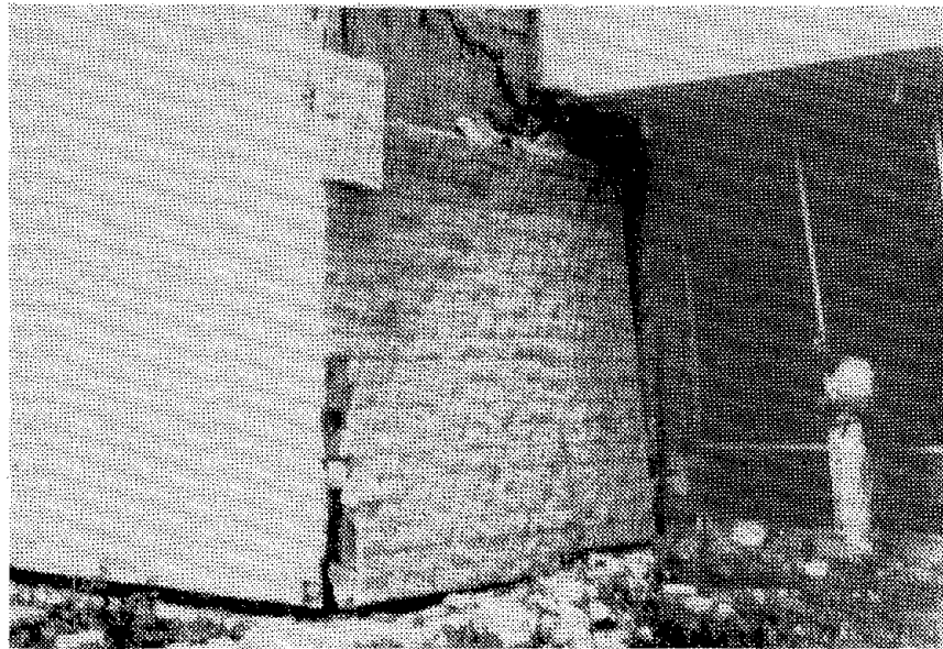
FIG. 3.16 DAMAGE IN FIRST STORY ELEVATOR SHAFT WALL NEAR P-19
