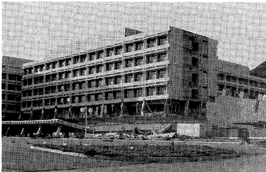
(b) GENERAL VIEW OF DAMAGE TO MAIN BUILDING (WING D IN FOREGROUND)
