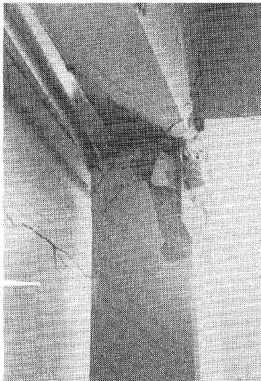
(b) DETAIL OF DAMAGE TO COLUMN FF-26.6 AND ADJACENT RETAINING WALL
