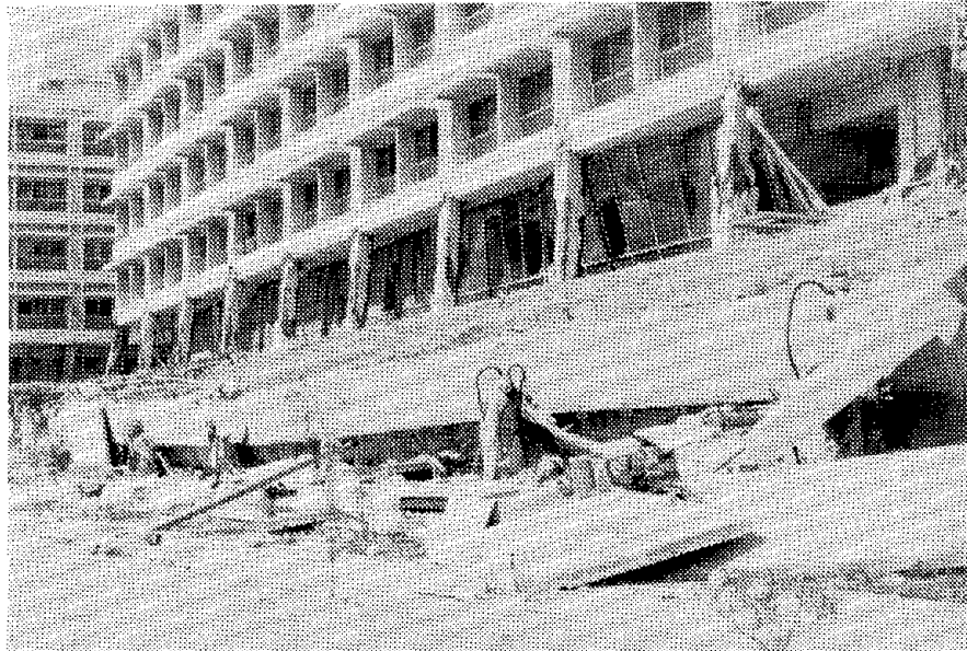
FIG. 3.19 DETAILS OF DAMAGE TO PRECAST PANELS
