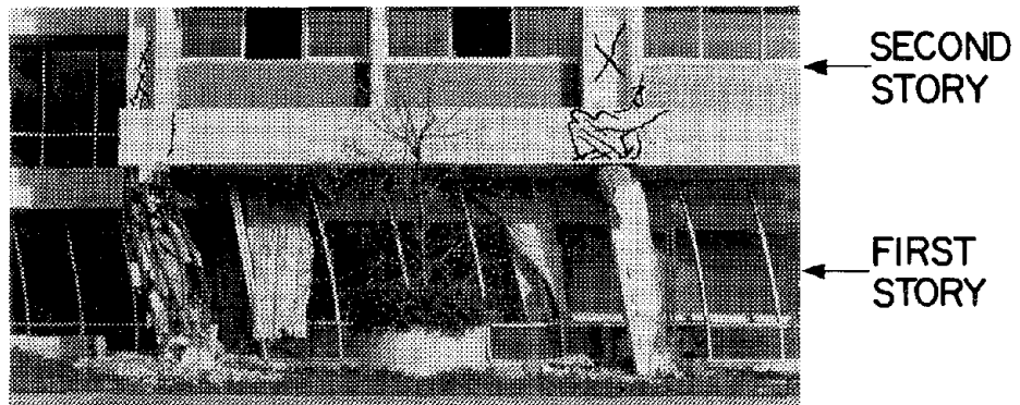
FIG. 3.12 COMPARISON OF DAMAGE TO FIRST STORY TIED AND SPIRAL COLUMNS (UNIT A). NOTE DISTRESS IN BEAM-COLUMN JOINT AND IN SECOND STORY TIED COLUMN
