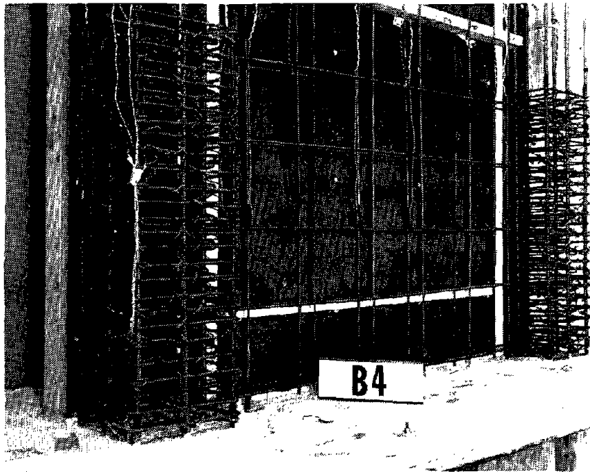
Fig. A-13 Reinforcing for Specimen B4
